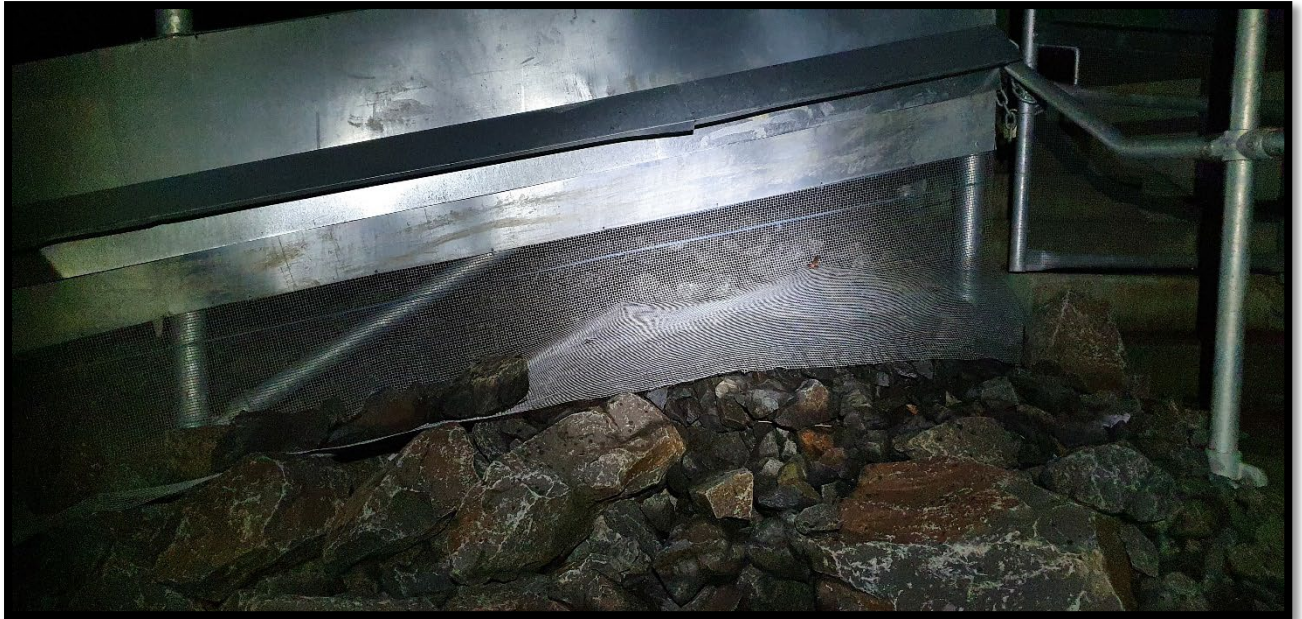
Plate 4-3. Example of return flap wash out or holes beneath the mesh within 50 m of installed ponds at ch.118500 Site 10 A (Tabbimoble).
