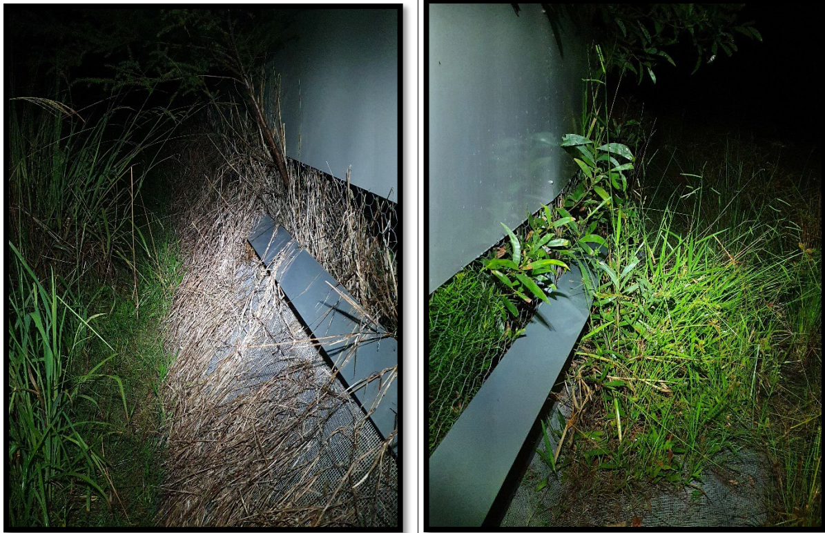
Plate 3-1. Evidence of herbicide treatment to contain or reduce the permeability of frog exclusion fence around ch. 140000 (left) and vegetation creating opportunities for frogs to move onto the roadway around ch.139000 (right).
