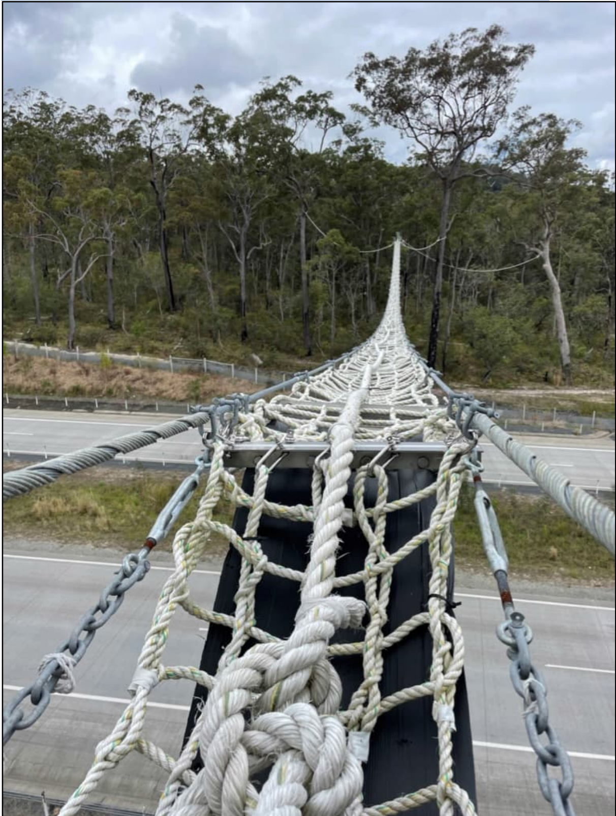
Plate 1: Rope bridges were suspended >10m above the road surface and supported by poles adjacent to the forest edge. A camera was fitted to the bulkhead at each end of the bridge.
