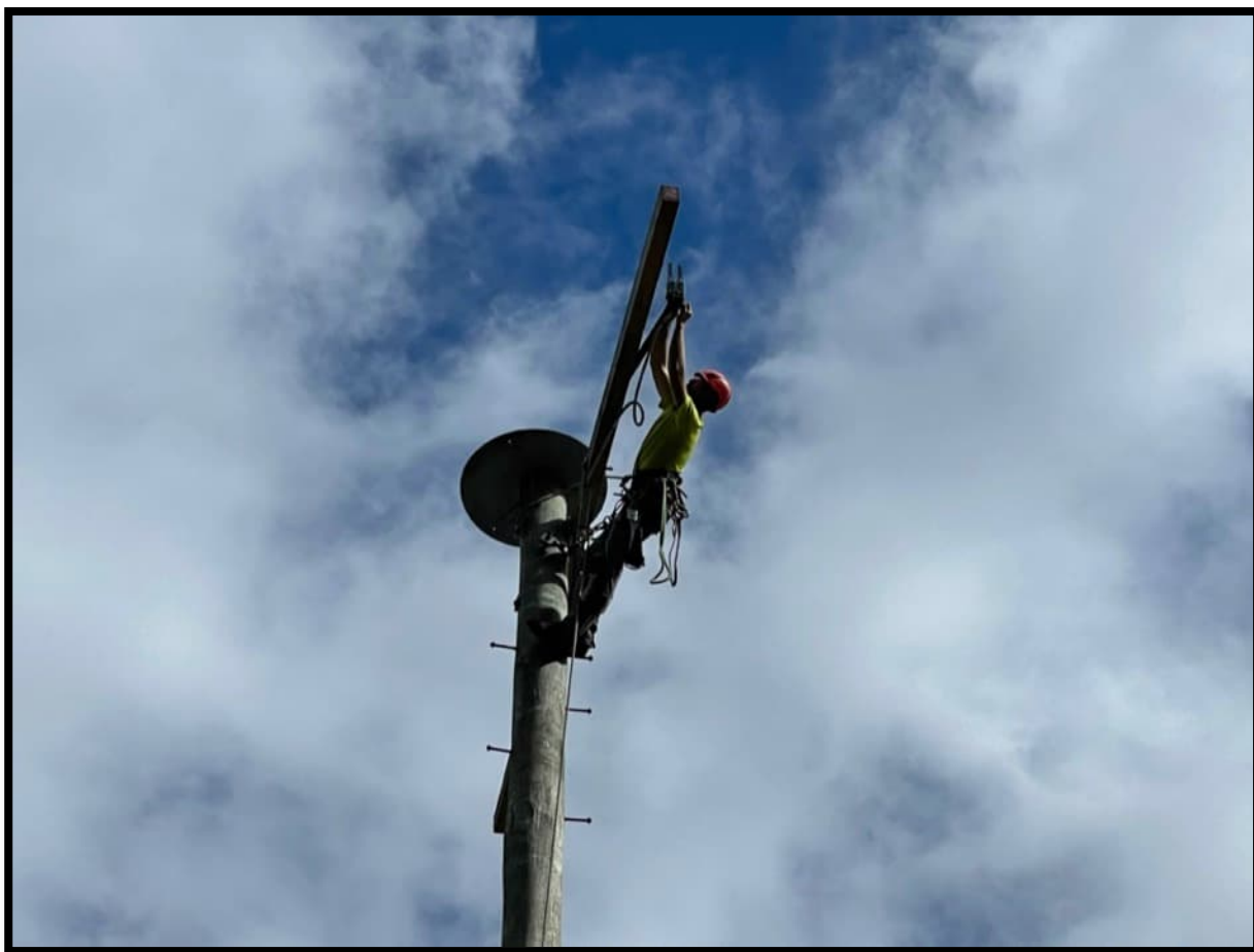
Plate 2: Location of camera attachment on glide poles in S3-11. Each structure contained a wireless 4G Enduro camera fitted to a steel arm and connected to a solar panel.
