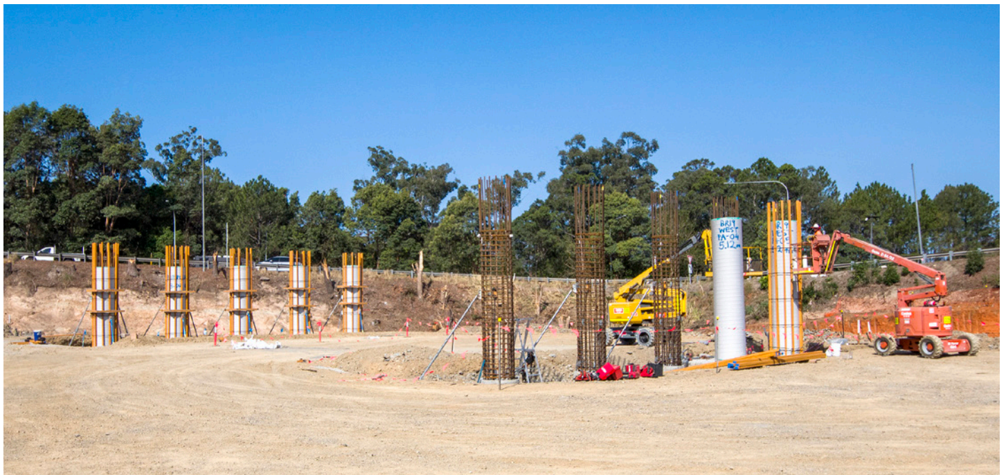
Steel reinforcement and temporary tubes in place for column construction at Korora Hill Interchange
