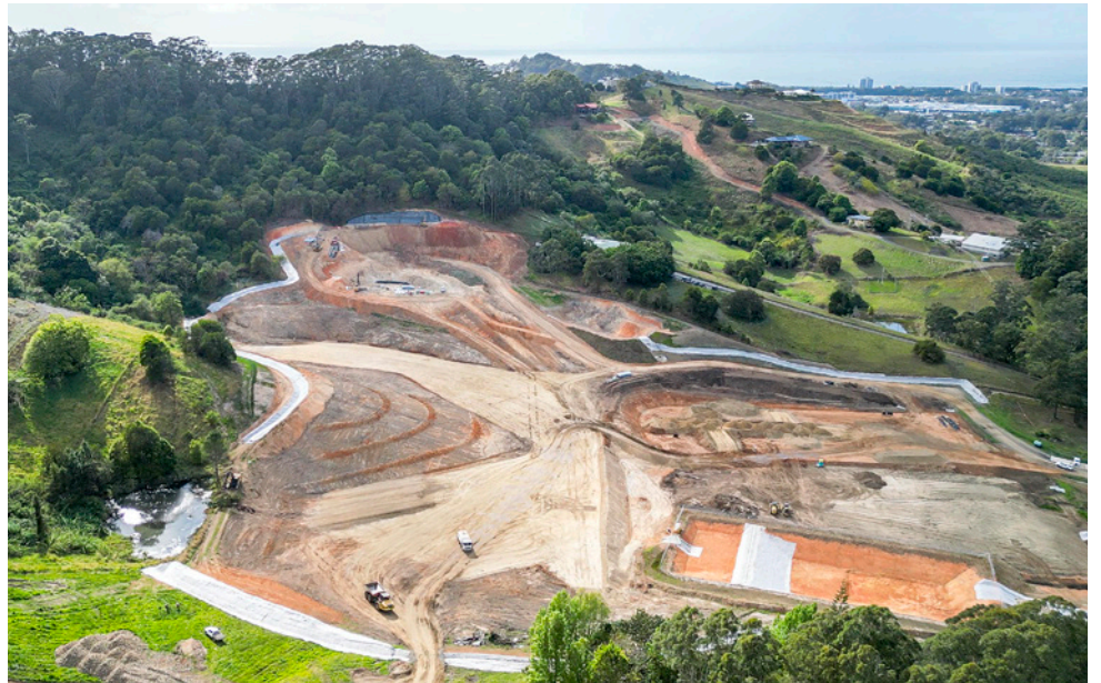
Temporary drainage and sediment basin near Gatelys Road Tunnel
