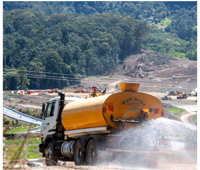
Water cart in use for dust suppression
