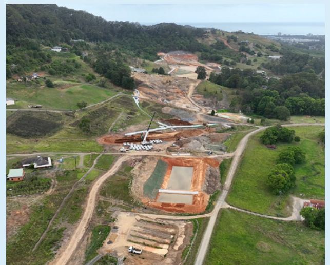
HES basin near Mackays Road
