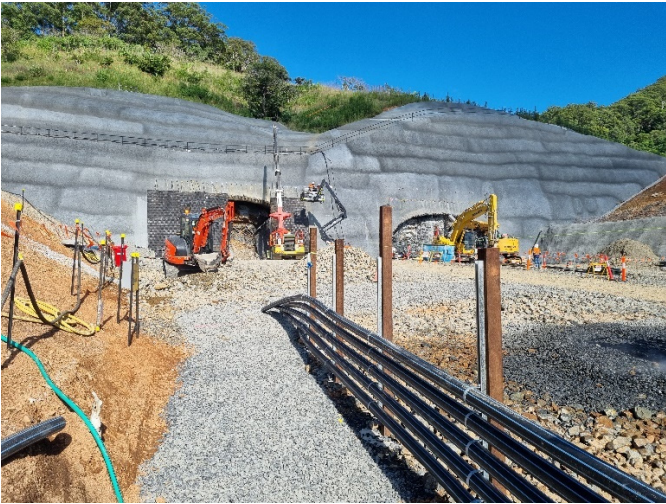
Image 5: Gatelys Rd tunnel north portal (Ch19300) – Initial tunnelling works, including rock hammering and drill & blast
