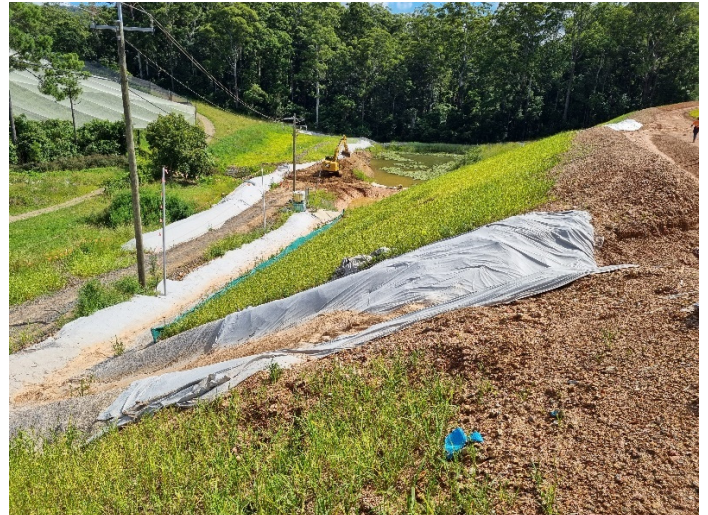
Image 8: Korora Hill, Fill 18 (Ch21700) – Fill batter that has been hydromulched and sediment basin repairs after rain
