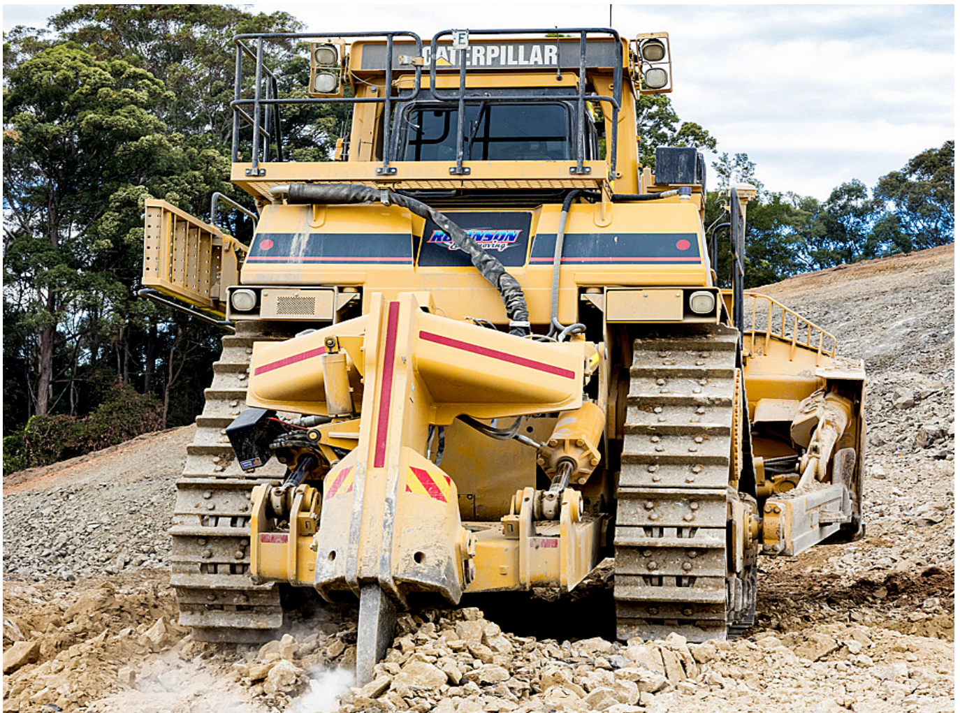
Bulldozer breaking through rock on the Coffs Harbour bypass
