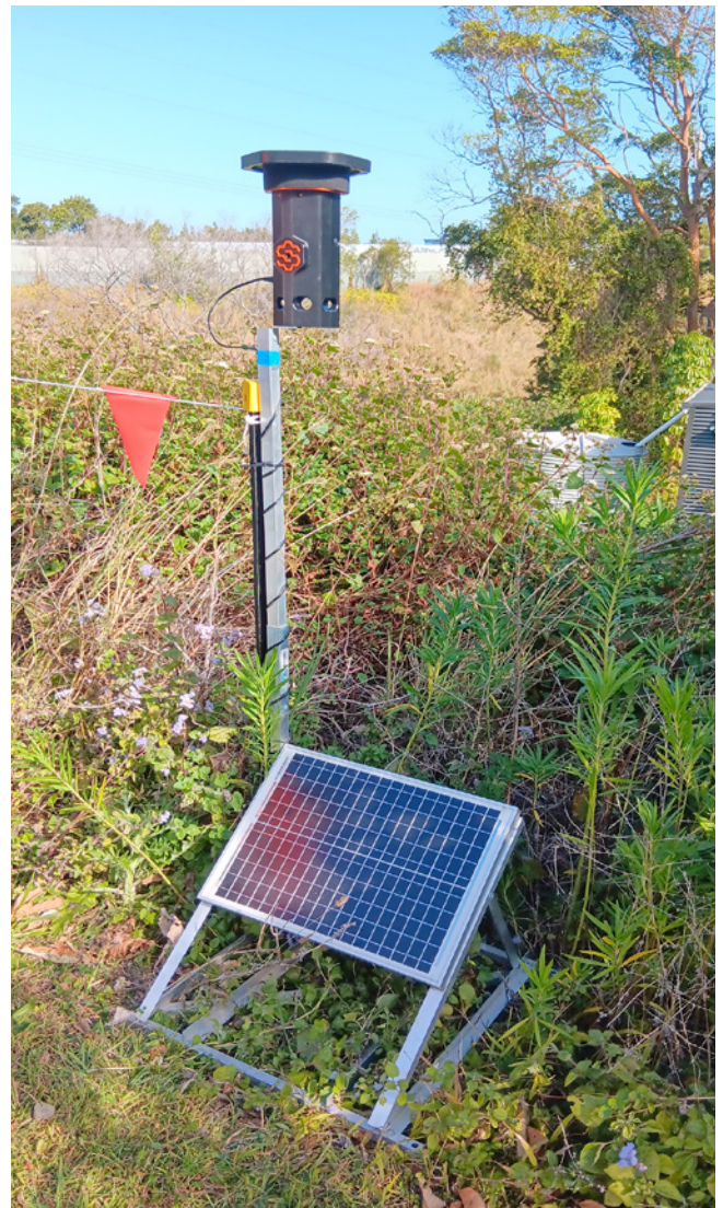
Noise monitor in place on the Coffs Harbour bypass
