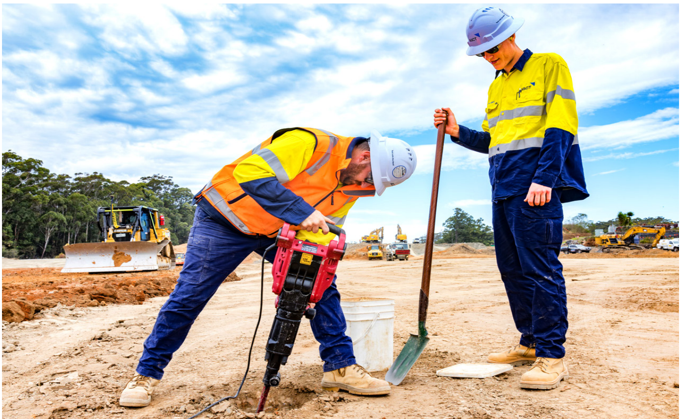
Jackhammer in use on the Coffs Harbour bypass
