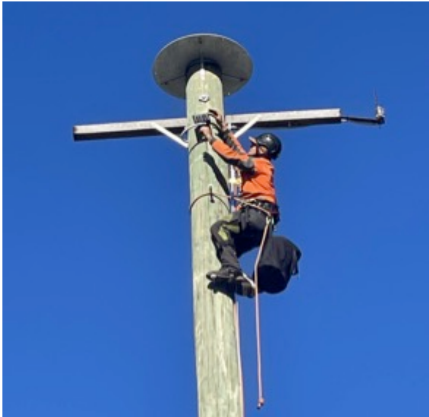
Plate 2: Location of camera attachment on glide poles in S3-11. Each structure contained a wireless 4G Enduro camera with a solar panel.
