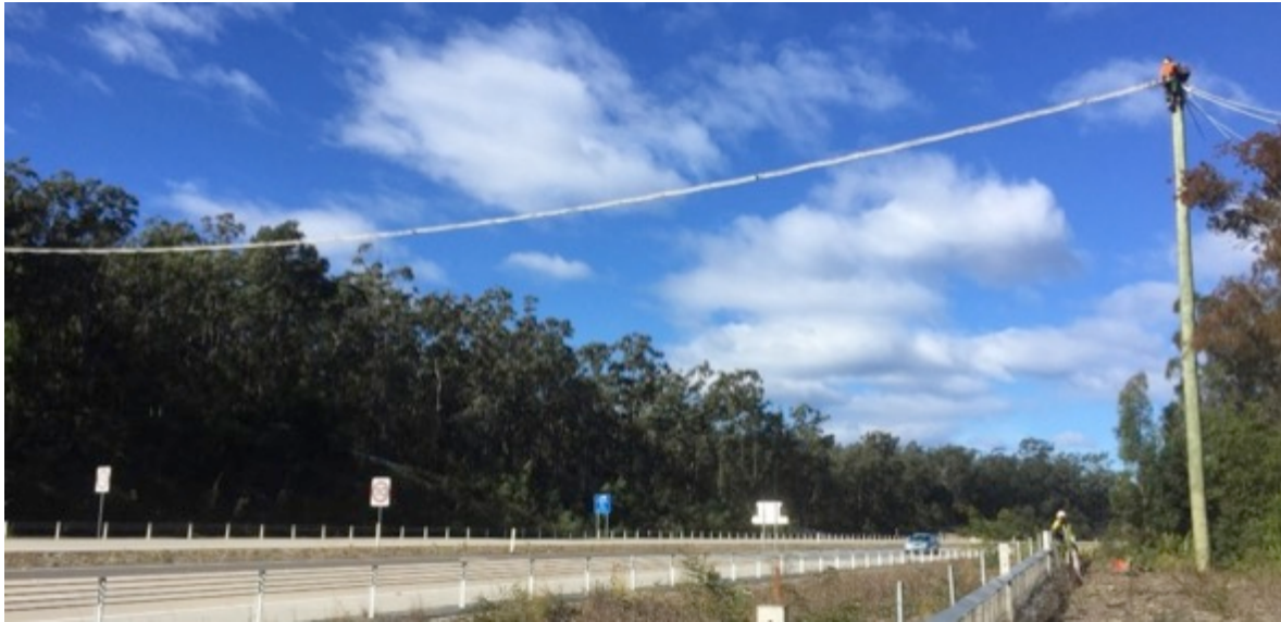
Plate 1: Rope bridges were suspended >10m above the road surface and supported by poles adjacent to the forest edge. A camera was fitted to the bulkhead at each end of the bridge. Black core-flute was cable tied to the underside of the rope ladder at each end during year 1 to reduce the incidence of false-triggering caused by traffic.
