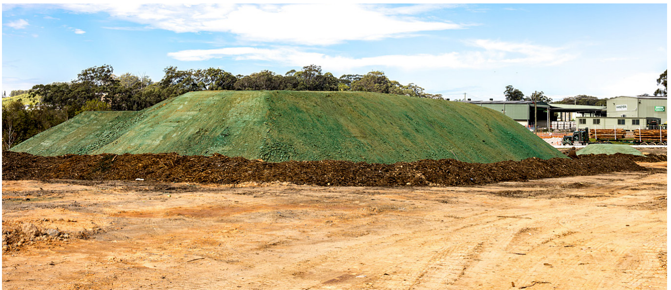
For stockpiles, we use soil binders to minimise dust
