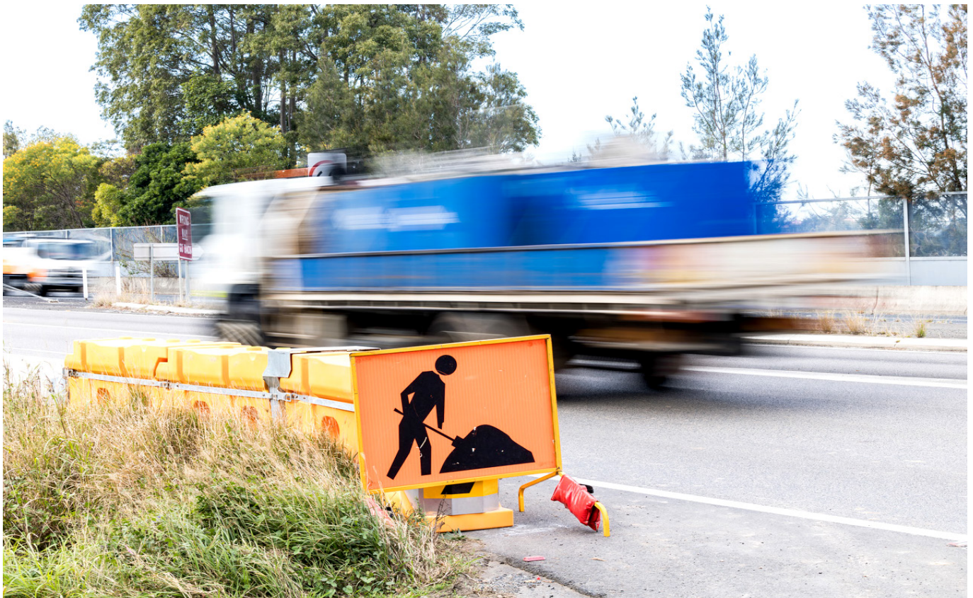
Road work signage in place on the Coffs Harbour bypass
