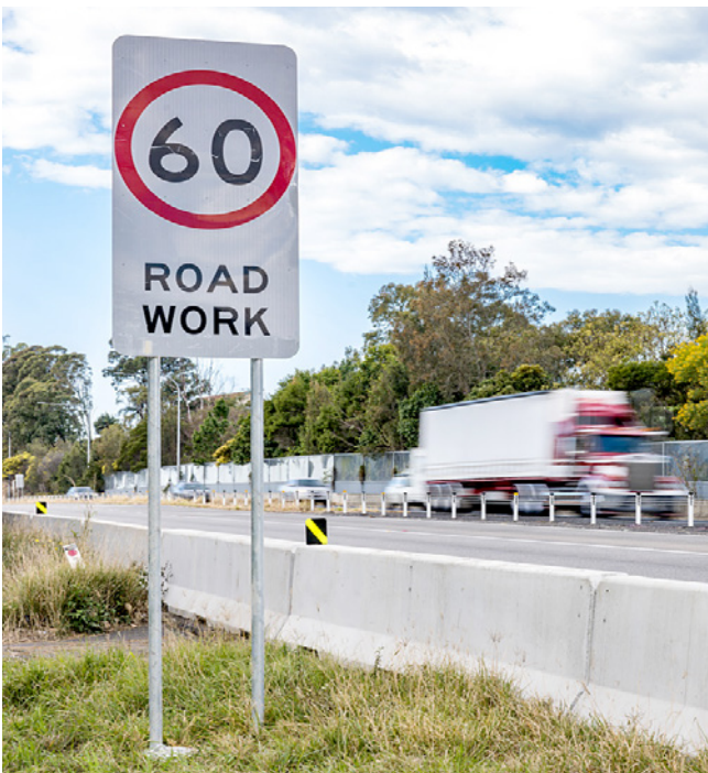
Road work speed limit in place at Korora
