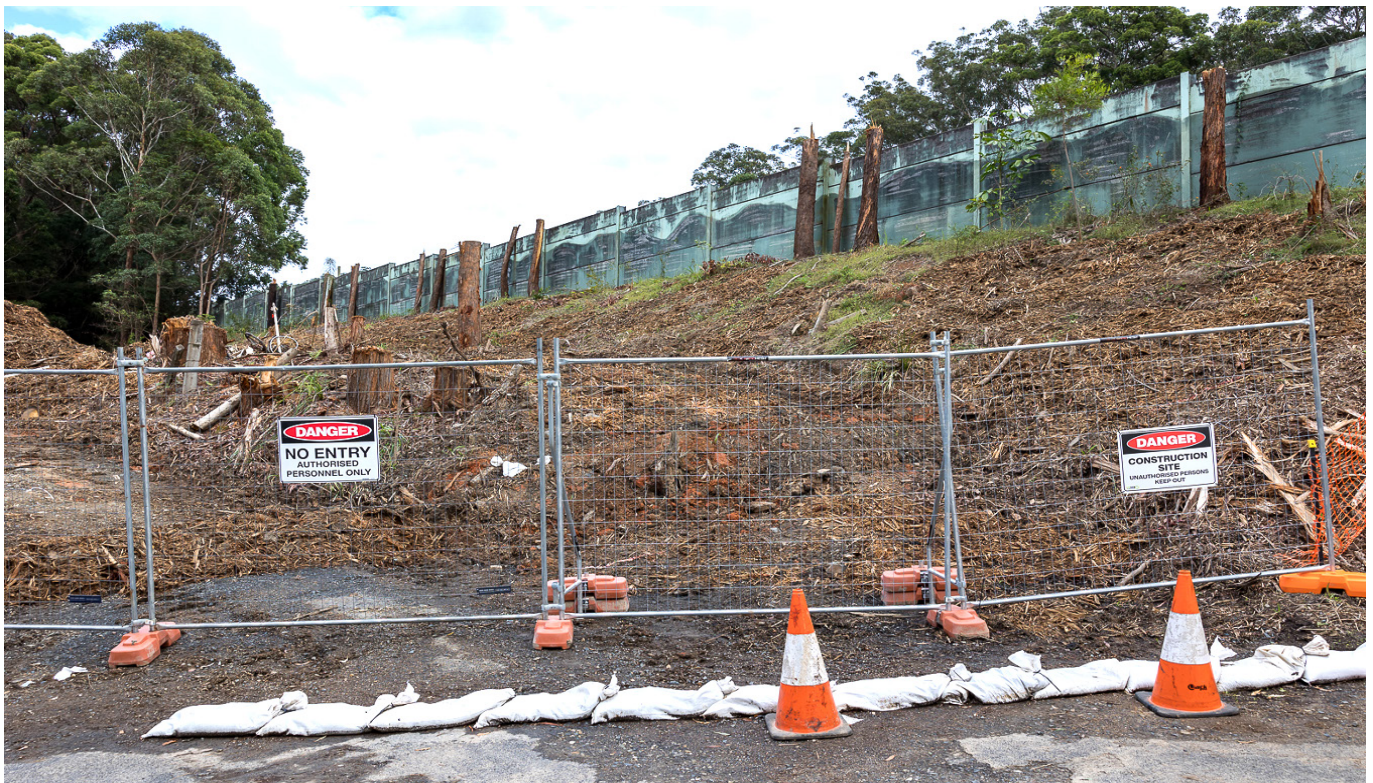
Temporary fencing and delineation signage on Korora School Road
