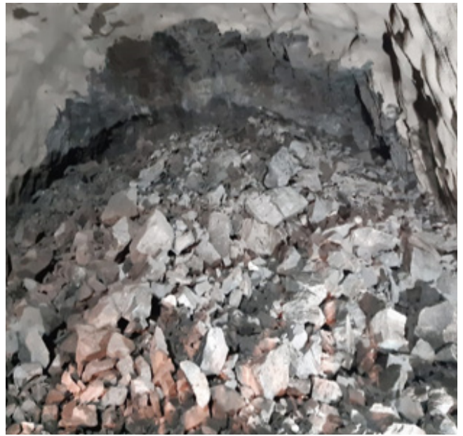
Excavating, hammering and removing rock from the floor and walls
