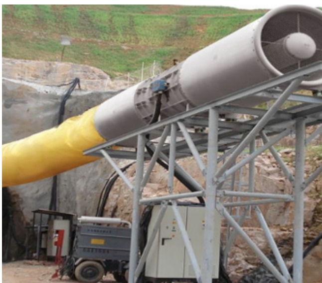
Ventilating the tunnel
