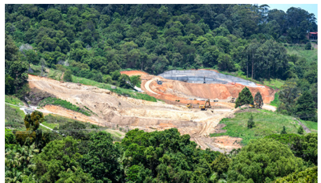
Tunnel portal preparation work at Gatelys Road Tunnel southern portal
