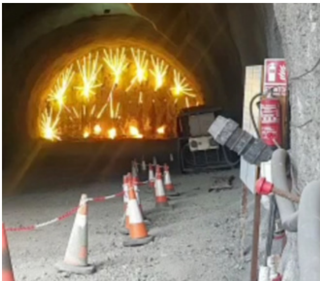
Detonating the blast
