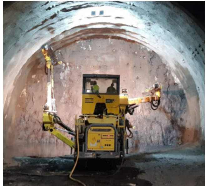
Drilling holes into the rock
