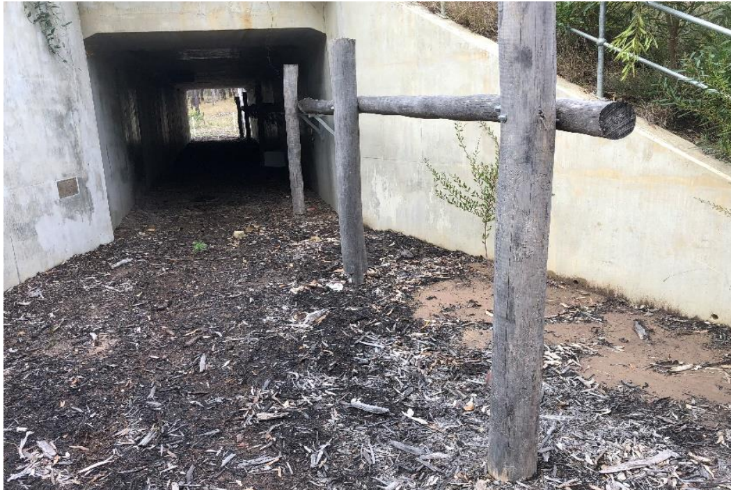
Plate 1: Box culverts monitored in sections 1-2 contained fauna furniture and some featured mulch spread over the concrete floor.
