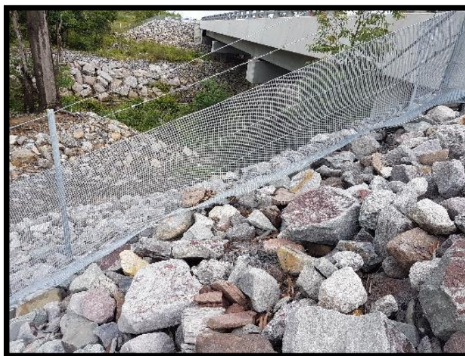
Plate 3-2. Missing frog exclusion fence at Corindi Creek on the northern abutment (left) and frog fence return facing the opposite way along with numerous holes at the bottom of the fence (right).
