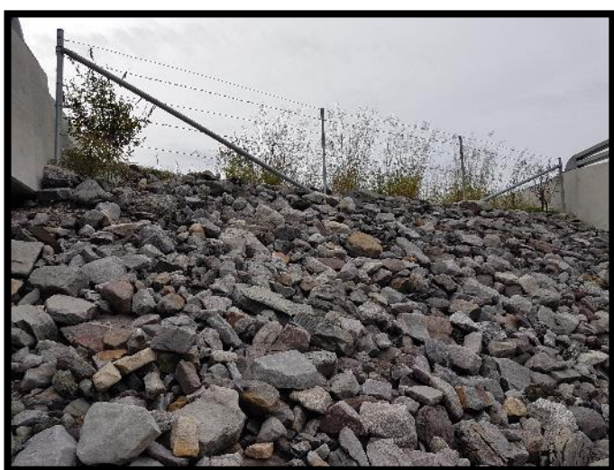
Plate 3-2. Missing frog exclusion fence at Corindi Creek on the northern abutment (left) and frog fence return facing the opposite way along with numerous holes at the bottom of the fence (right).
