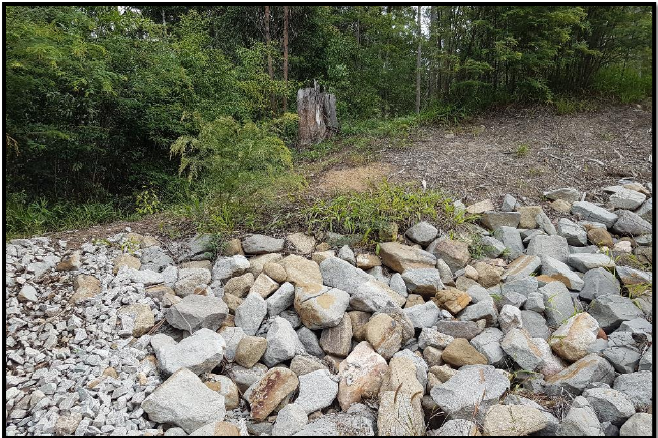
Plate 3-9. Riparian zone on upstream side at Boney's Creek with large aggregate to control erosion but no use of plantings on mulched creek bank.
