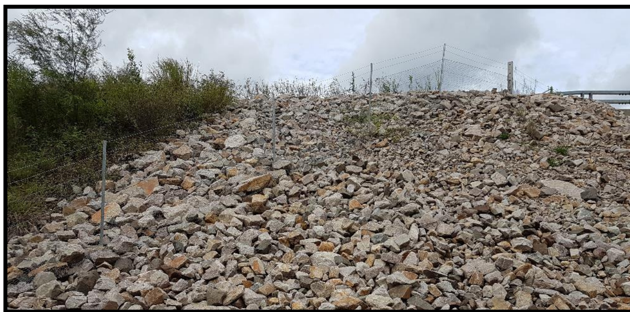
Plate 3-4. North bound fence on the Halfway Creek bridge abutment showing large aperture wire not suitable as frog fence.
