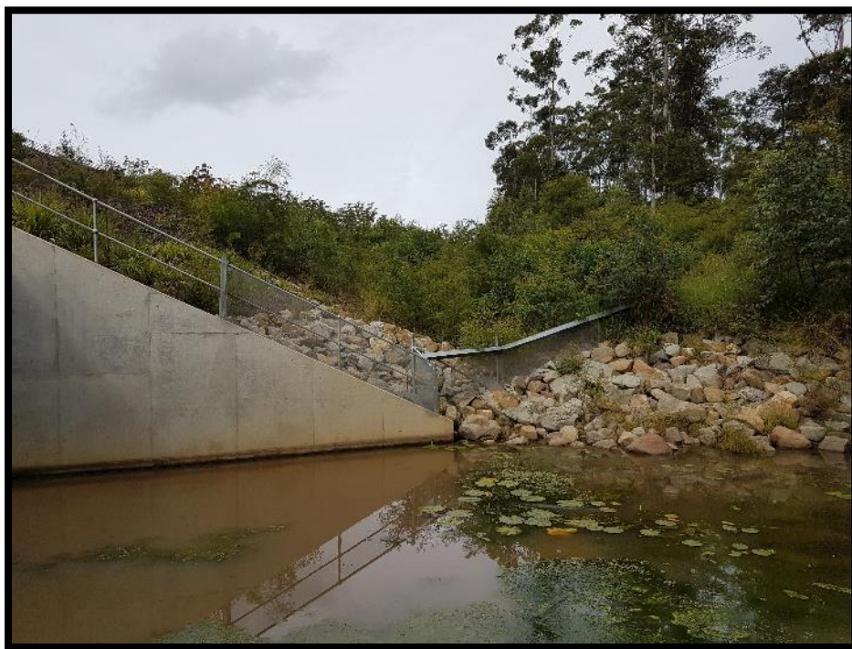
Plate 3-10. Frog exclusion fence at upstream side of Boneys Creek traversing large aggregate with gaps in the fence.
