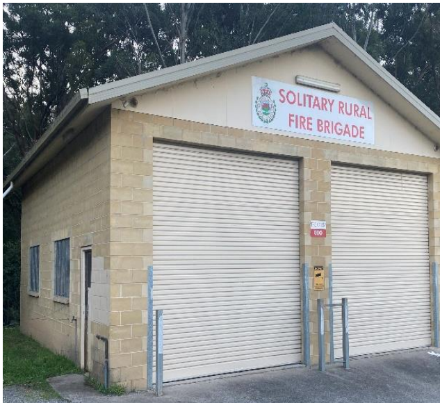
The existing RFS shed is being demolished and rebuilt.
