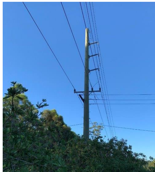
We have commenced replacing poles in the south of the alignment.
