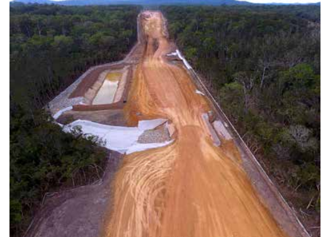
Foundation work on Coldstream area (November 2016)
