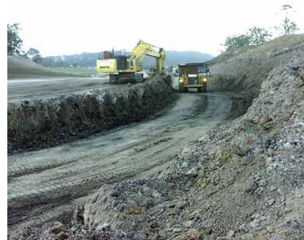
Loading and haulage work at Causleys Lane
