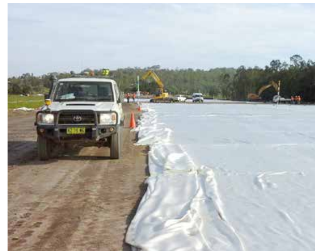
High strength fabric installation at Maclean
