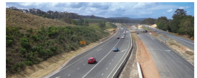
Headland Road overpass Sapphire looking north
