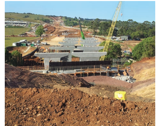
Tintenbar to Ewingsdale upgrade - bridge work looking south over Byron Creek
