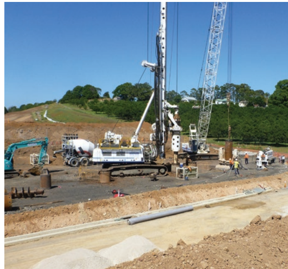
Tintenbar to Ewingsdale upgrade - bridge piling work at Watsons Lane
