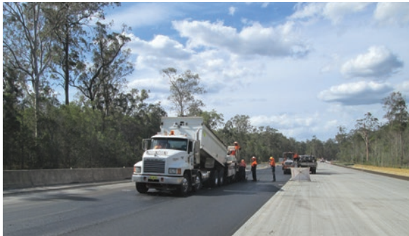
Asphalt paving work at the southern end of the project
