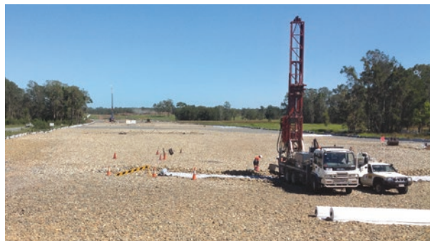
Geotechnical testing in soft soil north of Frederickton interchange
