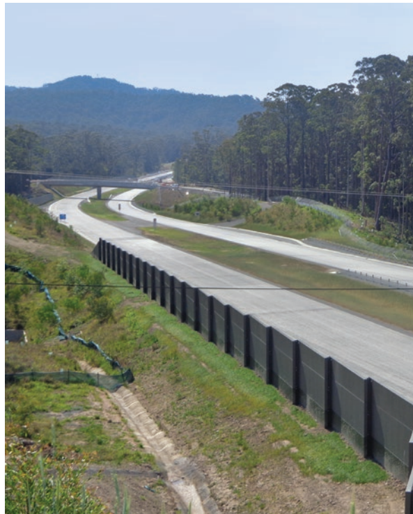
Sapphire to Woolgoolga upgrade - looking north to Woolgoolga Creek Road on the bypass
