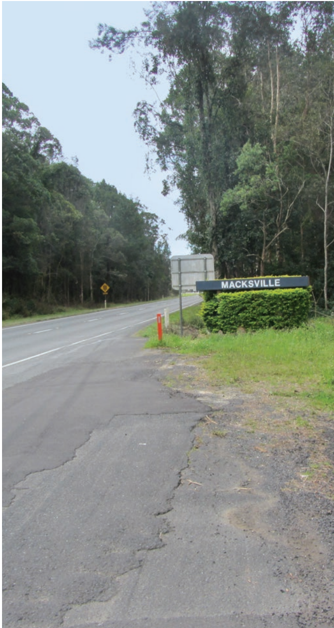
Existing Pacific Highway at Macksville
