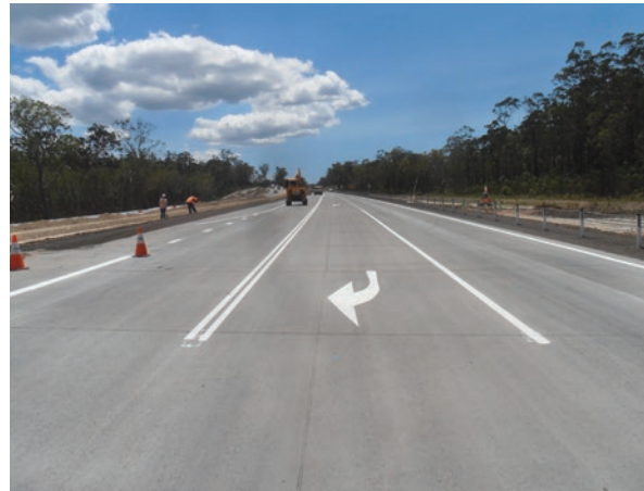
Devils Pulpit - line marking in preparation for upcoming traffic switch
