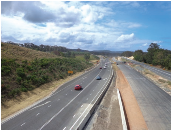
Sapphire to Woolgoolga upgrade - Headland Road overpass Sapphire looking north
