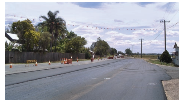
Old Post Office Lane - asphalt paving work under way
