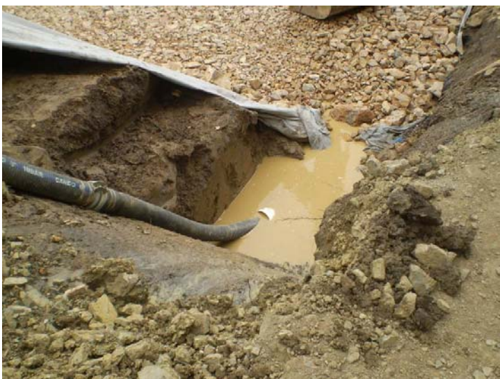
Figure 4. A sump adjacent to a working area may require higher levels of maintenance in order to remain effective. Dewatering to a larger sediment basin will be a more viable treatment measure when compared to flocculating the sump itself. Consideration to minimising exposed fines around the immediate catchment (e.g. bottom left corner of the figure) will also reduce sediment entering the sump if deemed practical for construction purposes.
