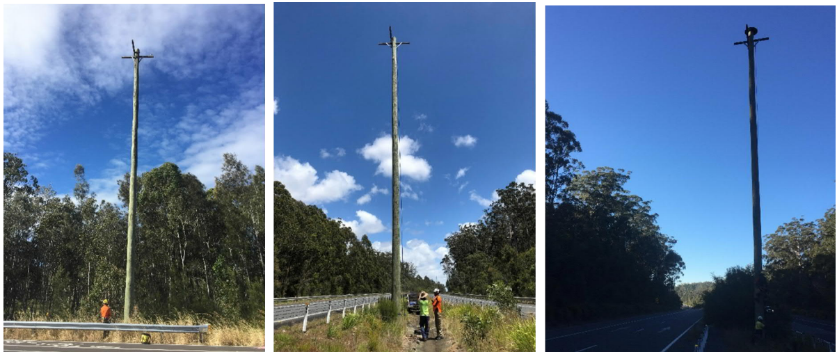
Plate 2: Glide poles stood 17.4m to 20m above road level and featured perpendicular and parallel-to-road cross arms. GP1 (left) was positioned adjacent roadside forest habitat on the eastern edge of the Solitary Island Way, approximately 50m from the rope bridge at chainage 1800 (RB1). GP2 (mid) and GP3 (right) were positioned within the highway median at Halfway Creek area (chainage 16060 & 16430).
