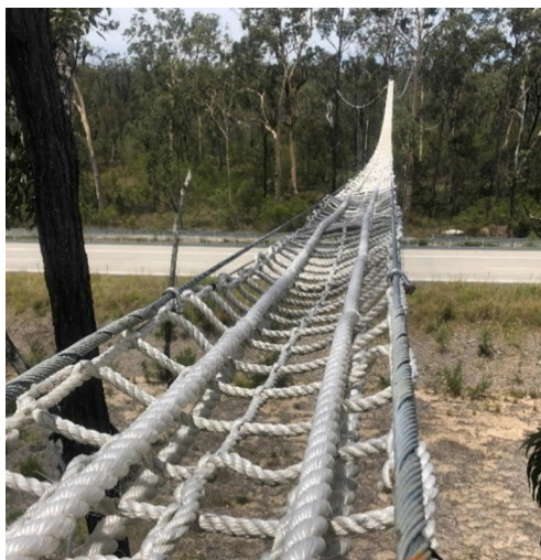
Plate 1: Rope bridges were suspended >10m above the road deck (upper) and supported by poles adjacent to the forest edge. The mesh ladder design included two 20mm thick ropes running the length (lower left). A camera was strapped to the bulkhead at each end of the bridge (lower right).
