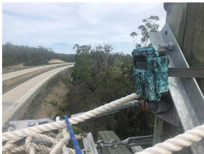
Plate 1: Rope bridges were suspended >10m above the road deck (upper) and supported by poles adjacent to the forest edge. The mesh ladder design included two 20mm thick ropes running the length (lower left). A camera was strapped to the bulkhead at each end of the bridge (lower right).
