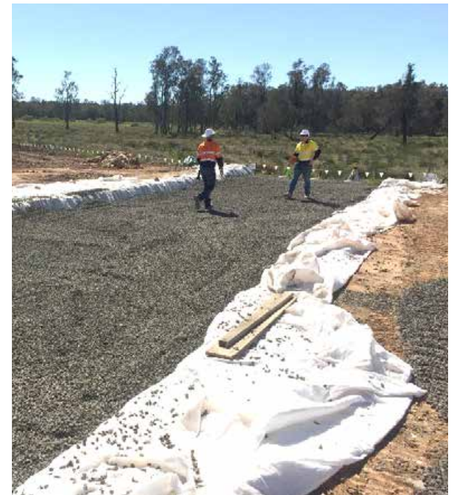
Installation of temporary drainage lines on the southern embankment (September 2016)
