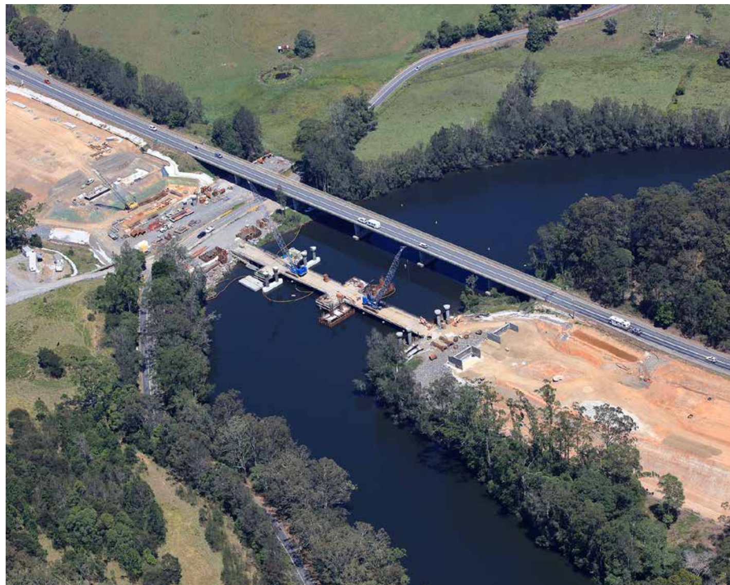
Aerial view of the Warrell Creek to Nambucca Heads upgrade – piling in the lower Warrell Creek (November 2016)
