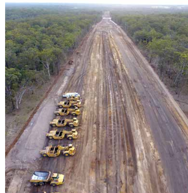
The scraper fleet was ready to start in October following clearing works at Wave 5A, between Glenugie and Tyndale
