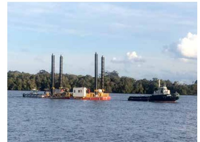
Work is in progress for a new bridge over the Clarence River at Harwood with geotechnical investigations under way (November 2016)
