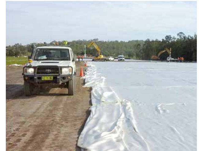
High strength fabric installation at Maclean
