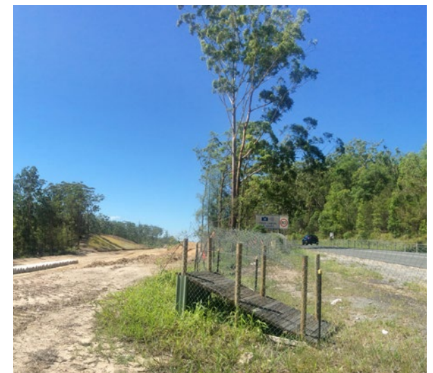
Temporary floppy top fencing and a koala drop down installed on the Nambucca Heads to Urunga project
