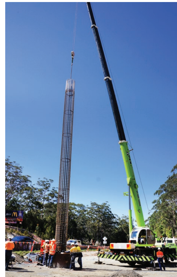
A standing piling cage on the western side of the Pacific Highway (November)
