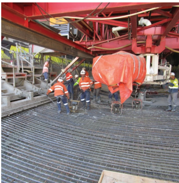
Tintenbar to Ewingsdale - pouring concrete at the southern tunnel portal
