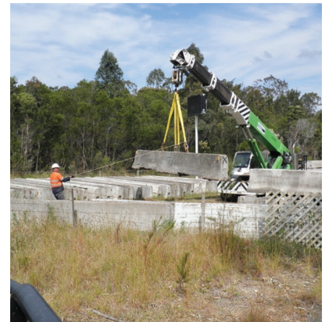
Installing barriers on the Pacific Highway
