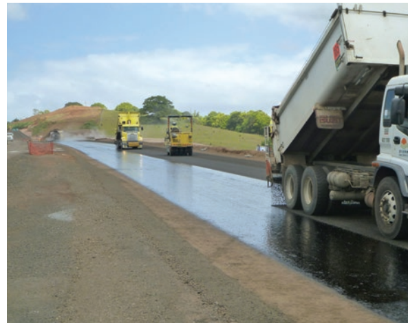
Tintenbar to Ewingsdale upgrade – A spreader truck applies aggregate to the next bitumen seal run on the northbound carriageway
