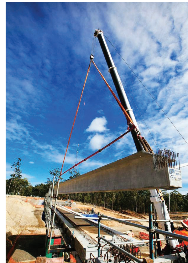
Nambucca Heads to Urunga project – A girder being placed for the Ballards Road overbridge (August)
