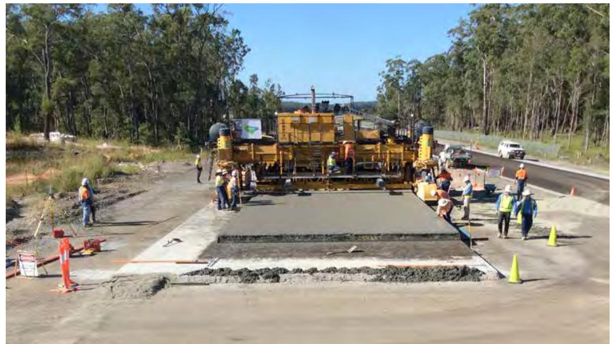
Work in progress to place mainline concrete paving, just north of the Hastings River, Oxley Highway to Kundabung project (March 2016)
