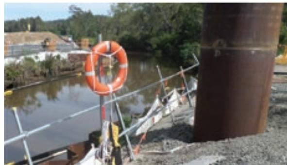
The working platform built to improve safety for workers welding piling casings on the Pimlico to Teven project
