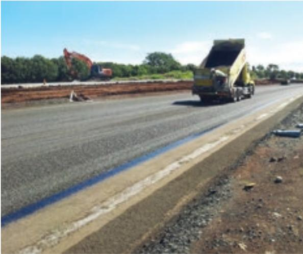
Tintenbar to Ewingsdale upgrade - road sealing work on northbound lanes at Martins Lane, Knockrow
