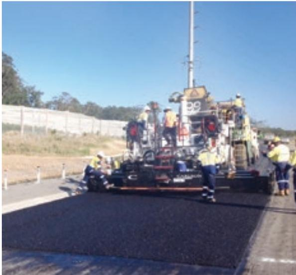
Sapphire to Woolgoolga upgrade - laying of the low noise road surface on the new highway south of Woolgoolga
