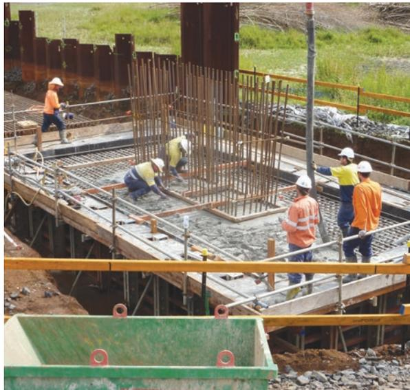
Tintenbar to Ewingsdale upgrade – concrete being poured for bridge at Minor Creek
