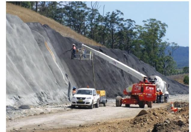
Bulahdelah upgrade – rock bolting work north of Bombah Point bridge
