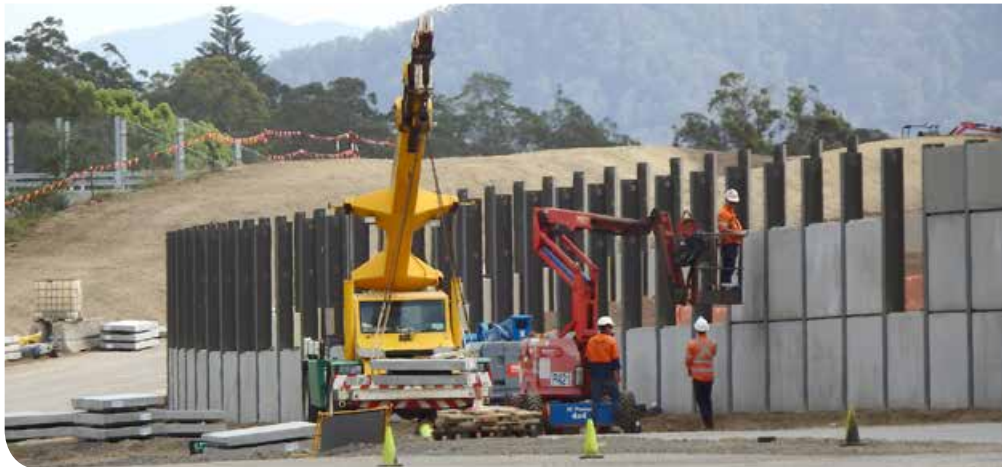
Building the acoustic wall between Bald Hill Road and Lower Warrell Creek
