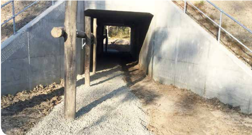
Fauna furniture installed in a fauna connectivity underpass
