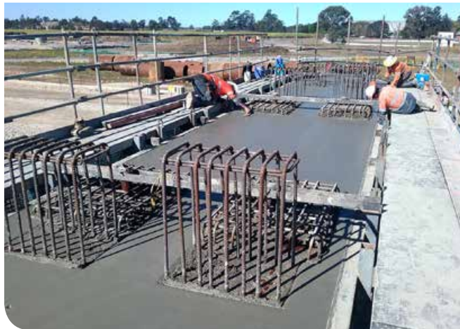
Concreting the bridge headstock
