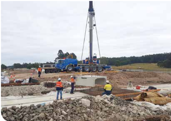
Installing pre-cast concrete drainage culverts at Banana Road
