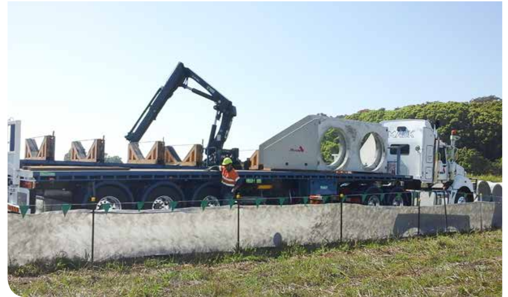
Delivery of precast concrete headwalls for cane drain crossings
