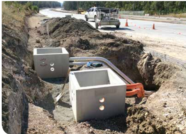
Installing electrical and communications pits for Point to Point speed cameras, near Blackmans Point Road
