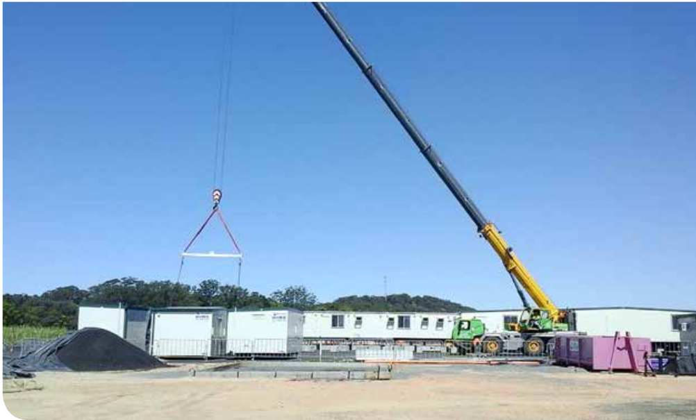
Using a crane to position site office buildings
