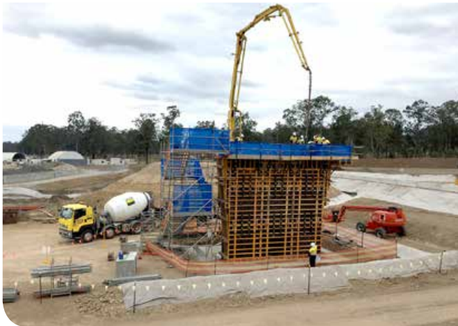
Concreting the centre pier of a bridge at Tyndale
