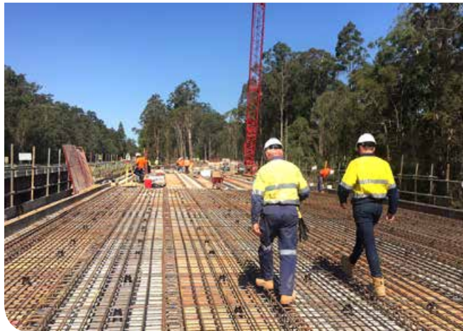
Preparing the bridge deck for the first concrete pour, at Tabbimoble Creek
