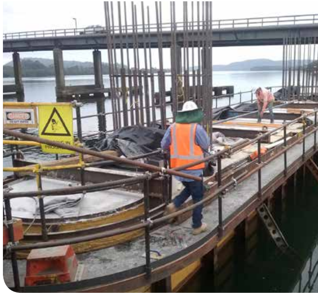
Concreting the first marine bridge pile cap
