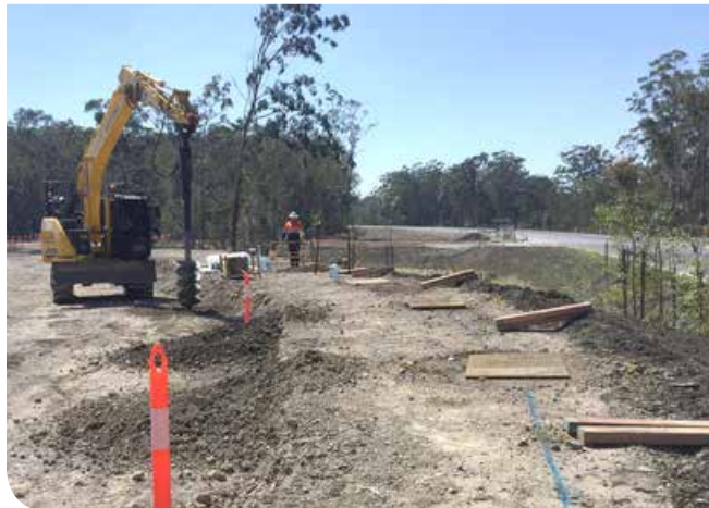
Drilling holes for noise wall posts, Arrawarra rest area
