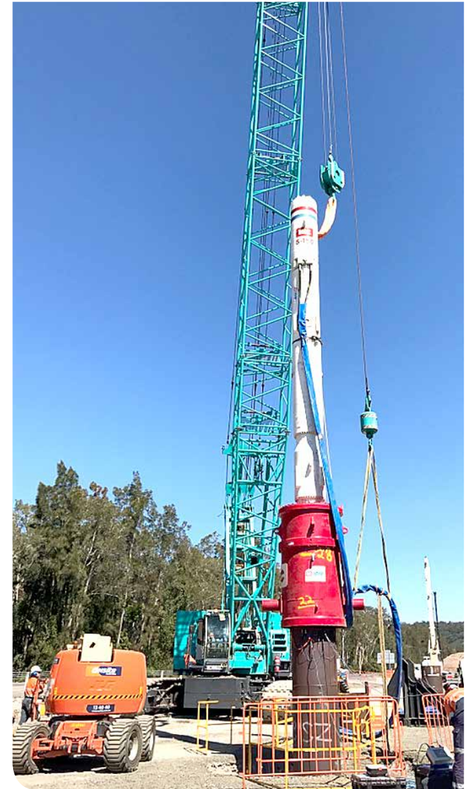
Driving land piles for the bridge north of Maclean
