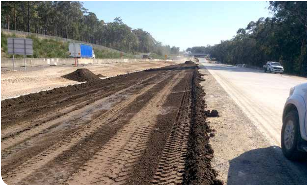
Topsoil being placed in central median near Blackmans Point Road
