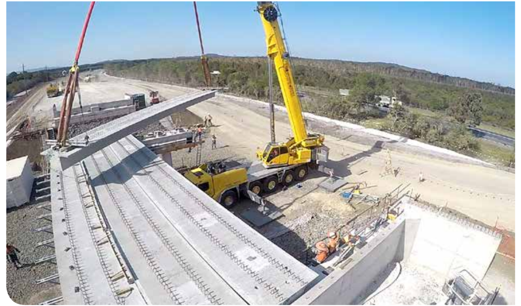
Using crane to place concrete bridge girders on a service road
