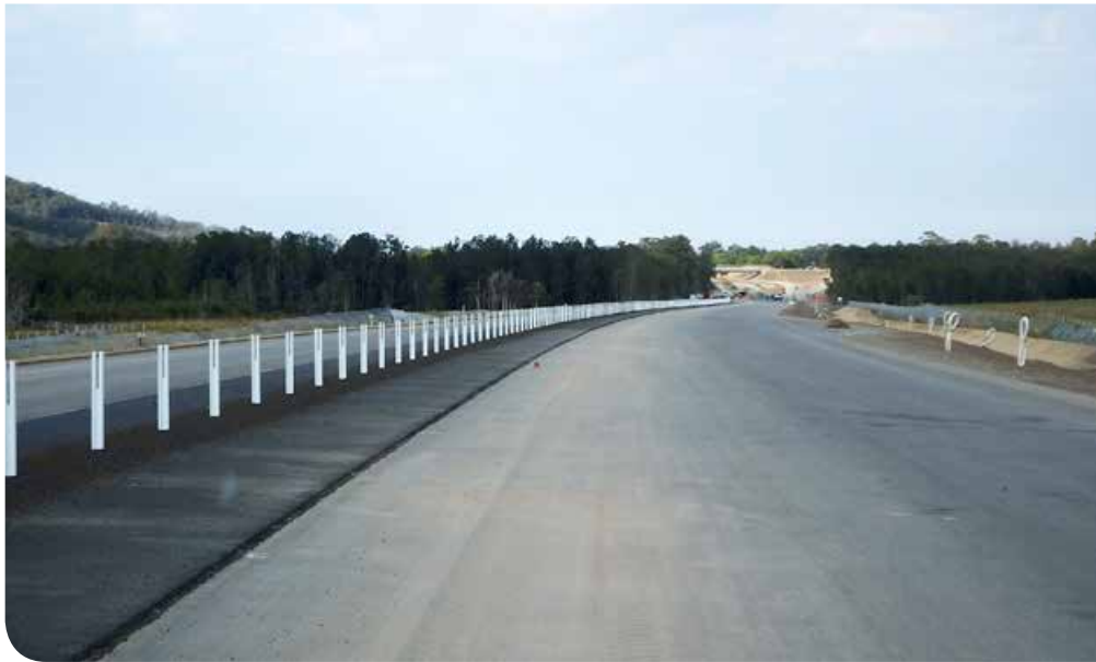
Wire rope barriers being installed in the flood plain area south of Nambucca River bridge
