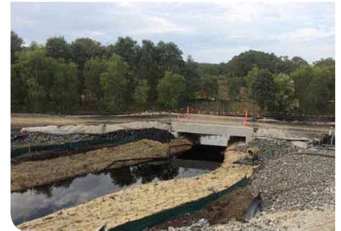
Bank stabilisation work in endangered fish habitat to protect the Oxleyan Pygmy Perch
