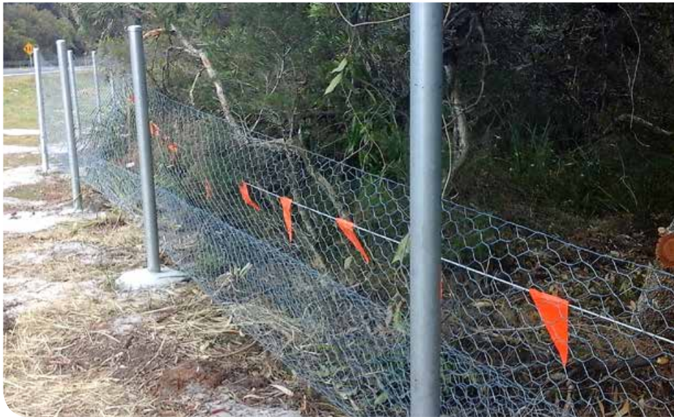
Fauna exclusion fencing being installed along the existing Pacific Highway Coolgardie Road
