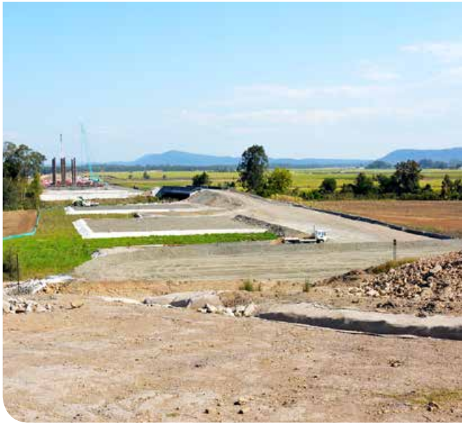
Bridge piling pads at Shark Creek, near Tyndale
