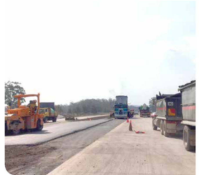
Placing asphalt in emergency turn around area north of Kangaroo Trail Road
