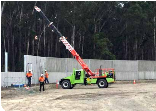
Installing noise wall panels, Arrawarra rest area
