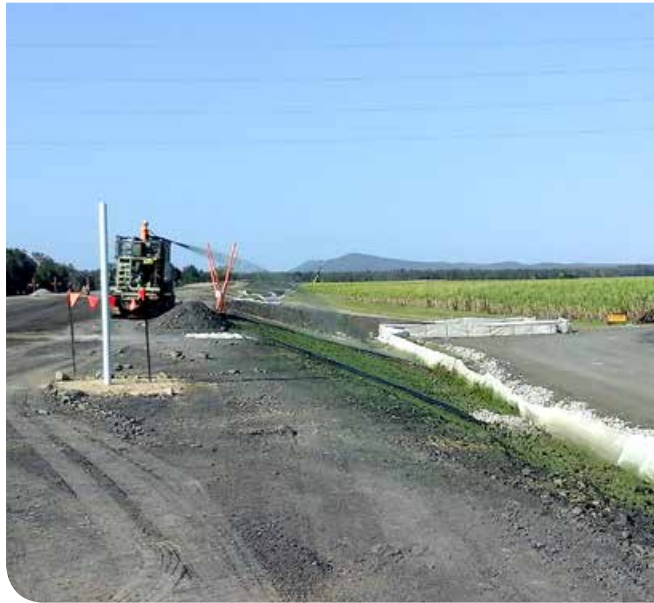
Hydromulching at Shark Creek, near Tyndale
