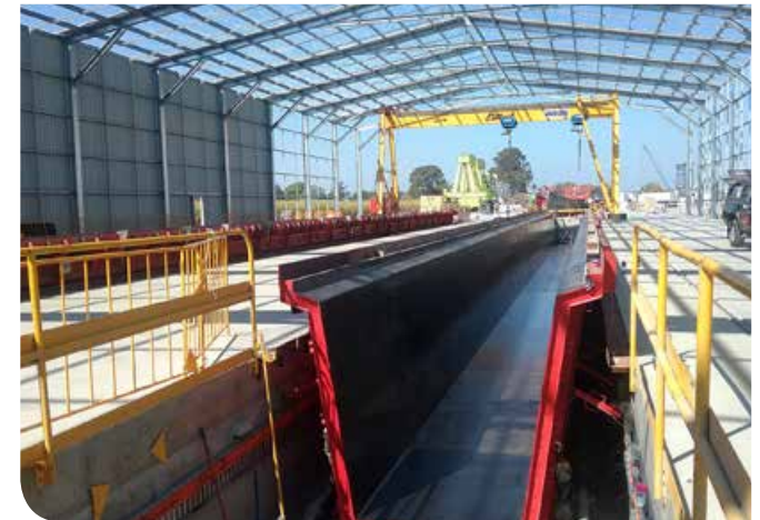
Preparing the formwork for pre-cast bridge girders
