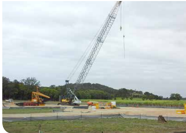
Crane in place to lift the piling rig in place
