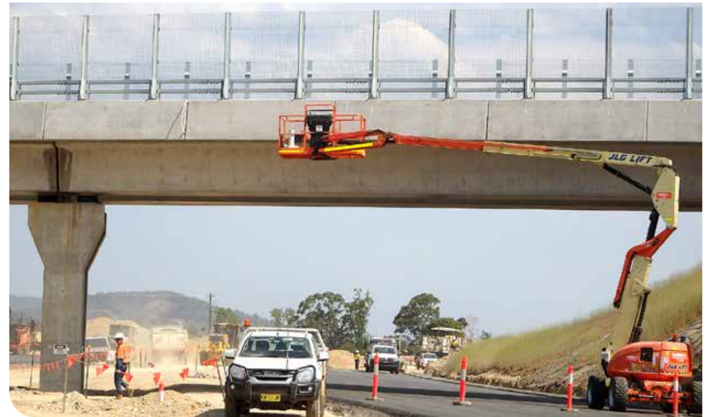
Installing underbridge drainage at the southern Old Coast Road bridge
