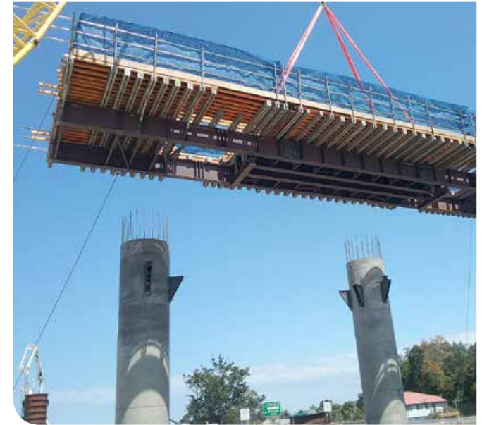
Using a crane to position the frame for bridge headstock
