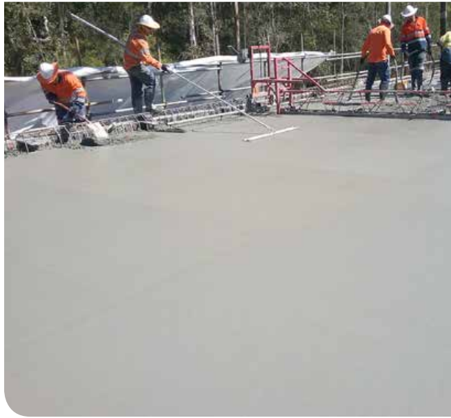
Concreting the bridge deck at Tabbimoble Creek
