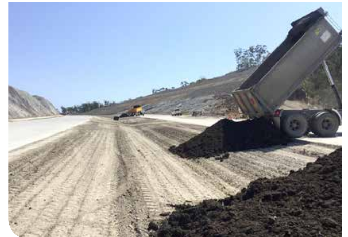
Placing topsoil in median at Dirty Creek Range
