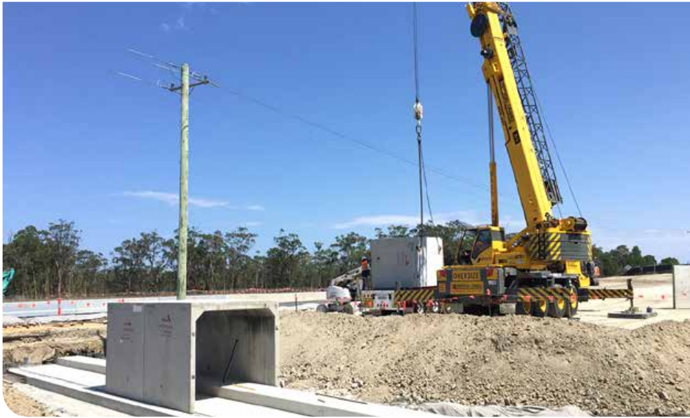
Installing a concrete drainage culvert on a service road
