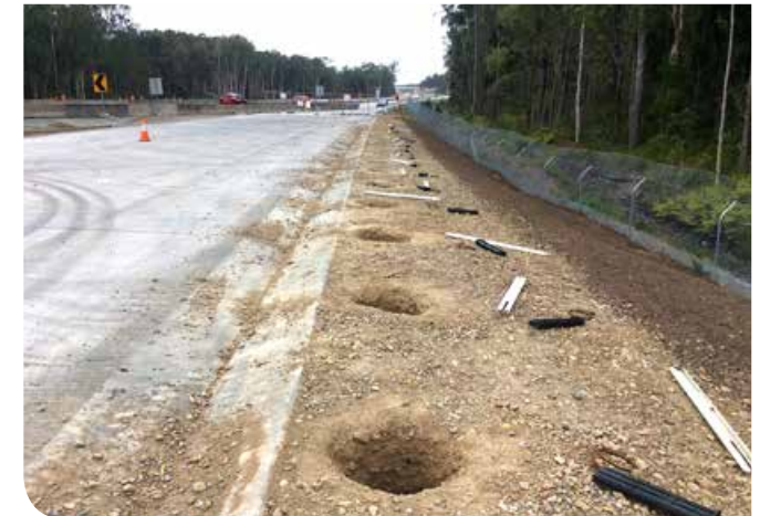
Preparing holes for concreting wire rope safety barrier posts, near Fernbank Creek
