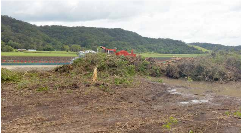
Sorting of cleared vegetation in preparation for commencement of mulching operations and off-site disposal
