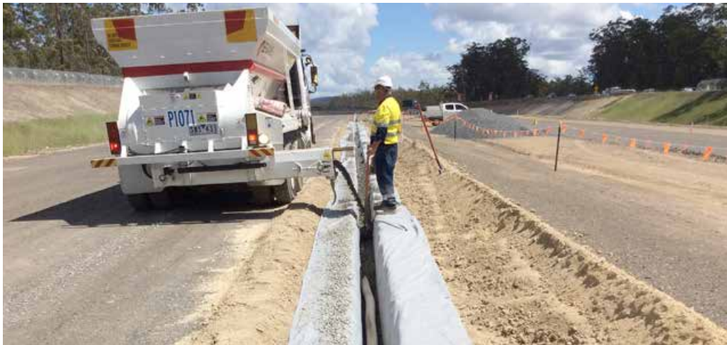
Subsoil drainage trench being installed near Blackmans Point Road interchange
