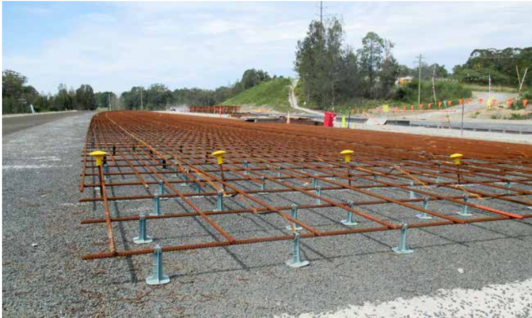
Concrete pavement steel north of Short Cut Road
