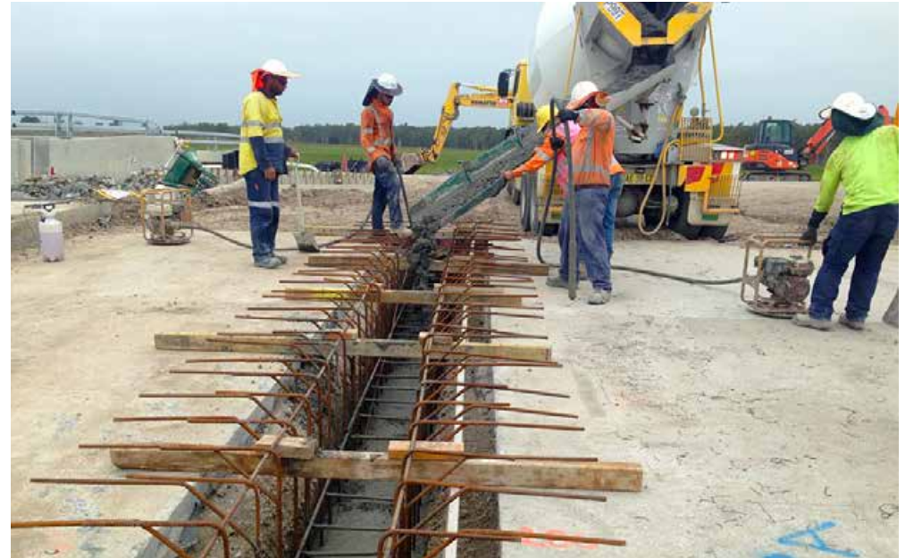
Hand pour for concrete pavement anchor, adjacent to bridge over Collombatti Creek, looking east
