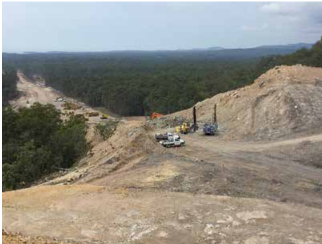
Drilling for blasting on the Dirty Creek Range looking south
