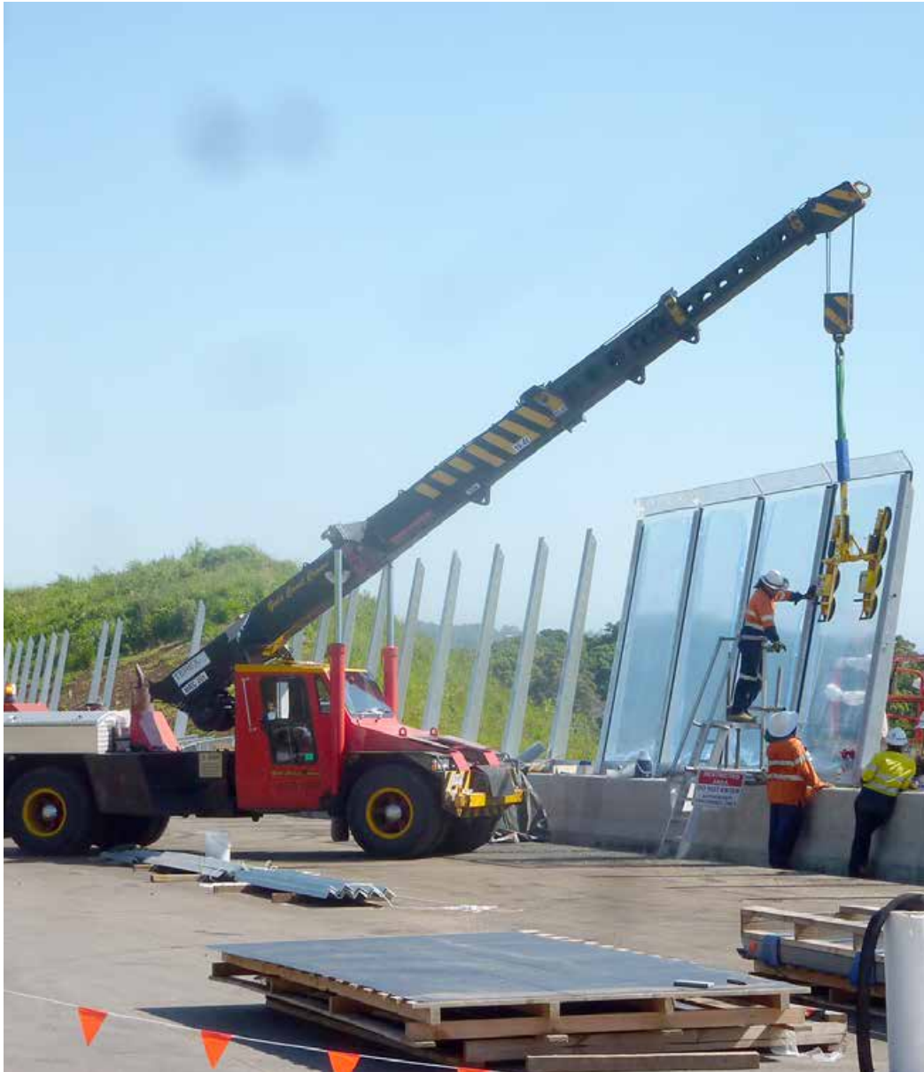
Noise wall installation at St Helena
