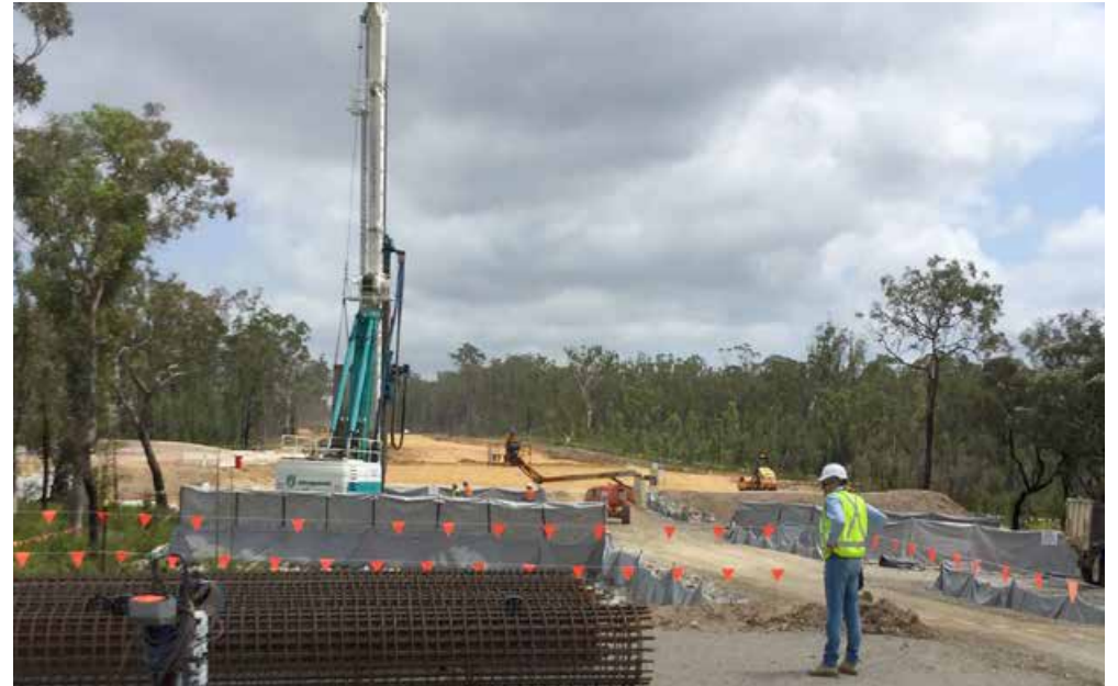
Start of Piling work at Wells Crossing
