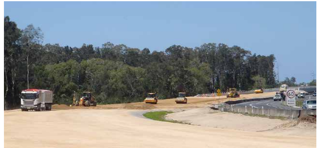
Placing road pavement south of Duck Creek
