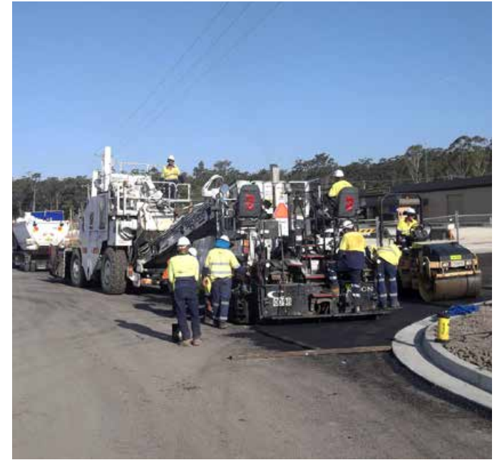
Placing asphalt on Sancrox Road
