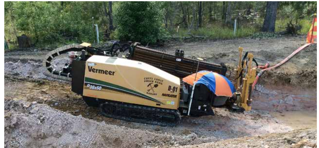
Underbore work near Blackmans Point Road interchange
