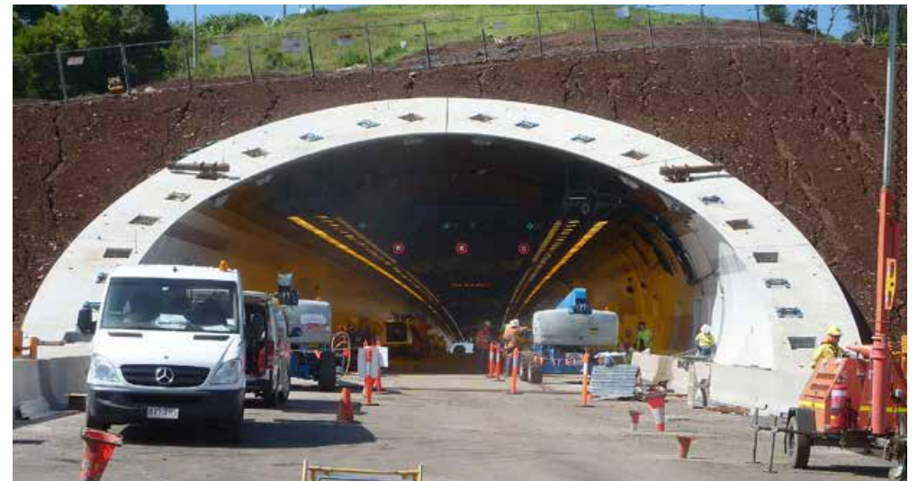
Tunnel portal collar installation
