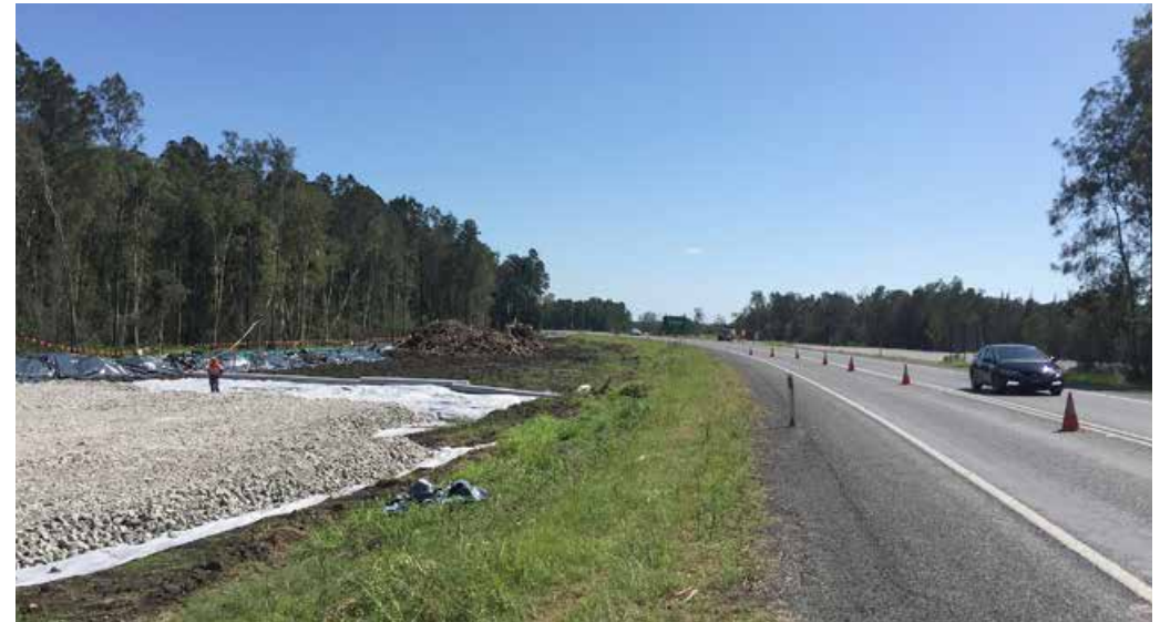
Installing drainage rock
