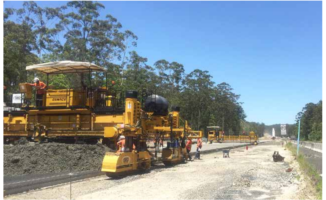
Concrete paving work underway
