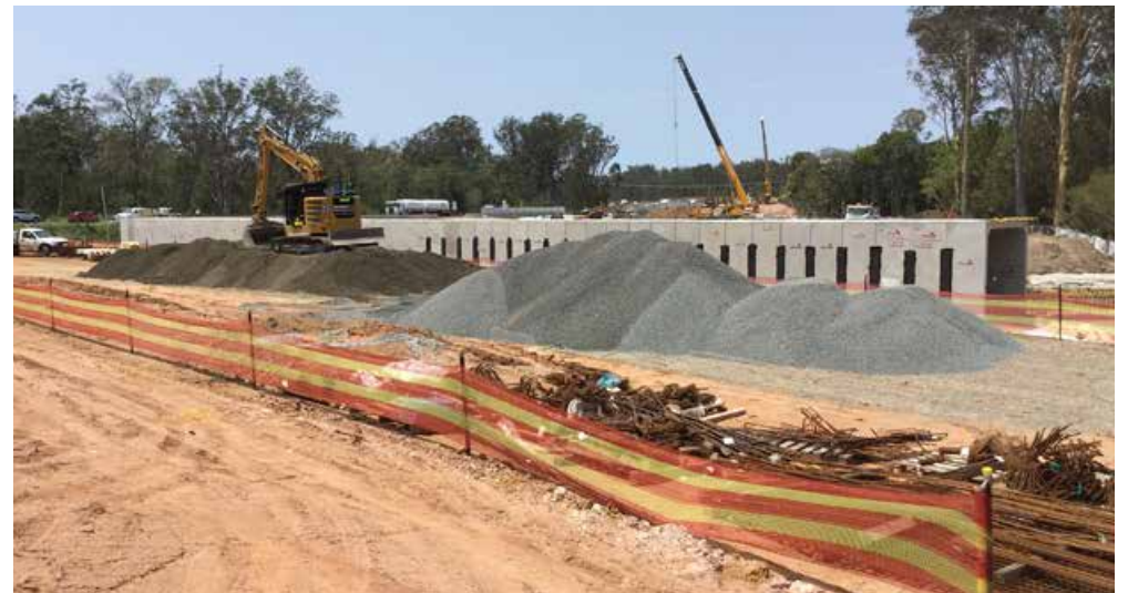
Installation of culvert units
