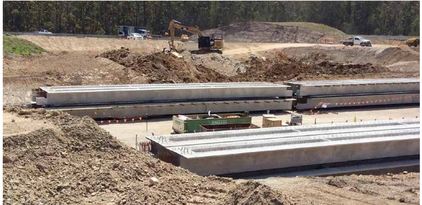
Bridge girders delivered to site ready for erection at the new Blackmans Point Road interchange
