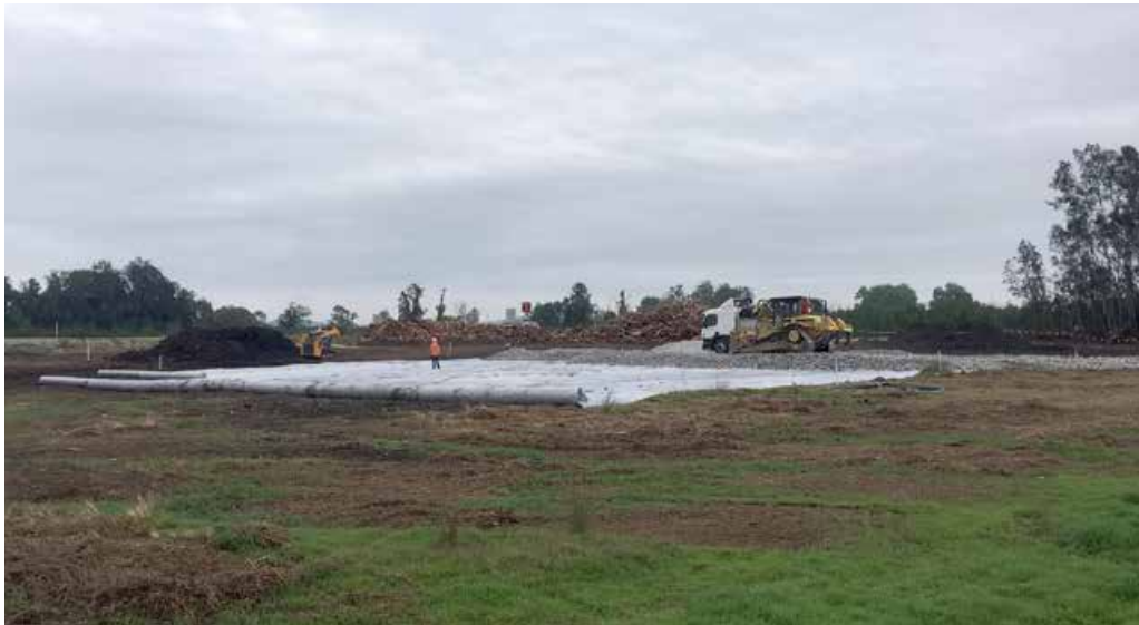
Installation of geofabric in preparation for drainage rock
