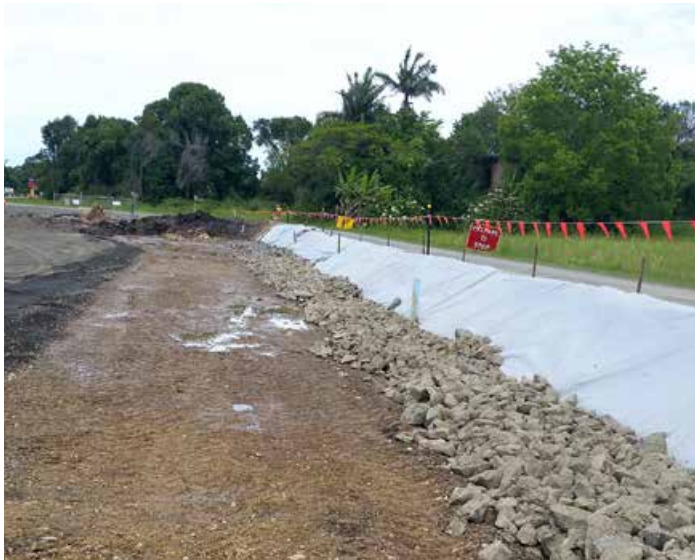
Sediment control in place
