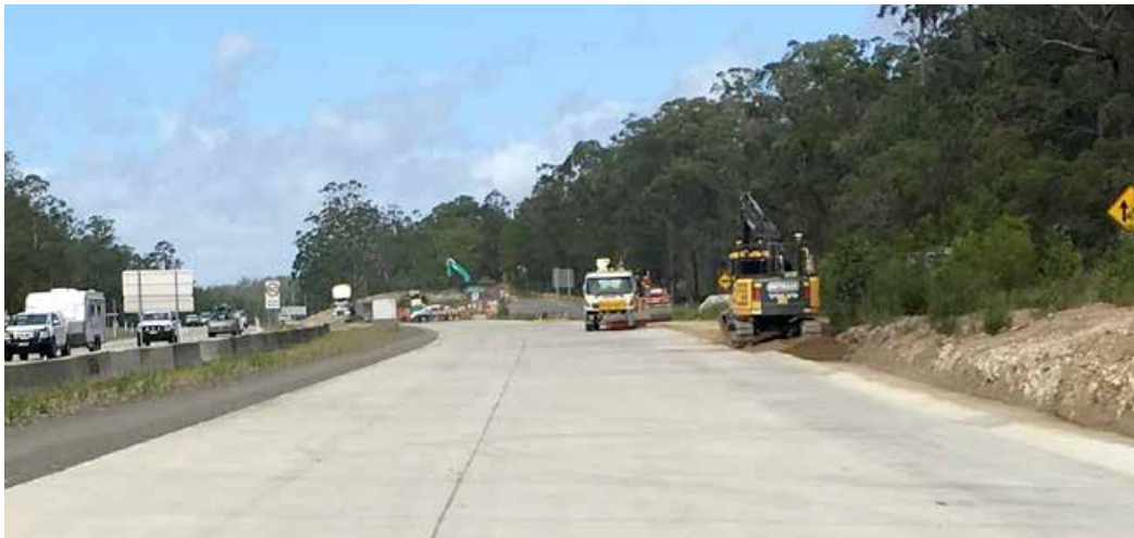
Verge placement, south of Stumpy Creek
