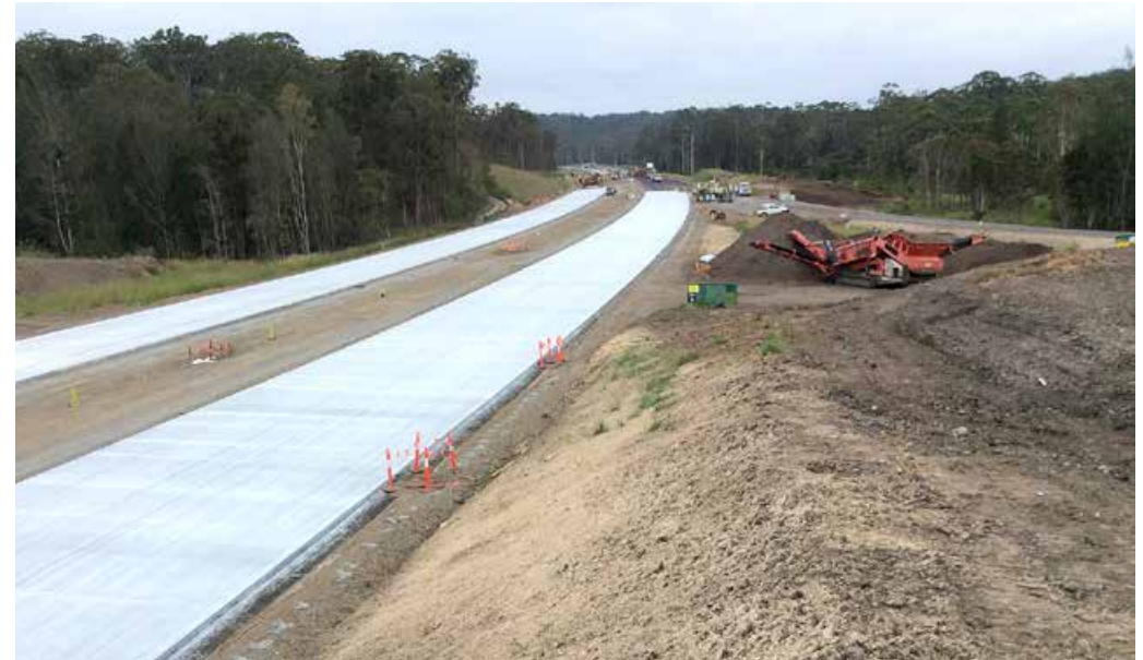
Concrete paving north of Haydons Wharf Road
