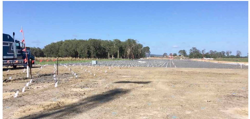
Soil wick was installed at the additional soft soil area
