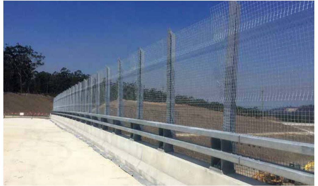
Safety screen installation at Range Road overpass bridge
