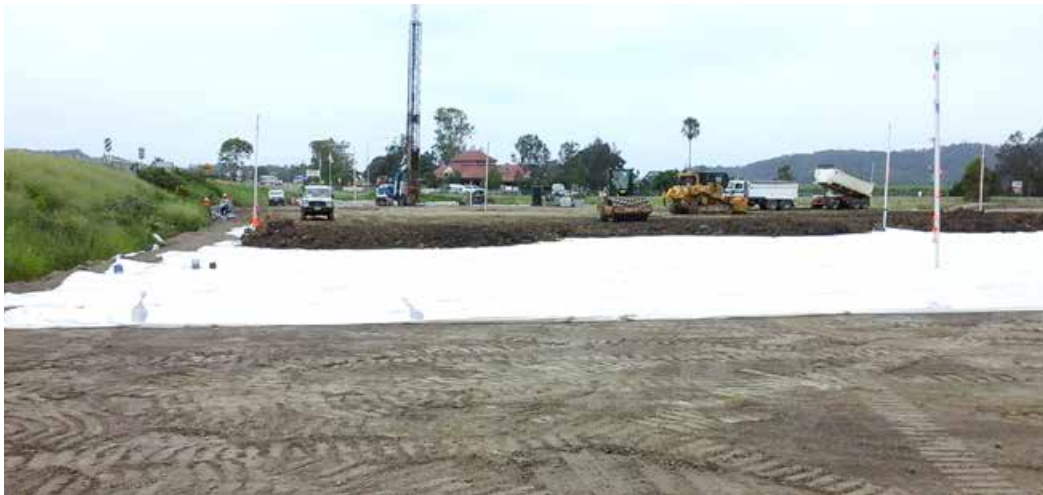
Placement of fill over high strength fabric, north of Edwards Drain
