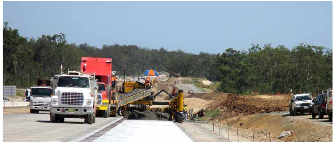
Shoulder paving, southbound carriageway, north of Lemon Tree Road
