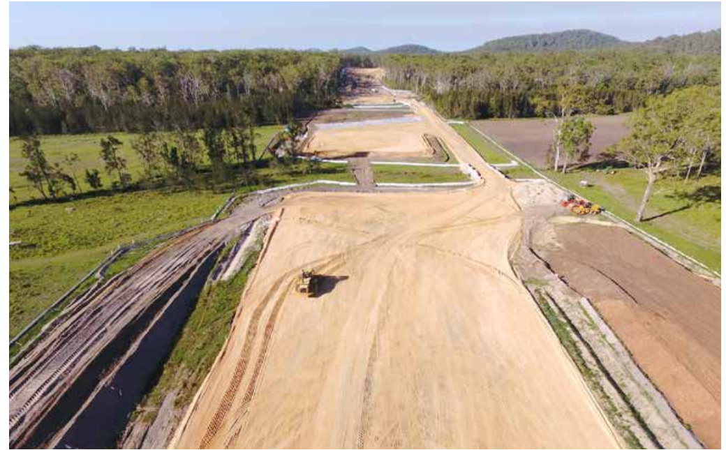
General fill at embankments at Pillar Valley
