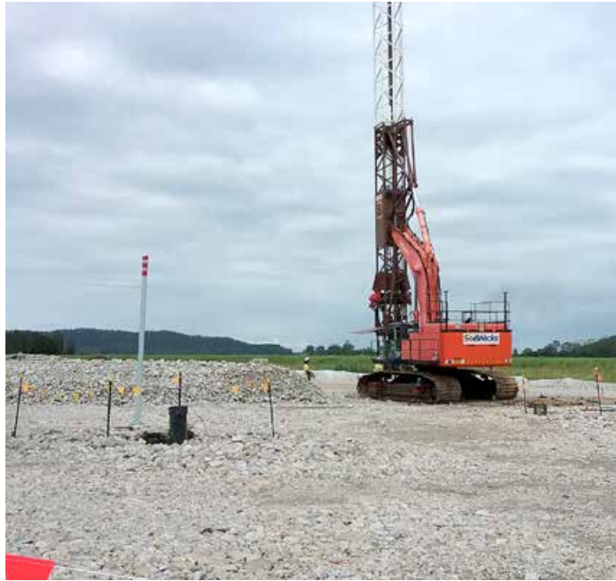
Installation of soil wick at Lees Drain
