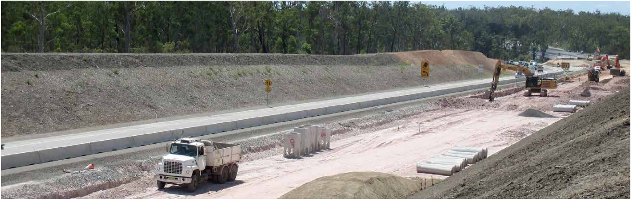
Drainage work, southbound carriageway, south of Wells Crossing
