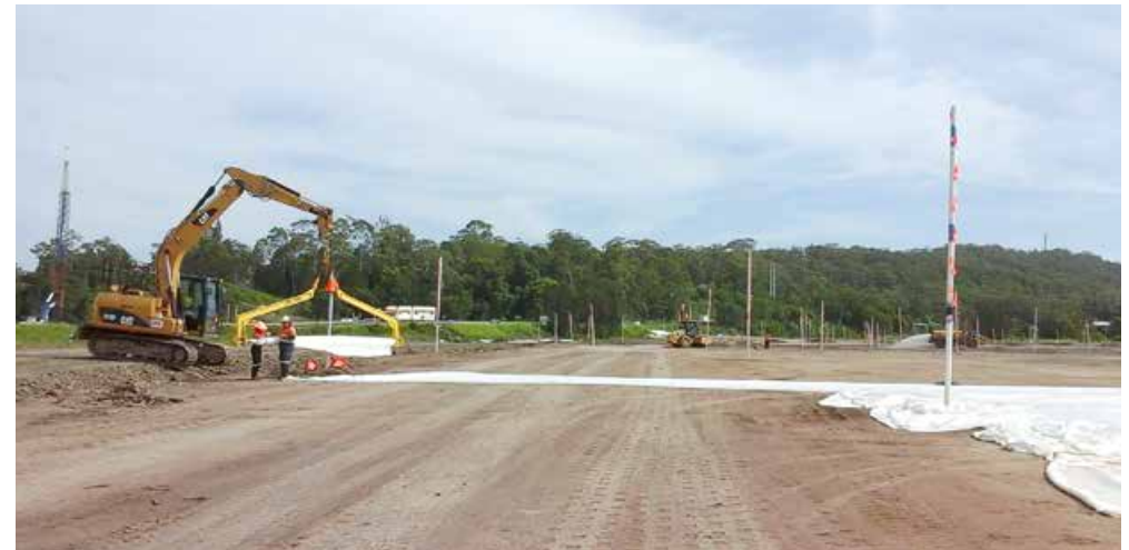
Rolling high strength material, north of Edwards Drain
