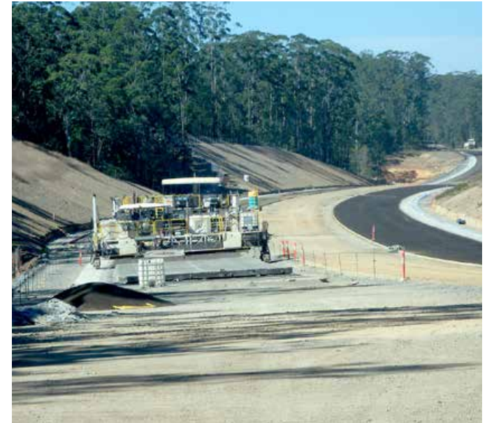
Concrete paving machine, north of the Nambucca River
