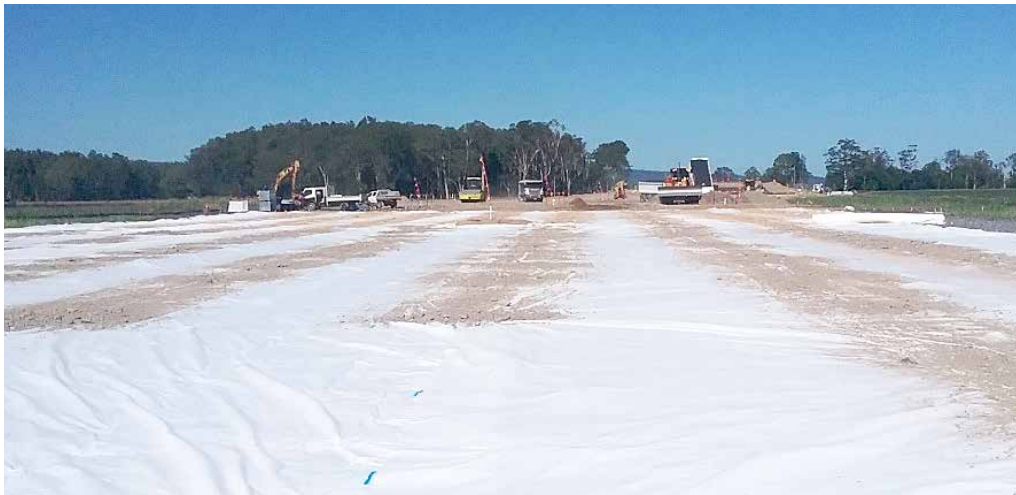
Separation fabric was placed on top of wick rock
