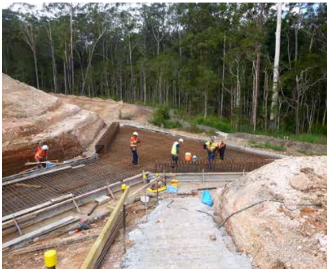
Placing reinforcing steel for a large box culvert under the highway south of Fernbank Creek Road
