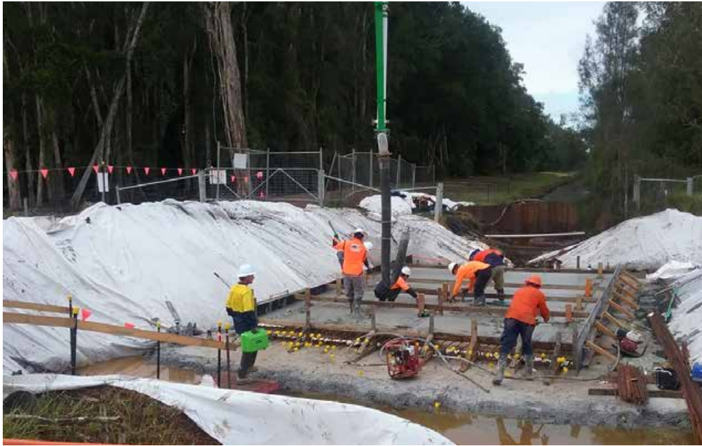
Pouring the base slab for underpasses in the town drain
