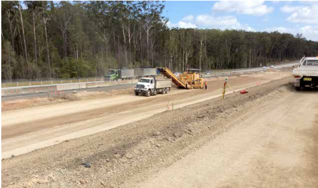
Trimming sub-grade layer south of Fernbank Creek
