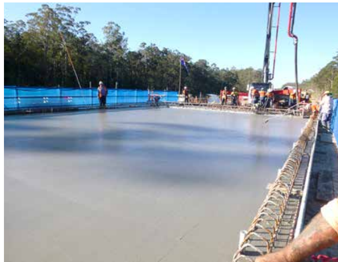
Pouring concrete deck at Barrys Creek northbound bridge
