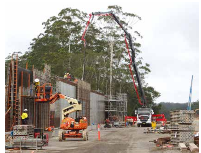
Pouring side walls for the railway overpass at Warrell Creek
