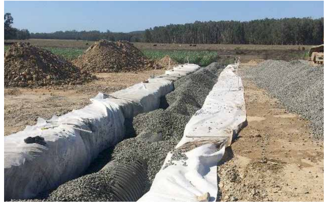
Installation of temporary drainage lines
