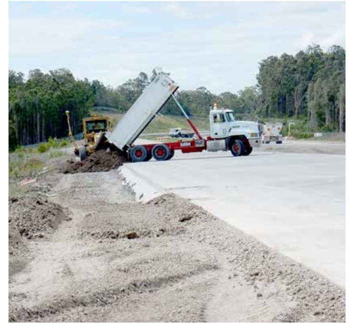
Verge material being placed south of Seven Hills Road
