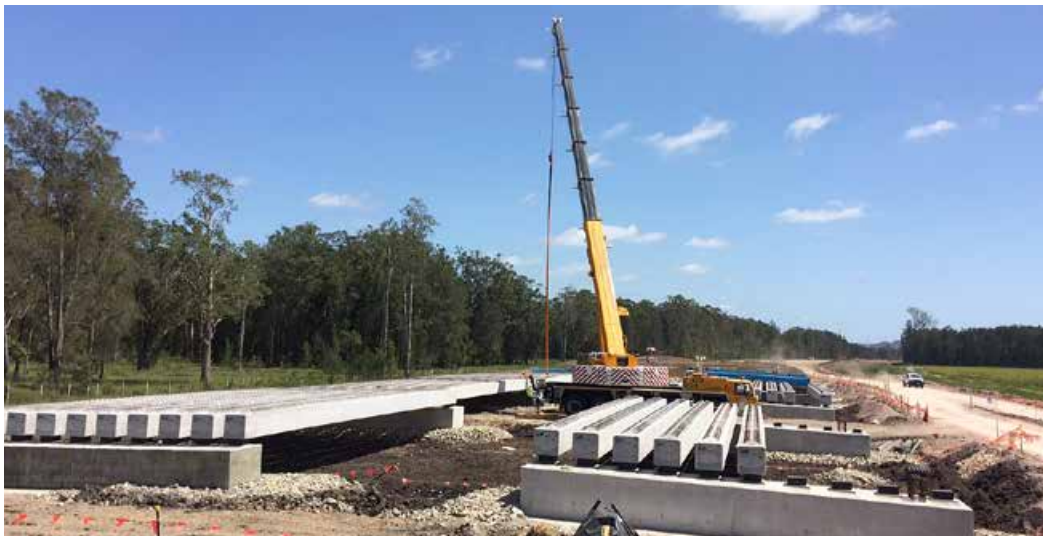
Placing precast bridge planks on one of the Wilson River floodplain bridges
