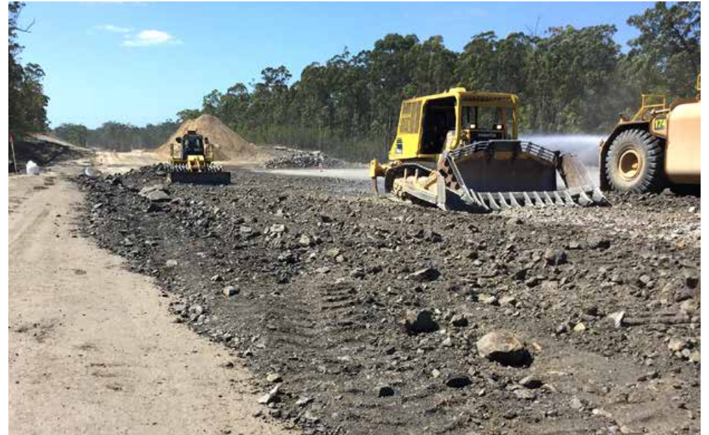
Placing fill at the base of Dirty Creek Range
