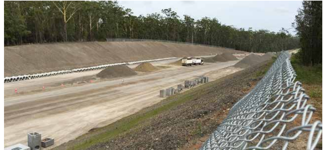
Topsoiling batters work near Bloodwood rest area
