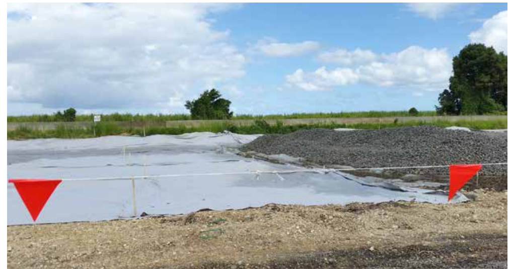
Geofabric installed in preparation for laying of drainage rock
