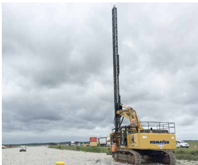
Wick drain construction for wave 1 soft soil work
