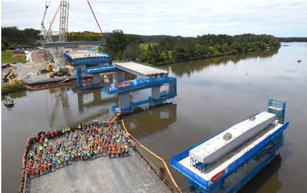
Girder installation on the Wilson River bridge
