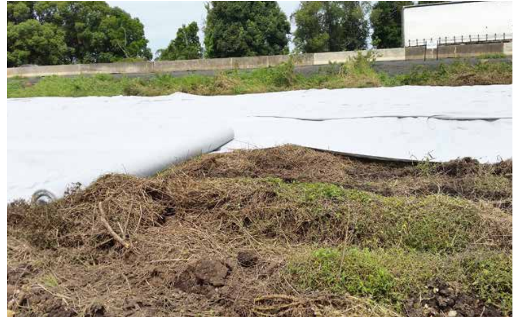
Installing geofabric, following completion of tree clearing and grubbing work
