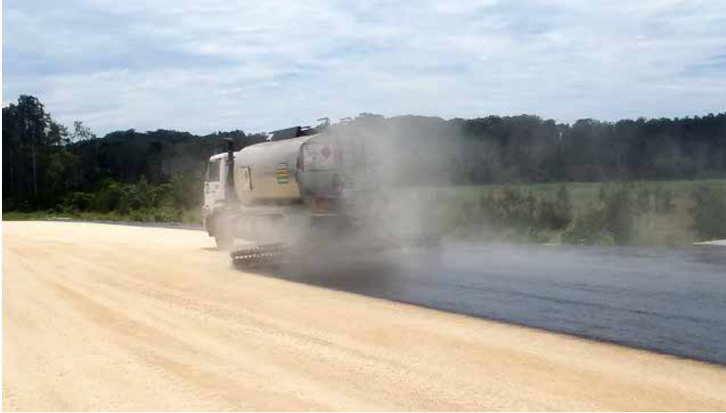
Spraying bitumen prime on the pavement south of Duck Creek
