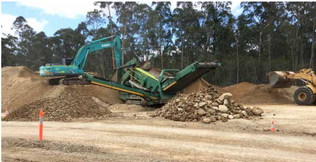
Screening earthworks to make culvert backfill material
