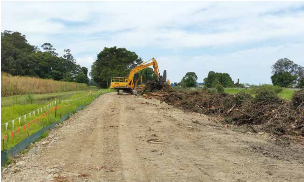
Clearing and grubbing work in progress
