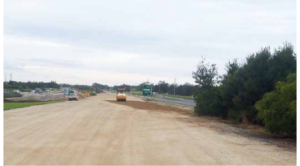
Placing road pavement north of Emigrant Creek
