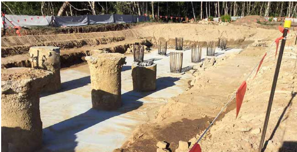
Piles in place at Halfway Creek bridge
