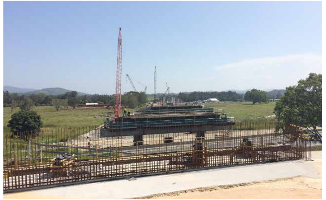
Girder installation at the Nambucca River pier
