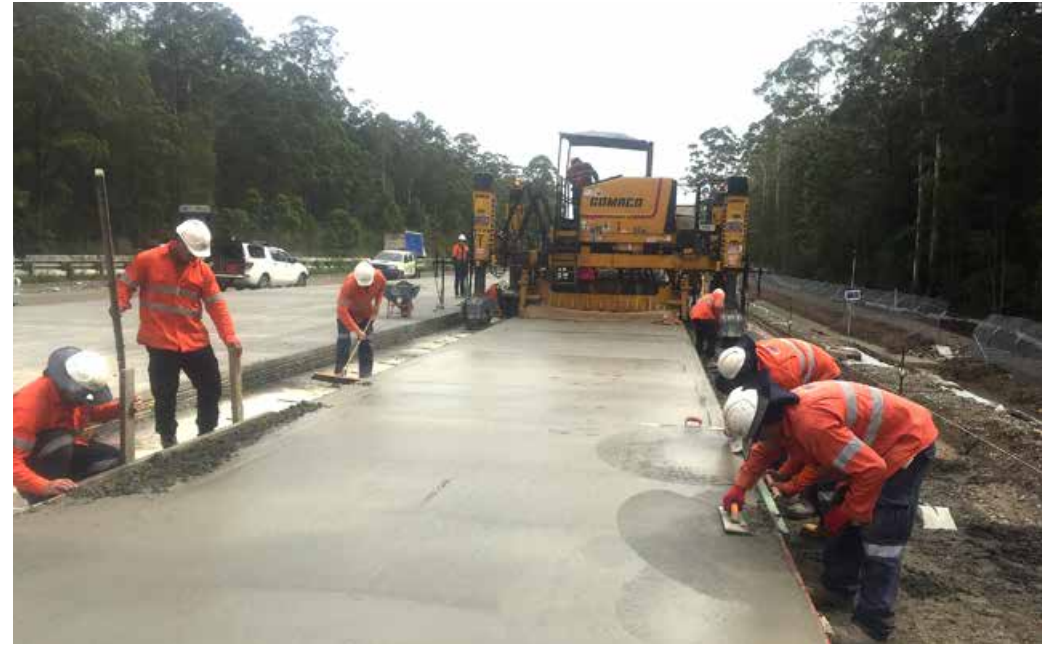
Concrete paving work near Barrys Creek
