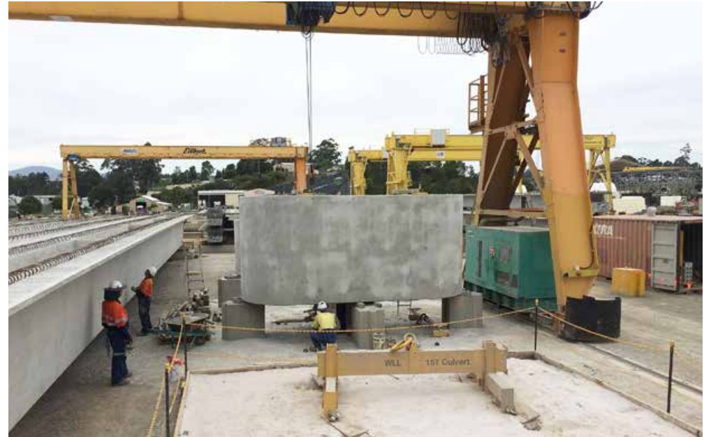
Precast pilecap tub prepared for the Hastings River bridge
