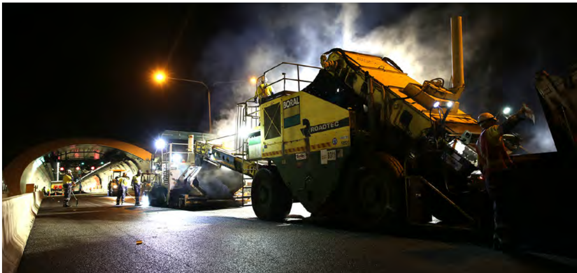
Placing asphalt near the southbound tunnel
