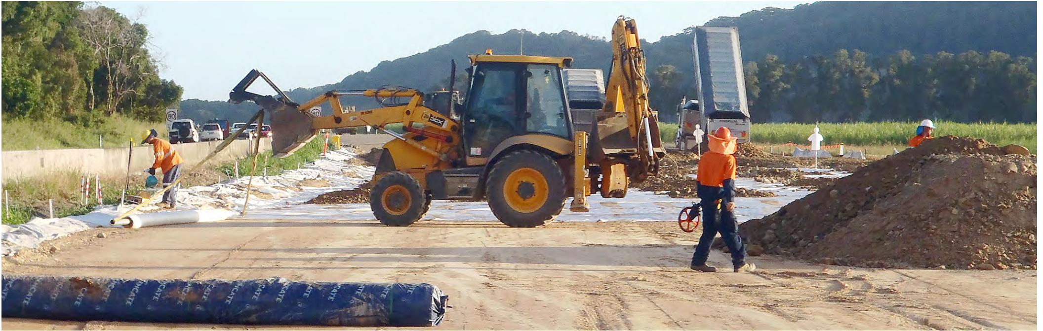
Installing high strength fabric as part of soft soil work
