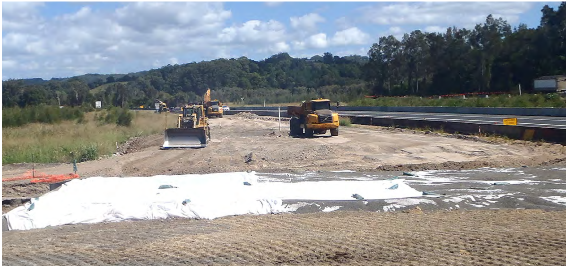
Work in progress to remove old road pavement south of Duck Creek
