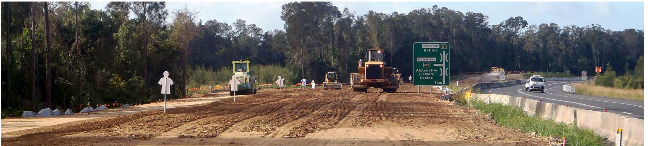
View of earthwork in progress, human form cut-outs in place to protect instrumentation.
