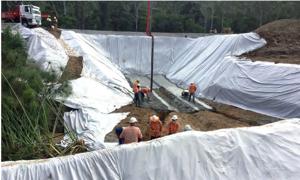
Concrete being placed for a large culvert at the northern end of the project
