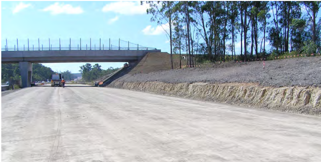
Placing select material under the Kundabung bridge looking north
