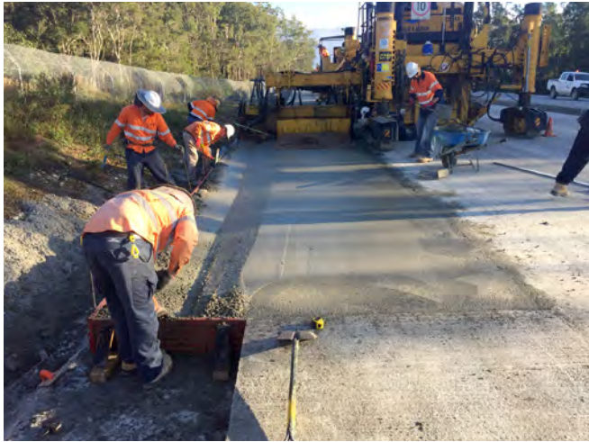
Paving the road shoulder incorporating a drain, just north of the Hastings River
