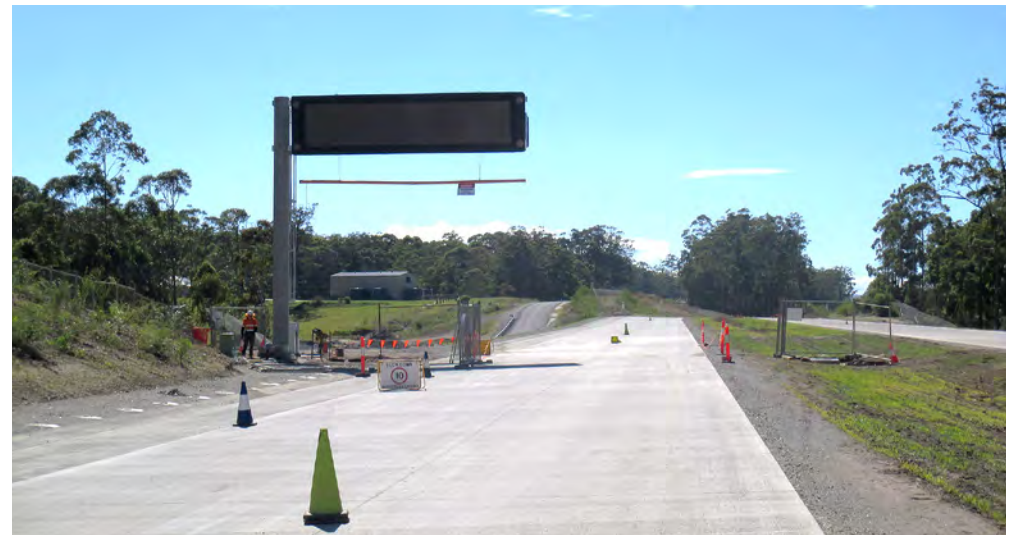
New variable message sign installed north of Burkes Lane
