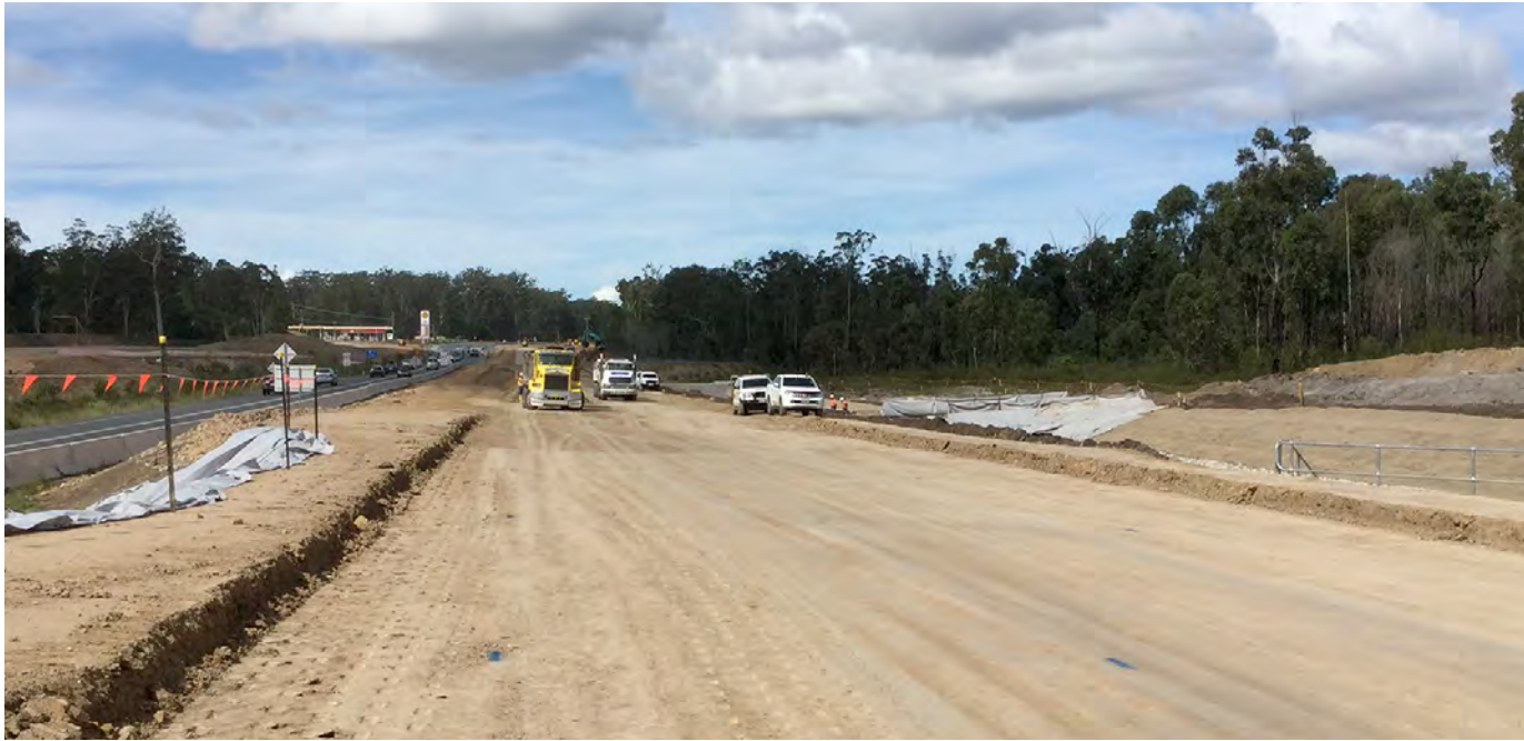
Placing select material for the northbound carriageway, near Lemon Tree Road
