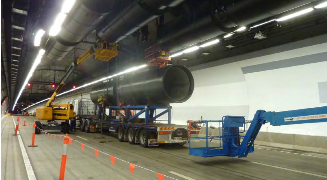
Jet fan repair work inside the tunnel
