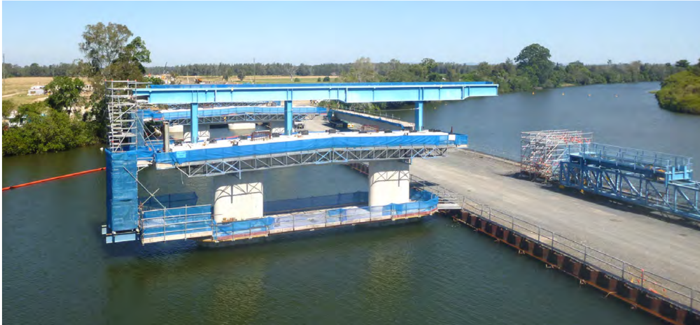
A view of the side lifting truss at the Wilson River bridge, to lift precast concrete girders onto the headstocks
