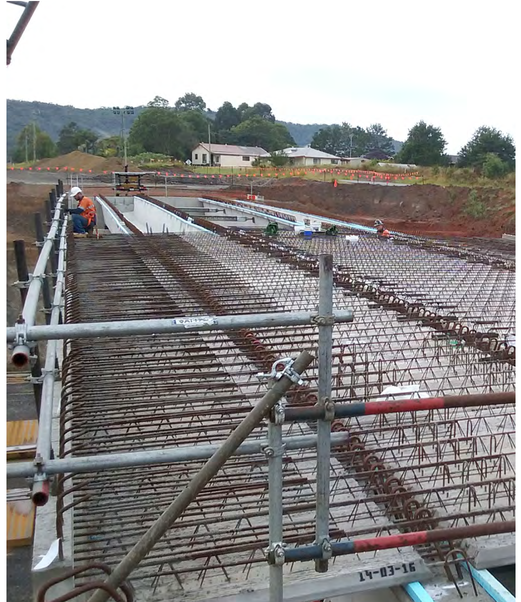
Pre-cast concrete floor panels being placed on the Bald Head Road bridges
