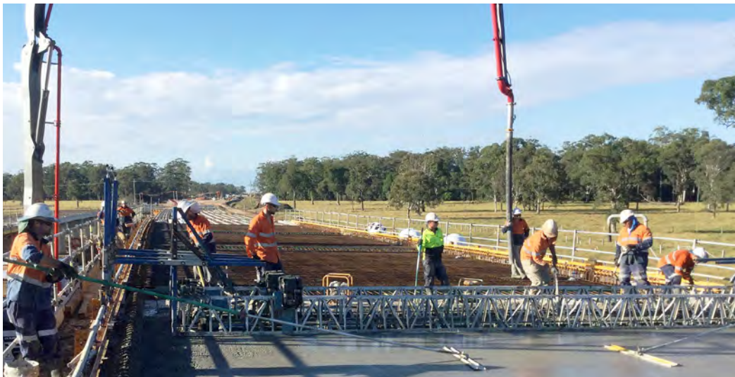
Placing concrete for the northbound deck of Corindi floodplain bridge
