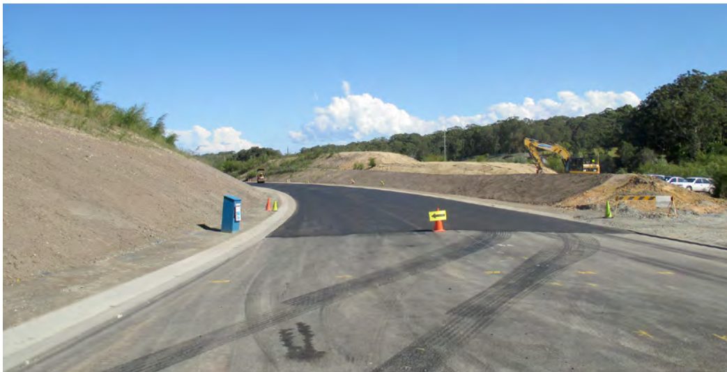
Ramp asphalt work at the Waterfall Way interchange
