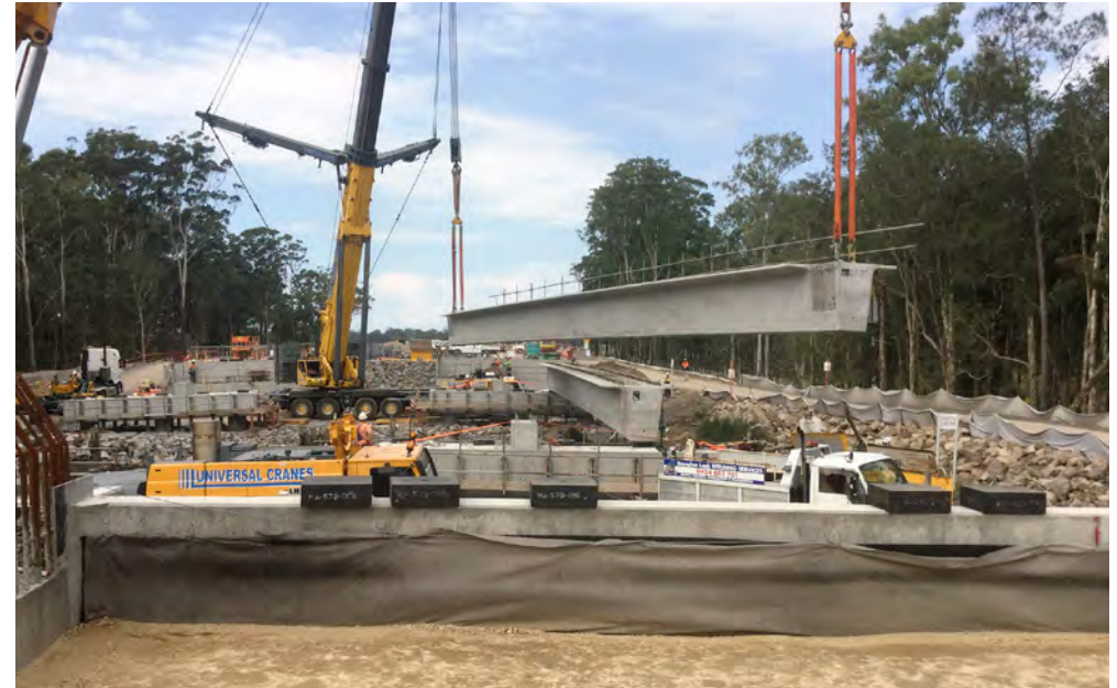
Concrete bridge girder being lifted into place at Cassons Creek
