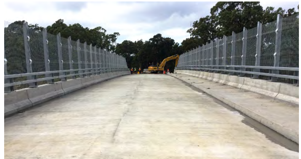
Sherwood Creek overbridge ready for asphalt deck placement
