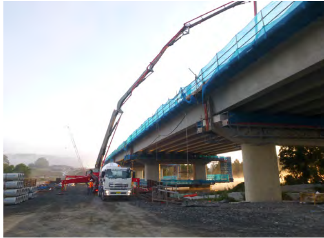
Concrete being poured for the Wilson River bridge
