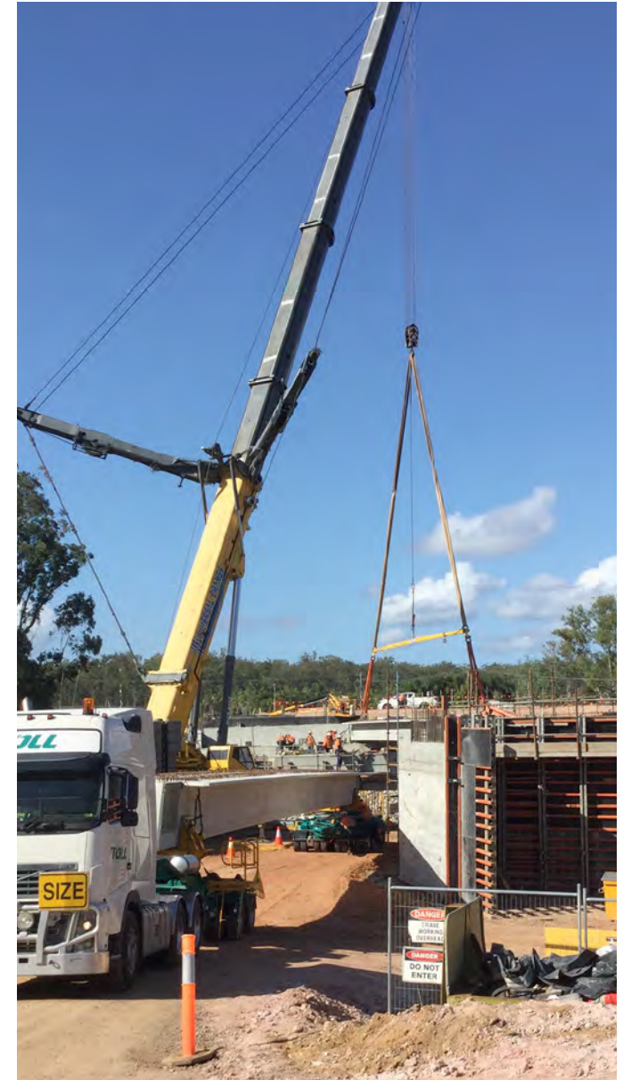
Concrete bridge girders being installed for the Halfway Creek bridge
