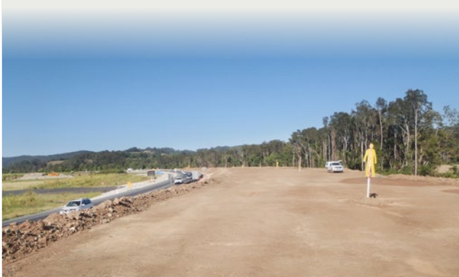
The 13 month settlement period has started on the wick drain embankment south of Duck Creek
