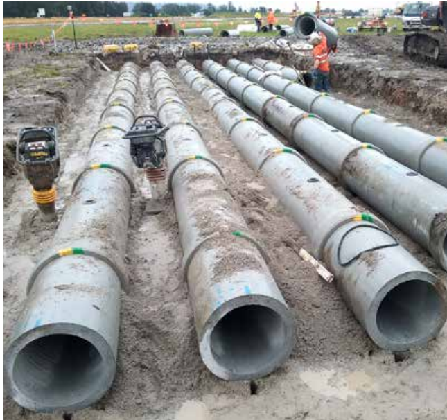
Installation of culverts over the northern section of the project
