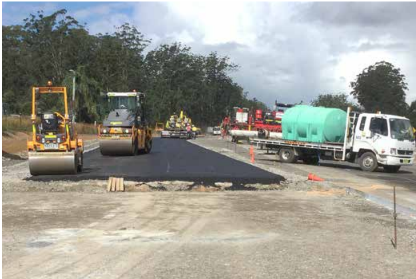
Asphalt paving service road near Lemon Tree Road
