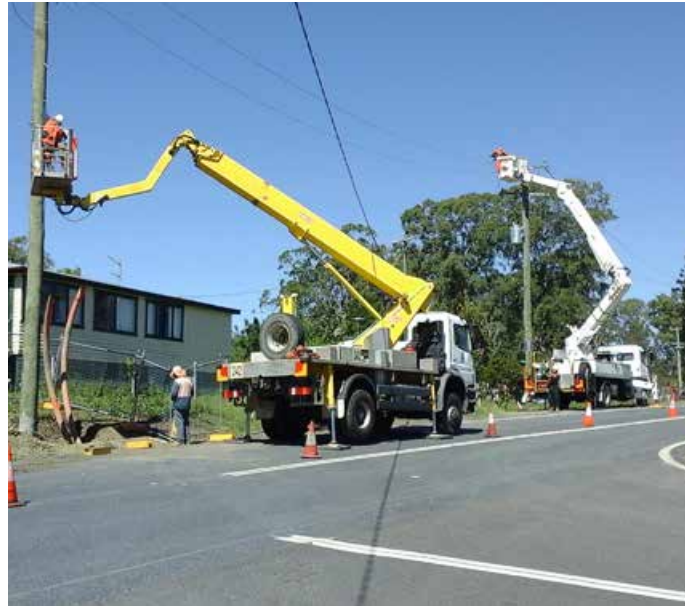
Cable pulling for electrical network relocations at Gap Road, Woodburn
