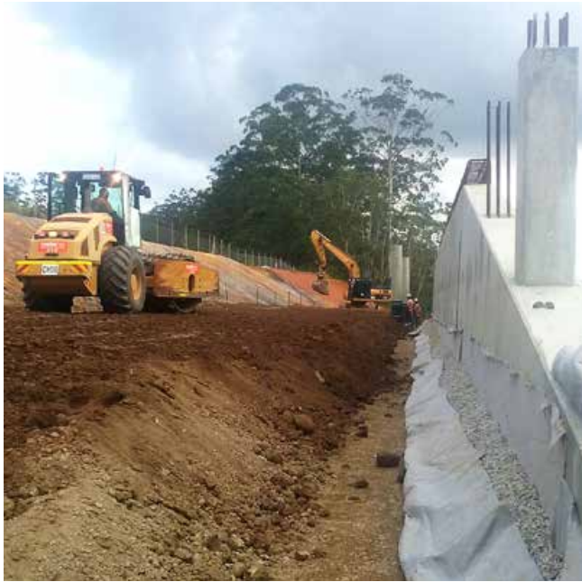
Backfilling the railway underpass
