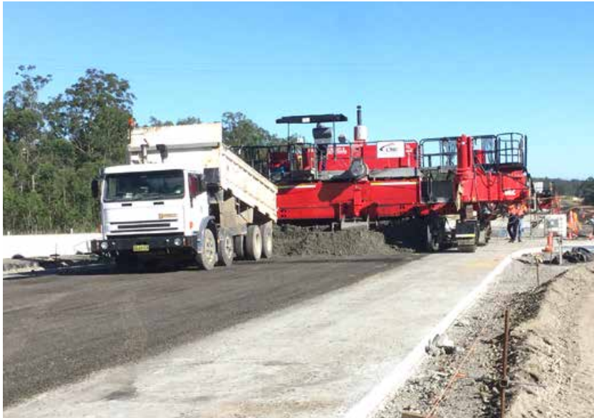
Concrete paving on the southbound carriageway at Lemon Tree Road
