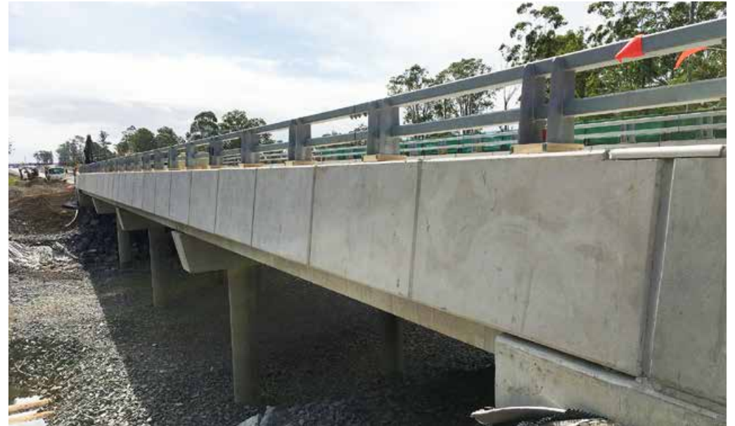
Smith Creek bridge barrier rail installed on the northbound carriageway
