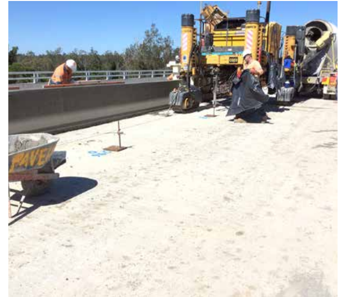
Concrete traffic barrier placed on Wilson River bridge
