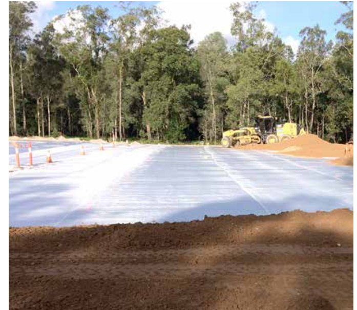
Placement of high strength geosynthetic and fill at Somervale Road
