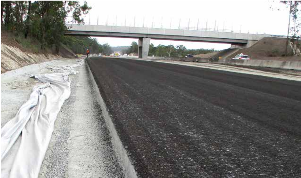
Sealing concrete subbase on northbound carriageway near Kundabung bridge, looking north
