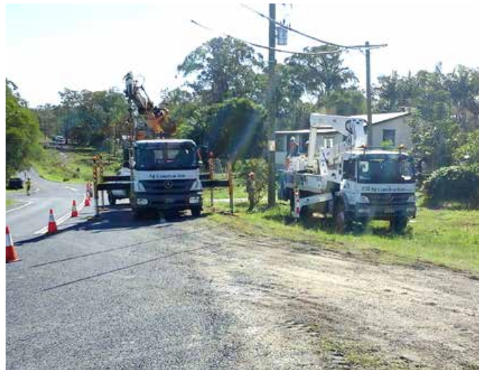
Electrical network relocations at Gap Road, Woodburn
