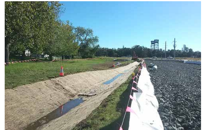
Foundation and open drain at Yamba interchange
