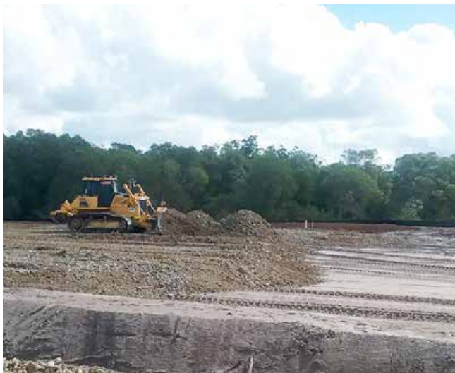
Earthwork to prepare road surface
