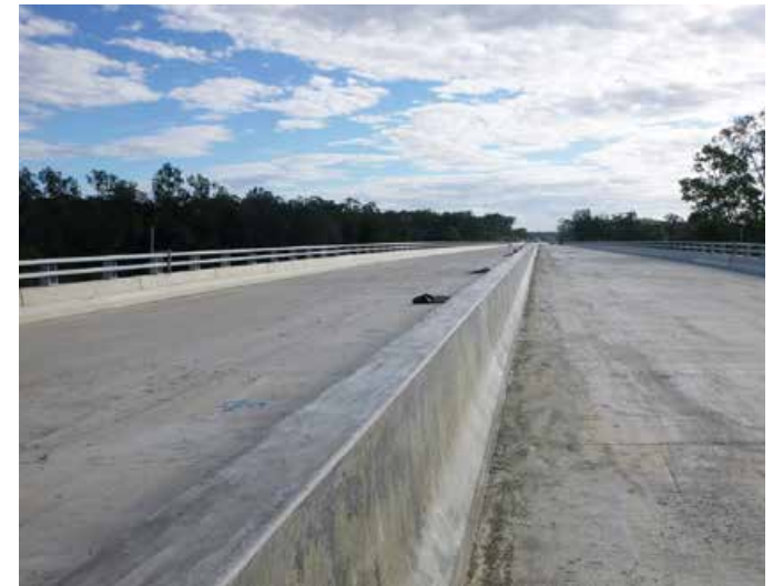
Finished median barrier on the new Wilson River bridge
