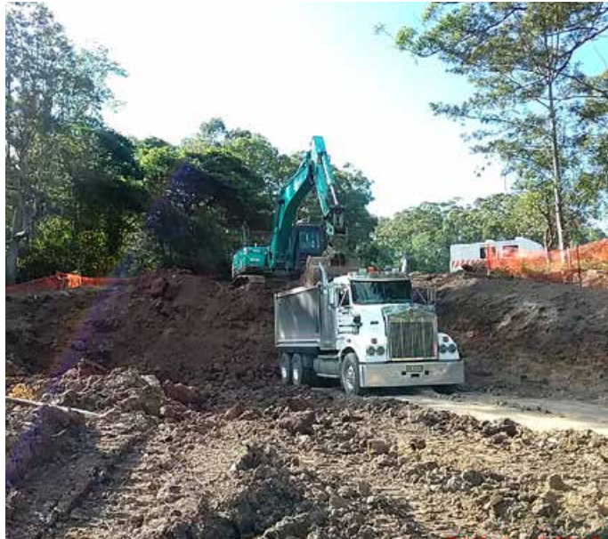
Installation of acid sulphate treatment area near Garretts Lane
