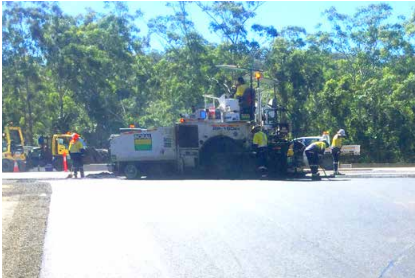
Placing asphalt at Dunmar Lane
