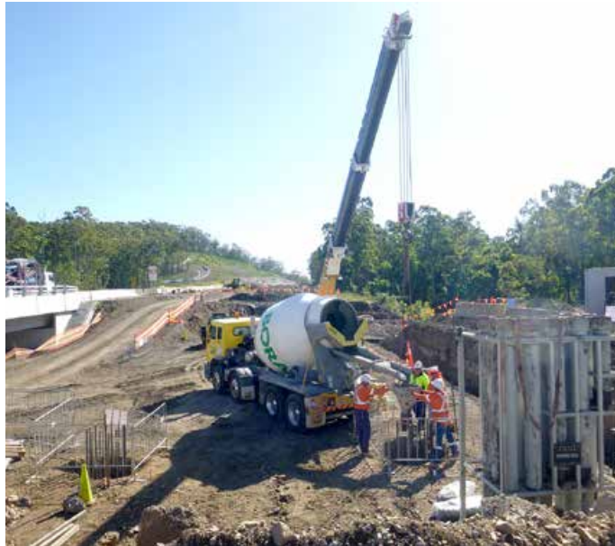
Concrete is placed into a pile hole at Yarrabee Road overbridge
