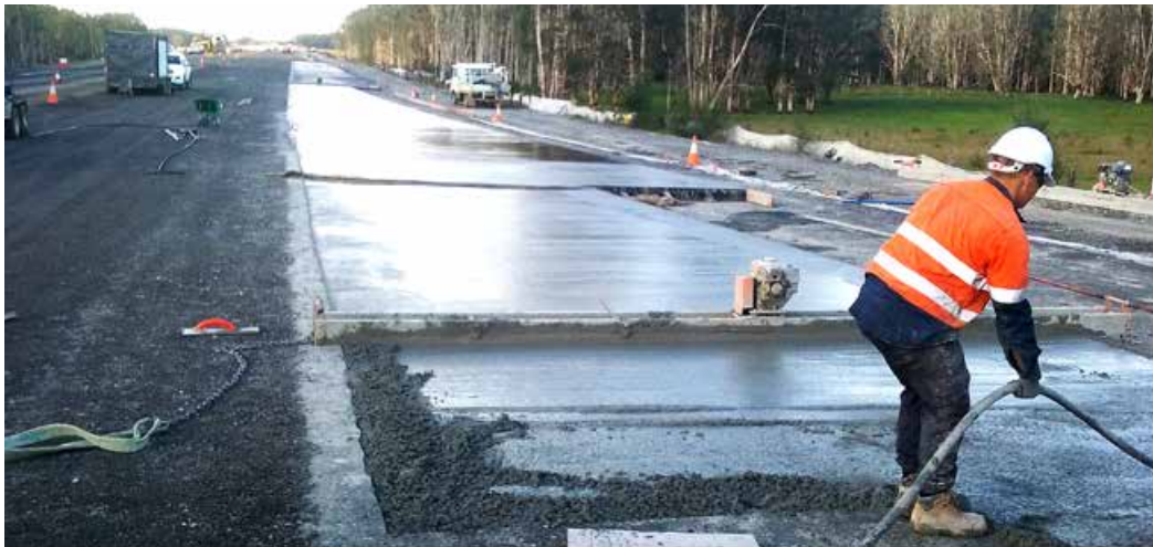
Hand pouring concrete in the north of the project
