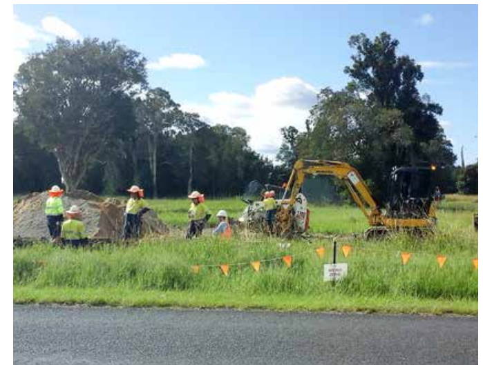
Sewer relocations on Woodburn-Evans Head Road
