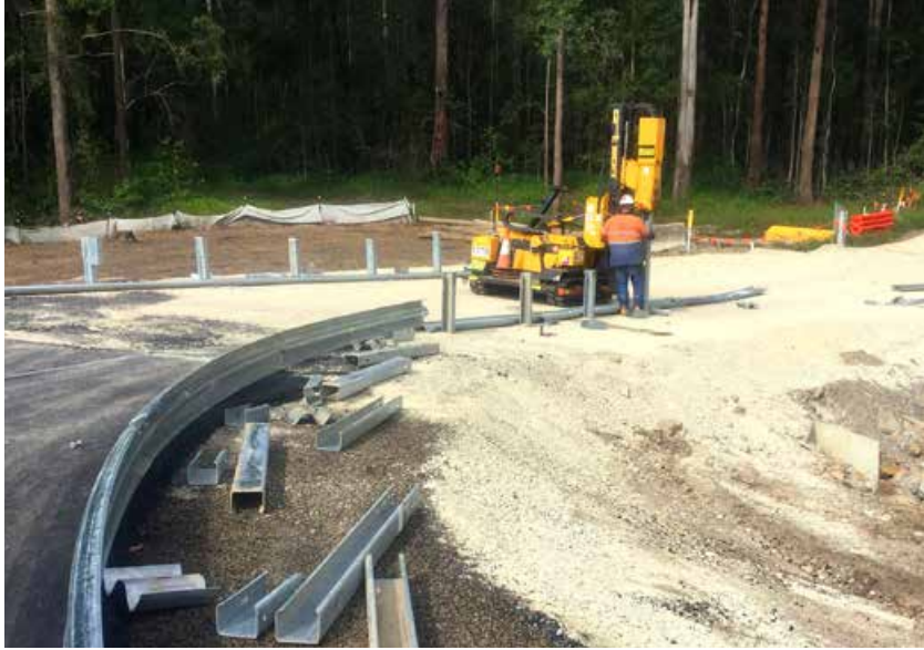
Installing a guardrail at a local access
