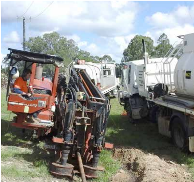
Drilling for Telstra network relocations at Gap Road, Woodburn
