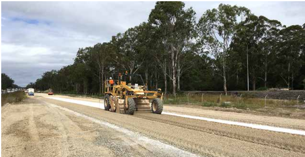
Lime stabilisation of pavement on the northbound carriageway south of Smiths Creek, looking south
