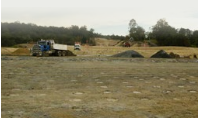
Soft soil treatment work at Kalang River
