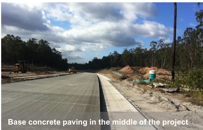
Concrete base paving for road shoulders
