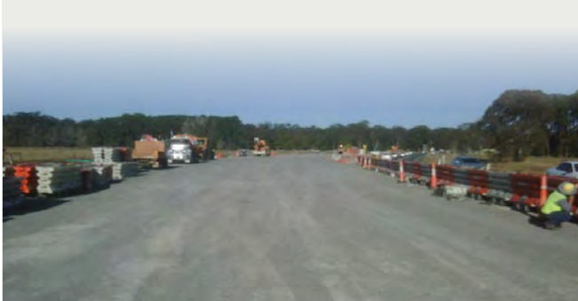
General fill over the bridging layer next to the existing highway at Farlows Flat
