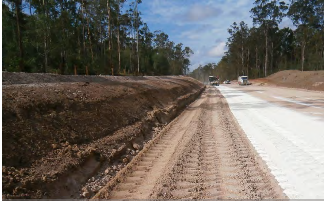
Stabilisation work at the southern end of the project
