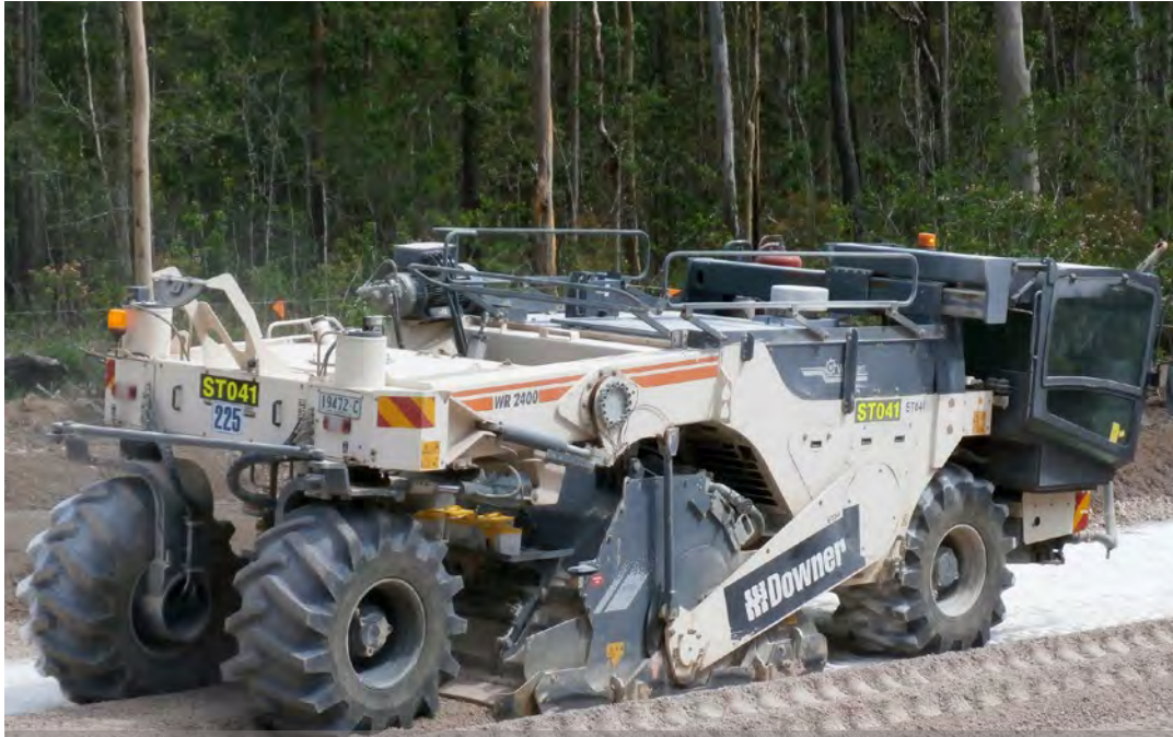
Lime stabiliser carrying out stabilising work
