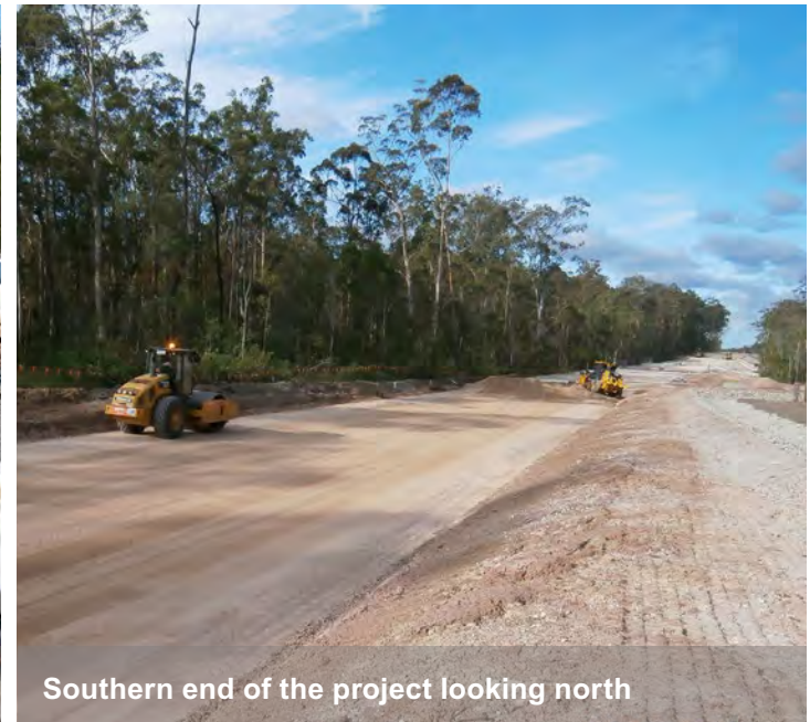
Stabilisation work at the southern end of the project
