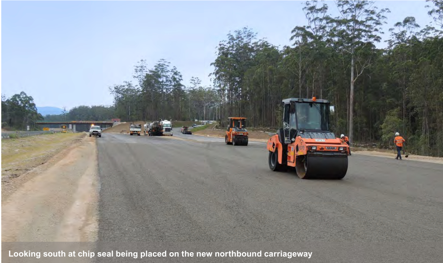
Pavement work under way for base bridging layer
