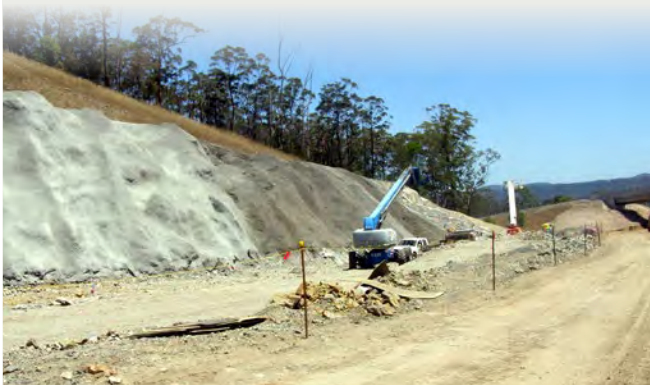
Batter stabilisation work on the eastern side of the main cutting north of Bombah Point Road
