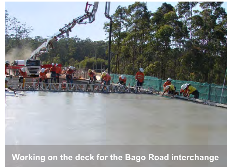
Pavement work under way for base bridging layer
