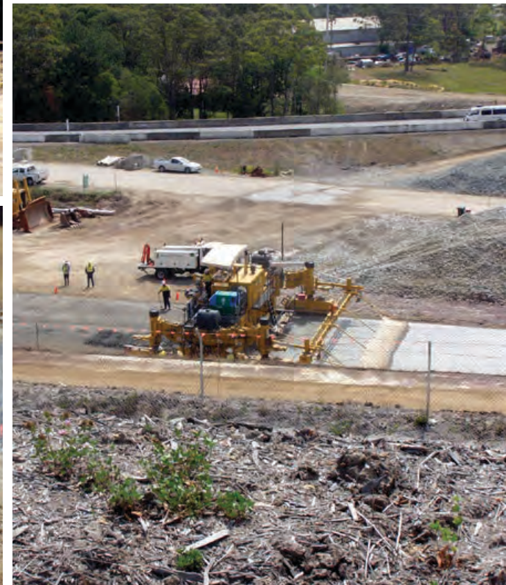
Concrete paving on the main alignment underneath the northern interchange
