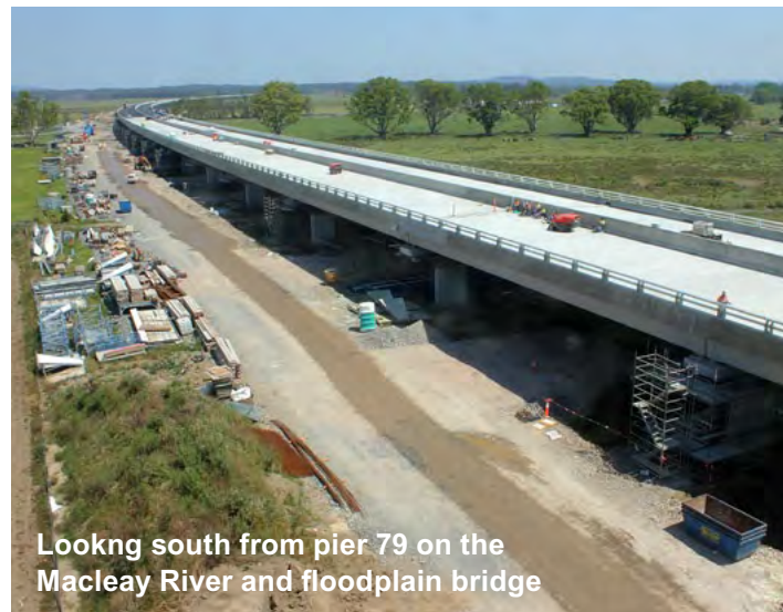
Asphalt surfacing of the bridge deck on the Macleay River and floodplain bridge
