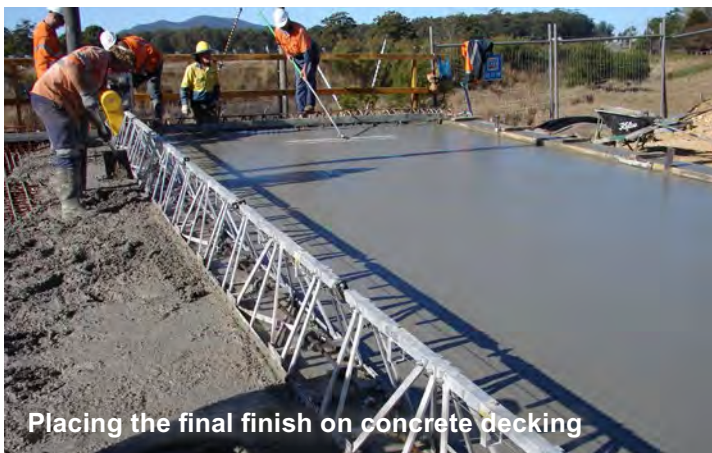
Concrete decking being poured on the Herons Creek floodway bridge
