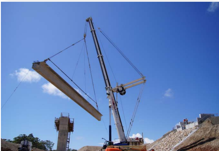
Girders being lifted into position on the Greys Road bridge
