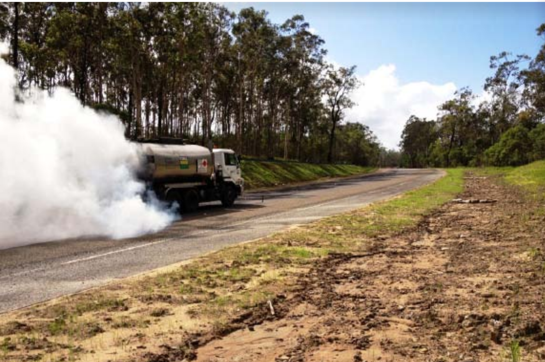
Spray sealing at Rocky Corner
