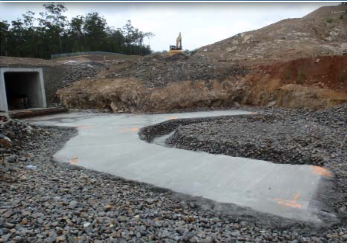
Preparing the last section of the Bingus Lane fauna underpass
