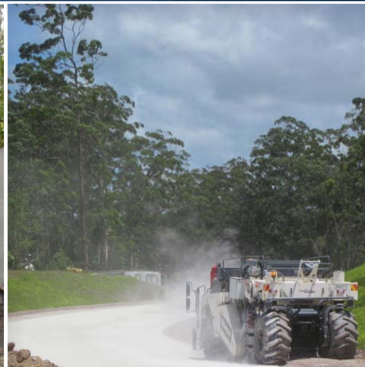
Lime stabilisation work on northbound on ramp
