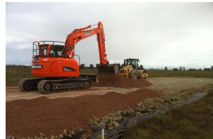
Placing the top layer of rock to complete the crane pad.
