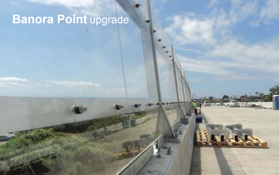
Noise walls on the eastern side of the southern valley viaduct
