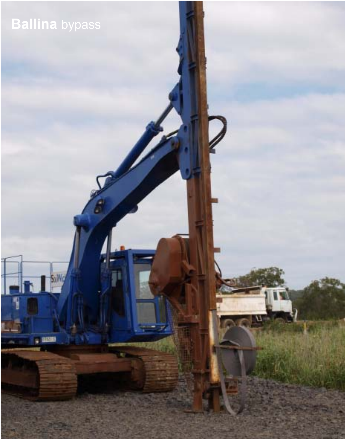
Installation of wick drains for soft soil settlement near the Bruxner Highway
