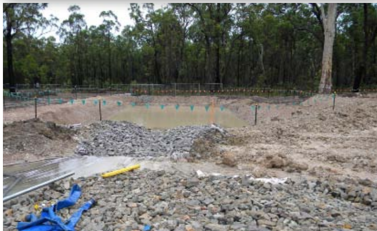
Construction of sedimentation basin
