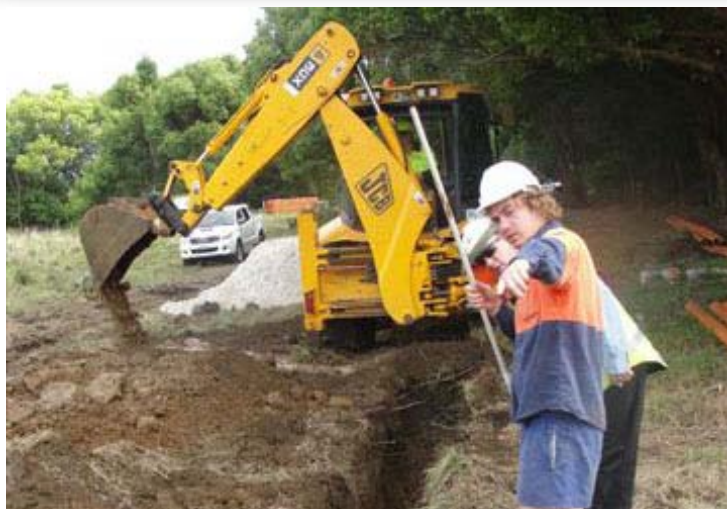
Dedicated electrical feeds for the St Helena tunnel
