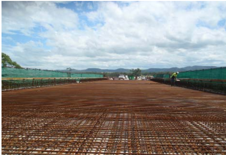
Deck reinforcement on the Myall River bridge
