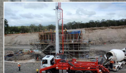
Building centre pier support, South Kempsey interchange
