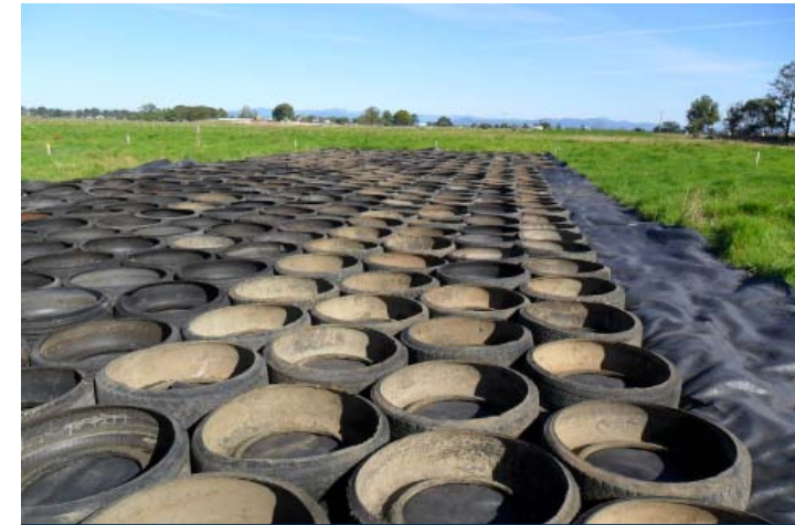
Initial placement of the used tyres to form the crane pad.
