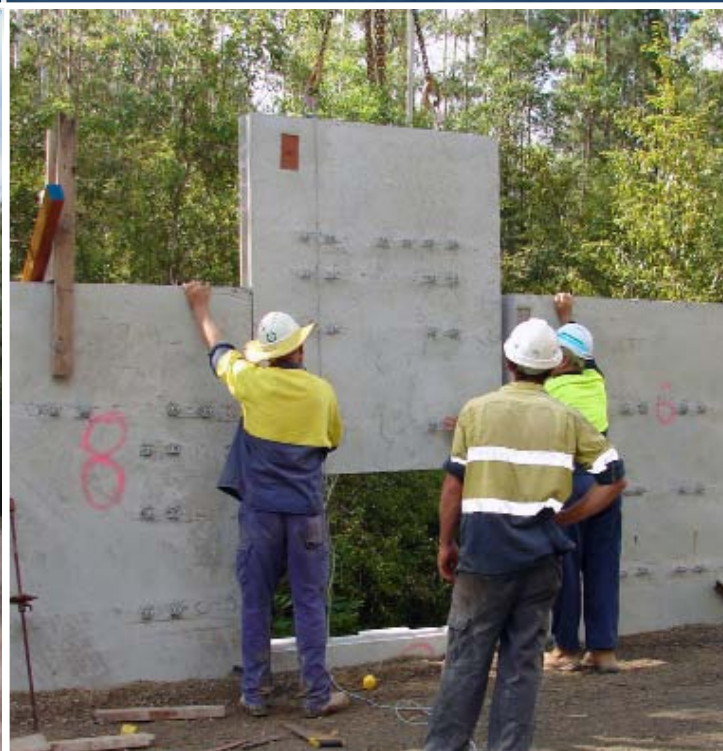
Placing final panels on reinforced earth wall
