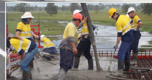
Placing concrete for first deck pour at the Macleay River and floodplain bridge
