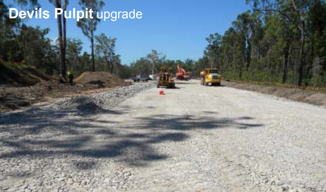
Construction of rock bridging
