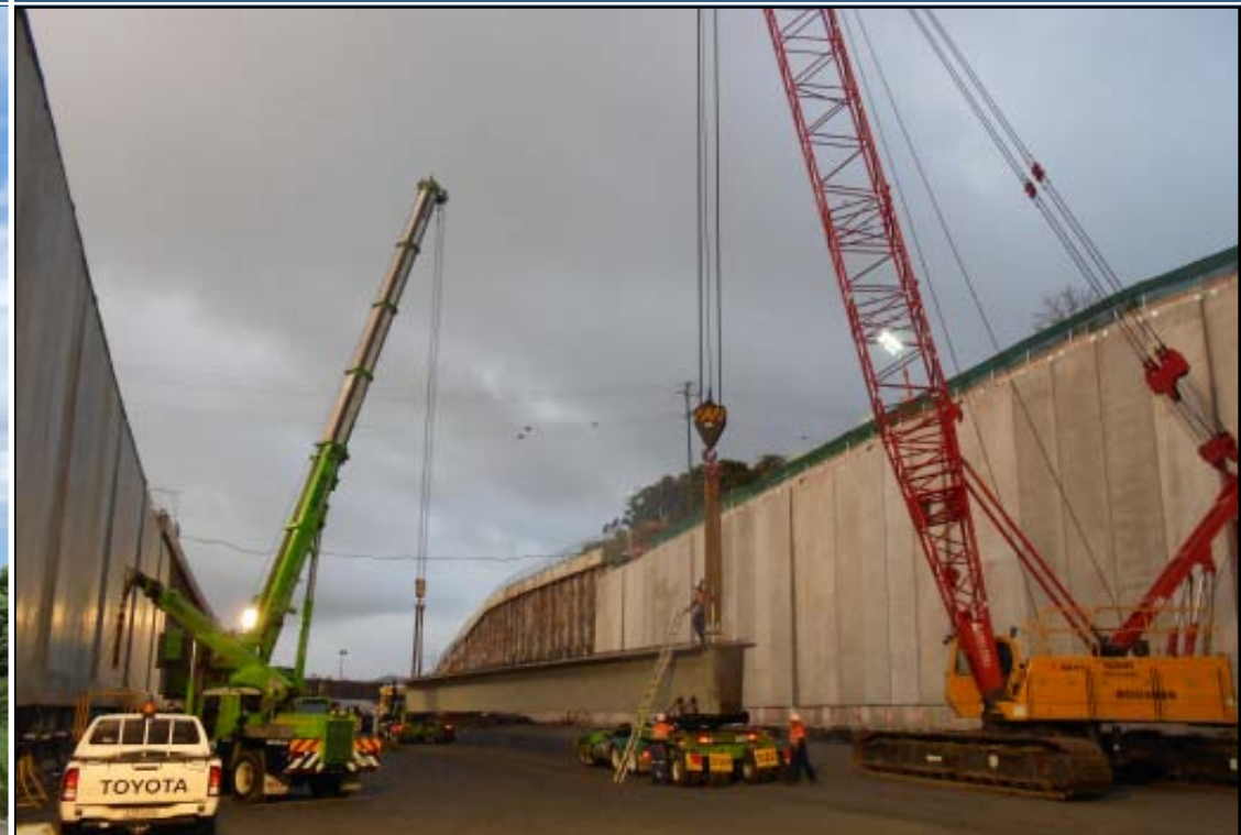
Preparation for girder placement on the landbridge
