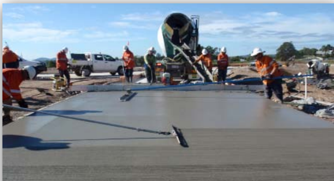
Placing base concrete at Frederickton interchange roundabout
