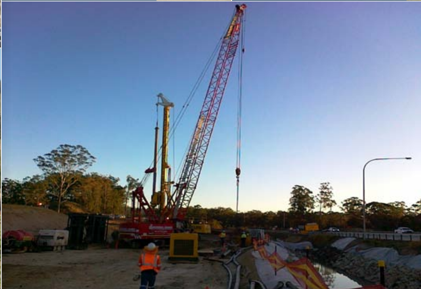
Piling operations for the Moonee Beach interchange
