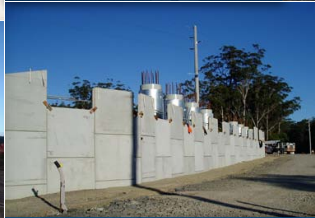
Construction of reinforced Soil Wall at North Coast Railway
