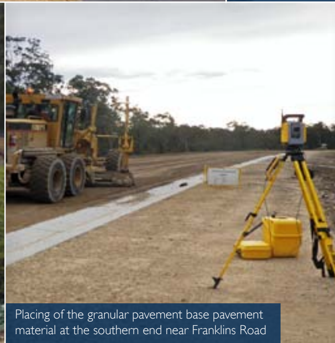
Importing of granu base pavement material
