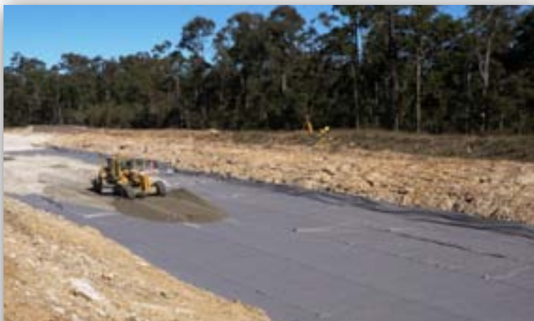
Installation of Geofabric material and the placement of select material over the drainage blanket rock north of Glenugie Creek
