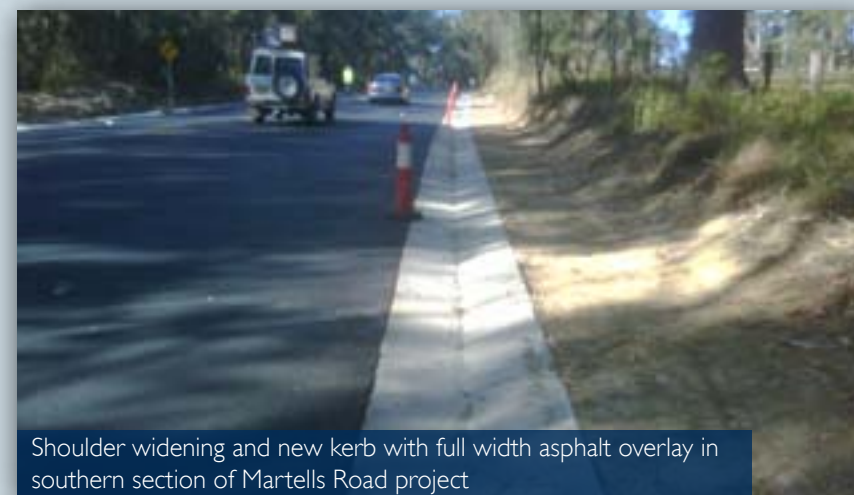
New widened pavement at Martells Road junction prior to asphalt overlay across full width
