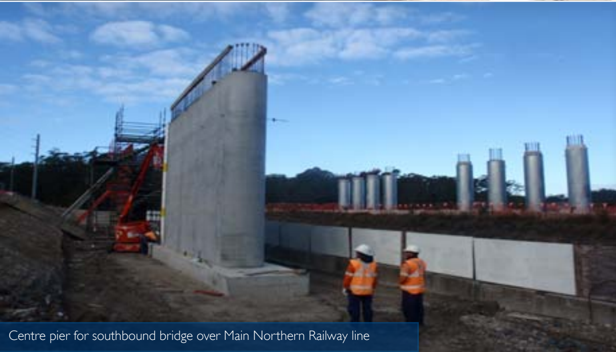
Concrete pour for centre pier at the North Coast Rail Overbridge
