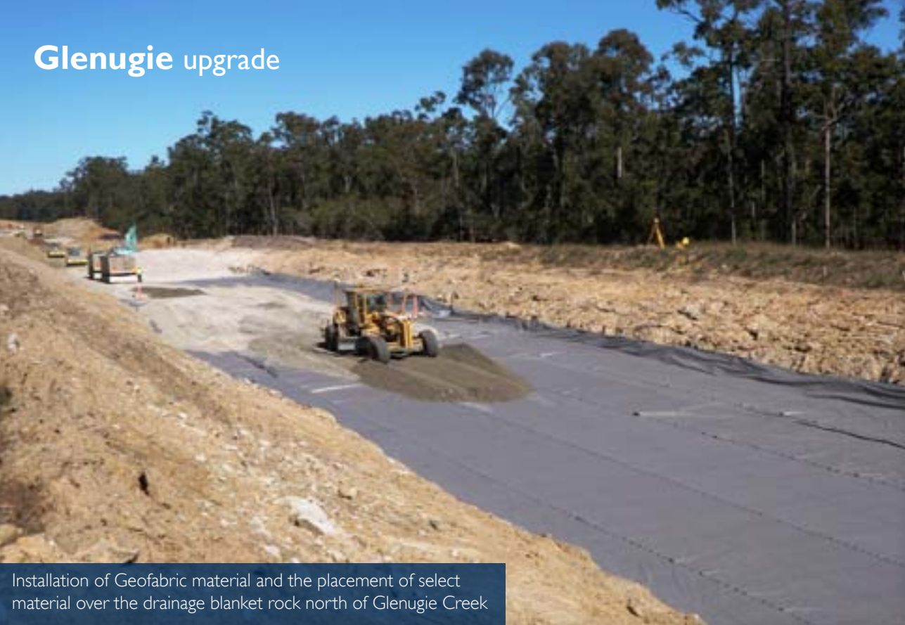
Importing of granu base pavement material
