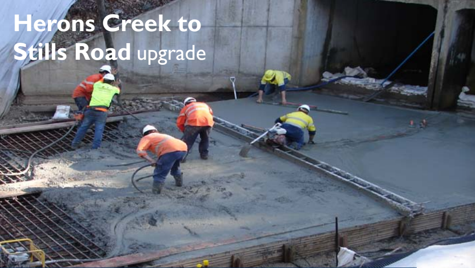
First concrete pour for Cutty Creek culvert base slab
