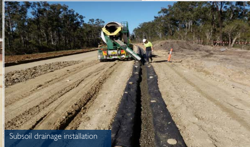
Drainage blanket rock being installed
