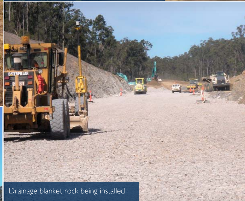
Placement of pavement material with the grade controlled by remote
