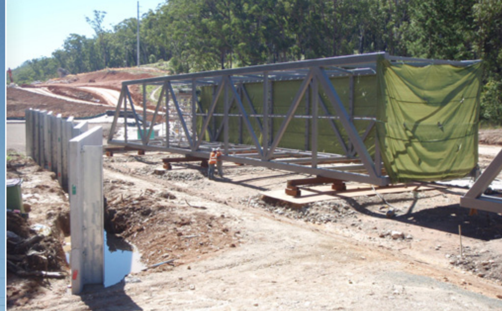
The noise wall and steel truss bridge being assembled at the Mountain Park area
