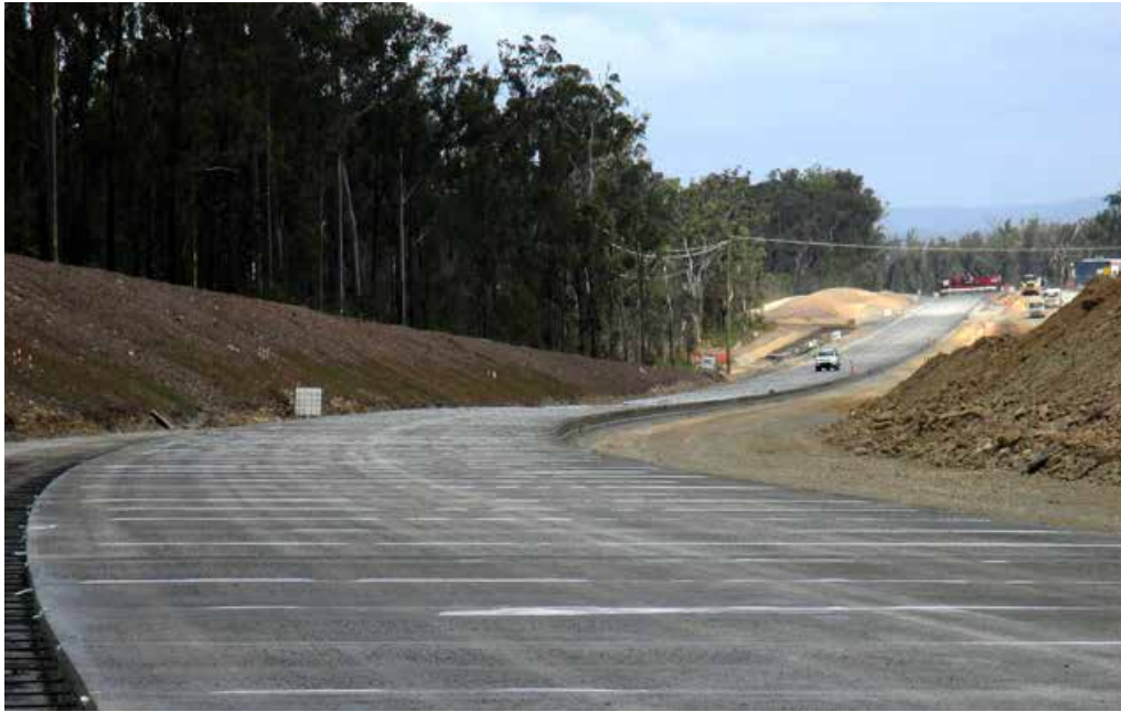
Concrete paving south of Bald Knob Road
