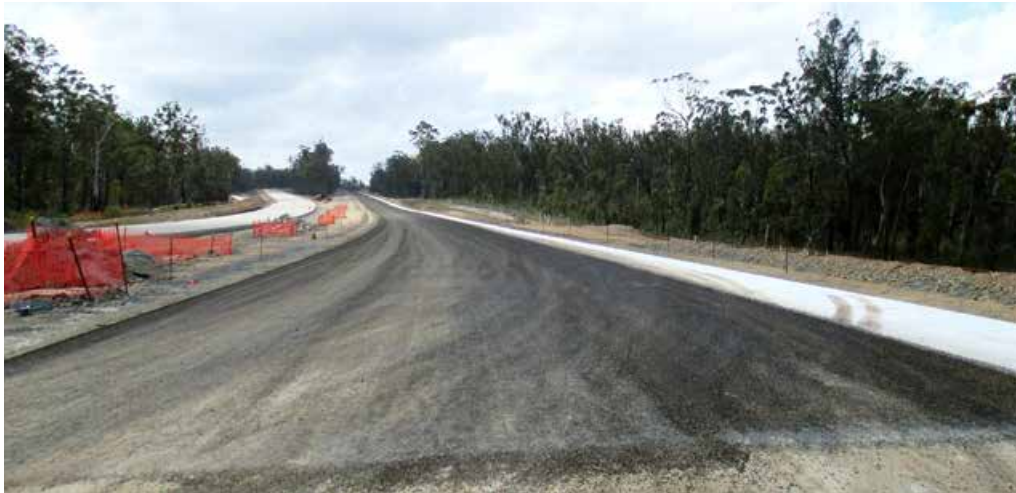
Concrete paving north of Wells Crossing
