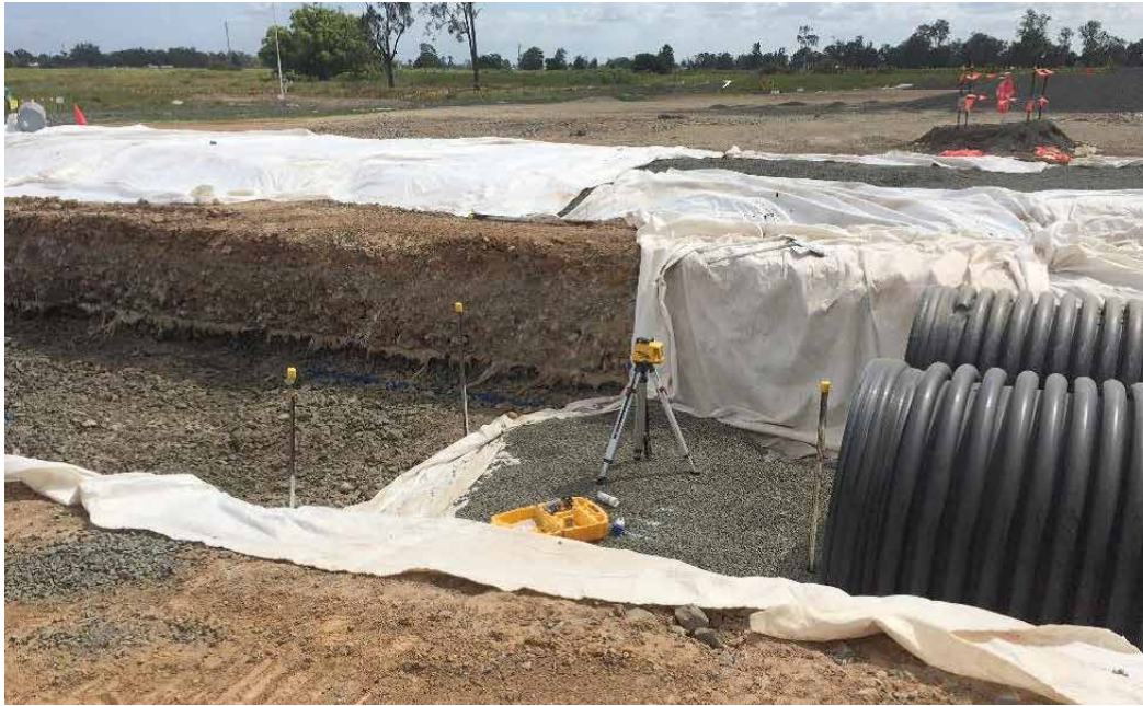
Building temporary drainage on the southern embankment
