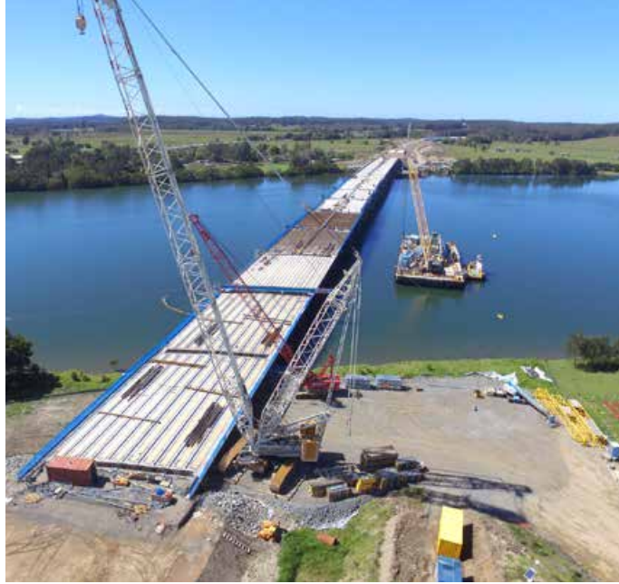
All girders are now in place on the new Wilson River bridge
