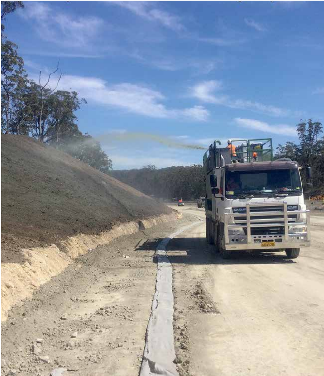
Hydroseeding the batters as part of the landscaping work
