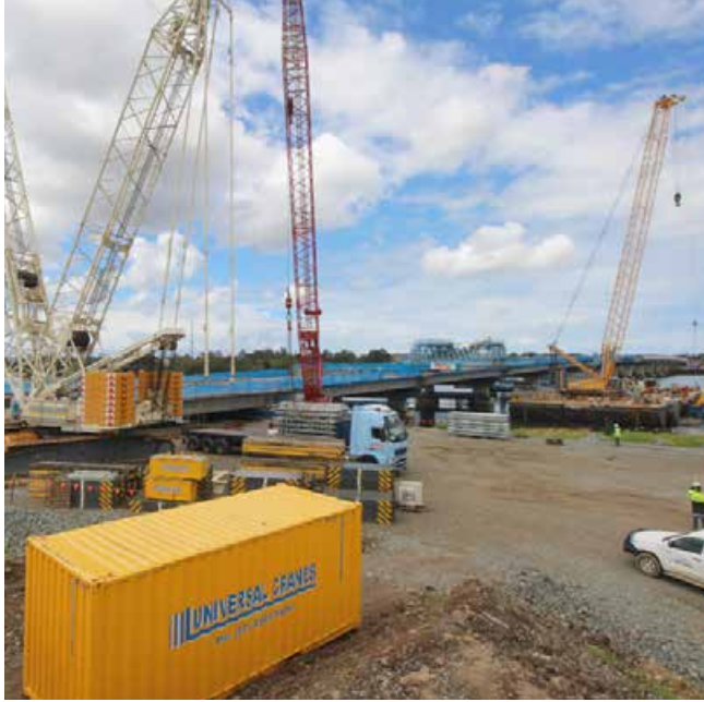
The final girder lifted into place on the new Hastings River bridge
