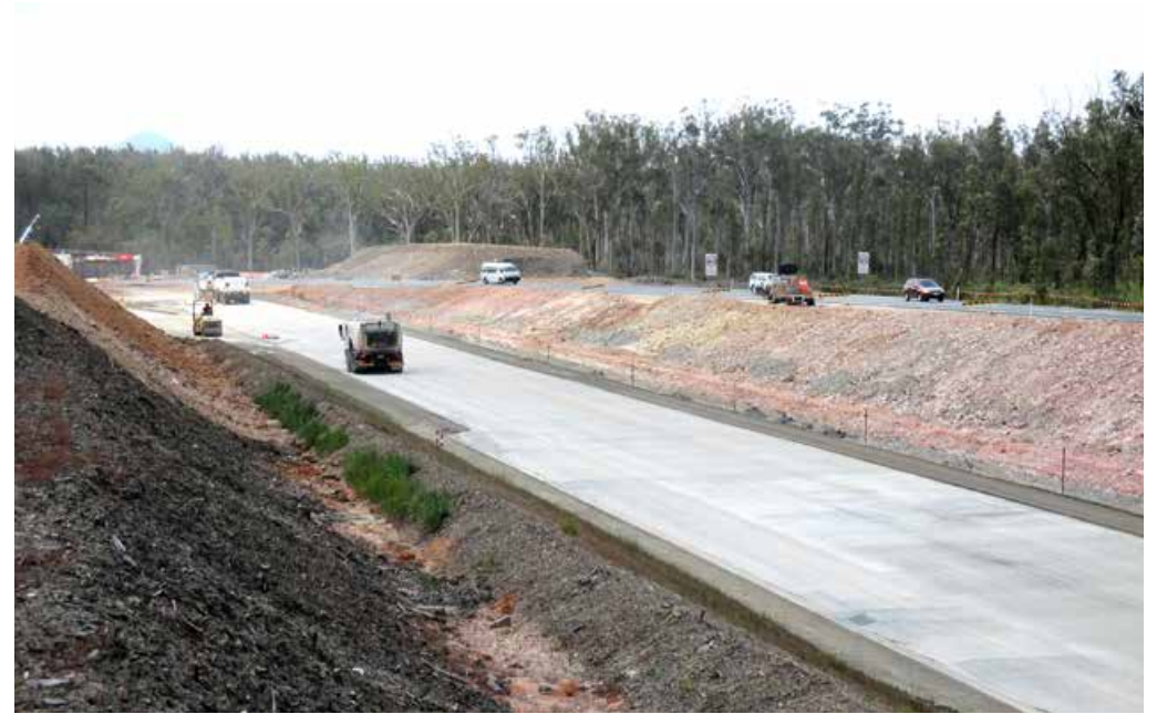
Finishing work on the new northbound carriageway south of Wells Crossing
