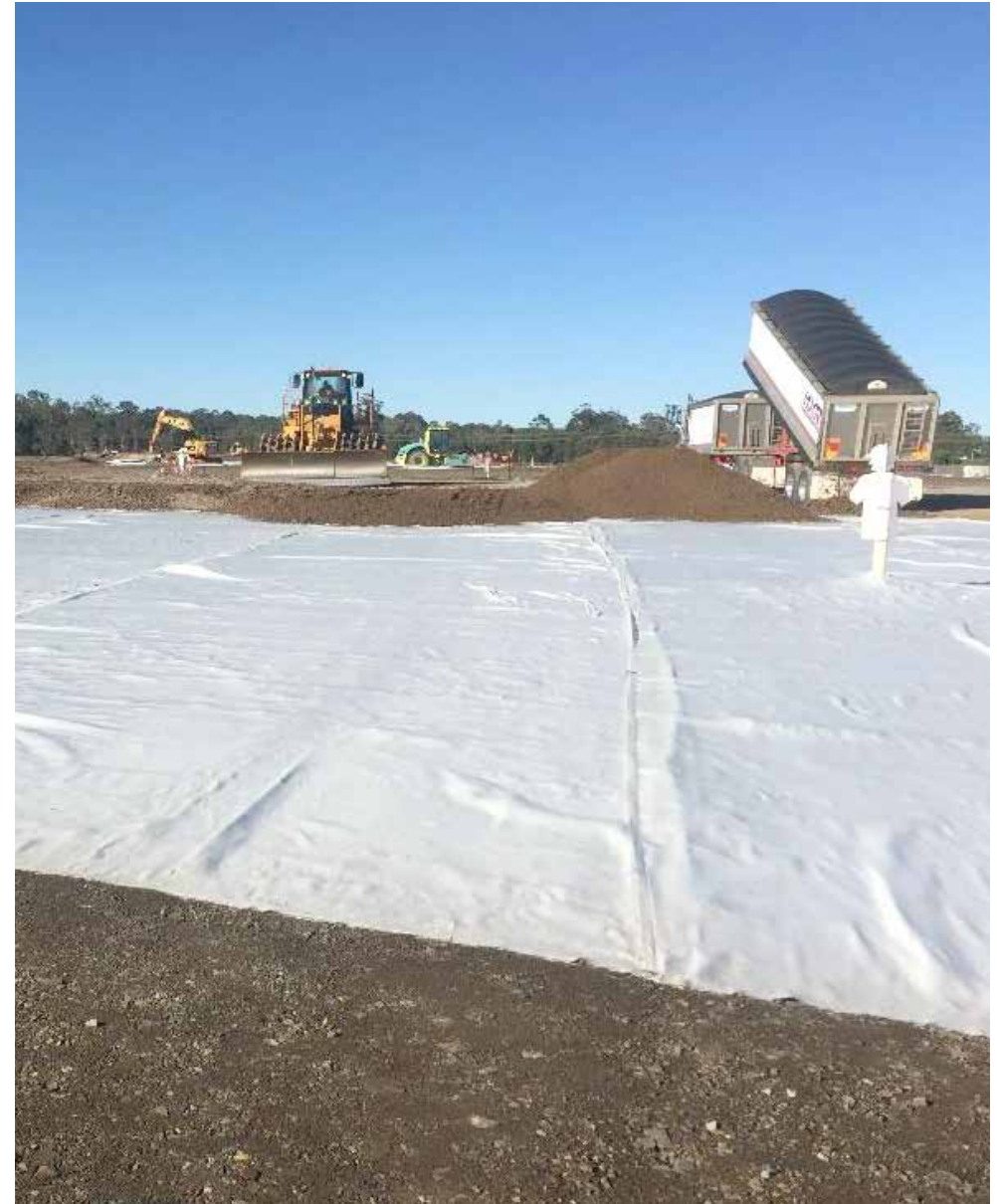
Placement of material over the high strength geosynthetic sheet on the southern embankment
