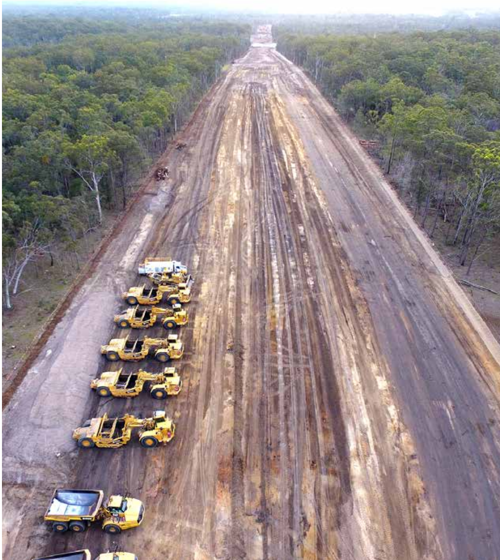
The scraper fleet ready to start following clearing works
