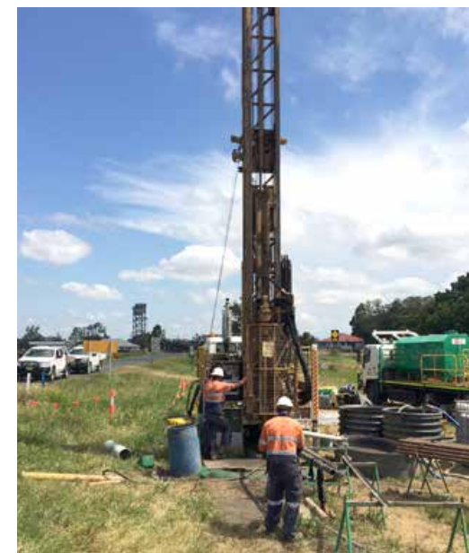
Geotechnical investigations in progress
