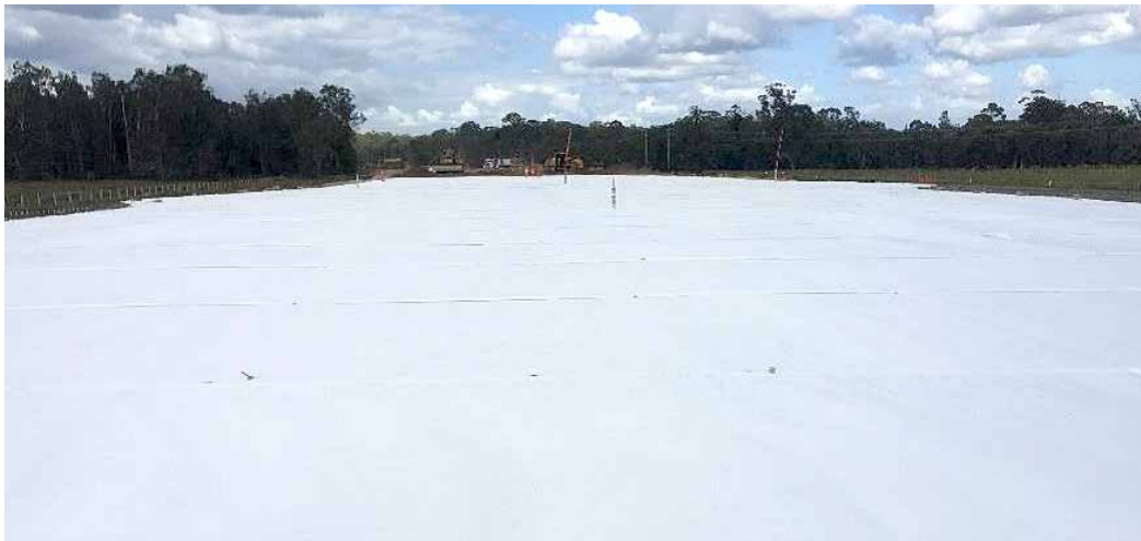
High strength geo-synthetic placement on the southern section
