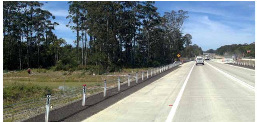
Wire roping and linemarking on new southbound traffic switch
