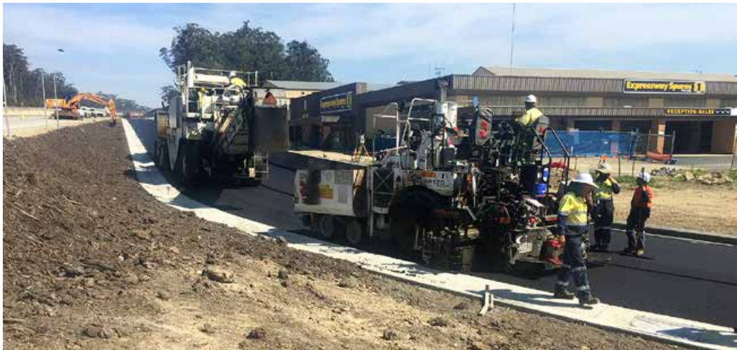
Asphalt placed on the off ramp at the new Sancrox Road intersection
