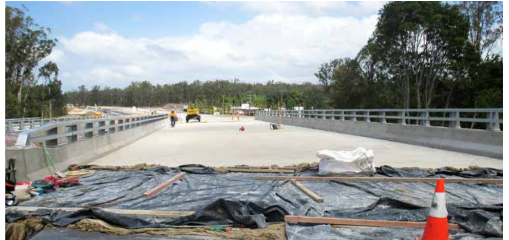
Northbound Halfway Creek bridge railing completed
