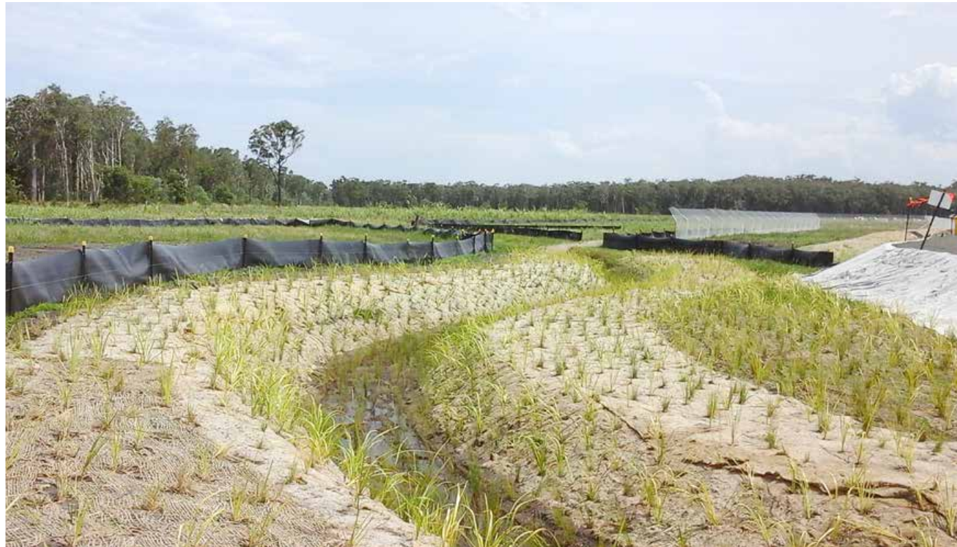
More than 8000 creek grass plants were used to stabilise the sites before the Oxleyan Pygmy Perch spawning season
