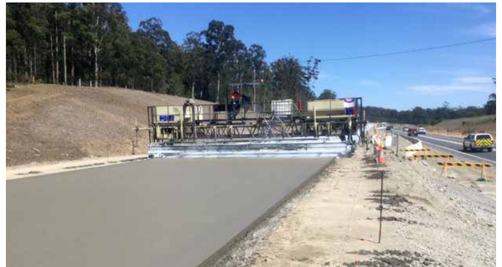
Wax compound application on concrete
