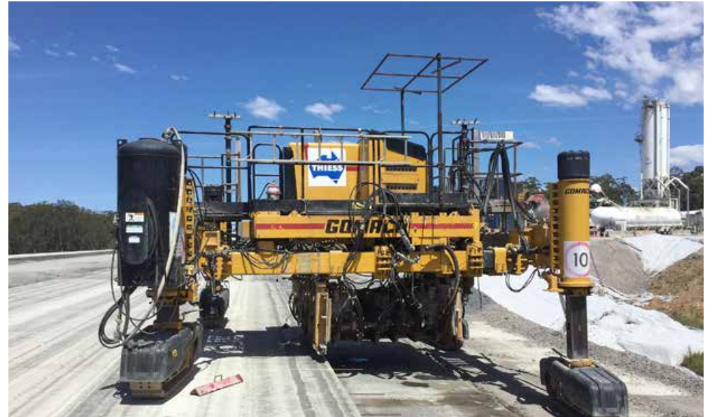
Shoulder pavement placement
