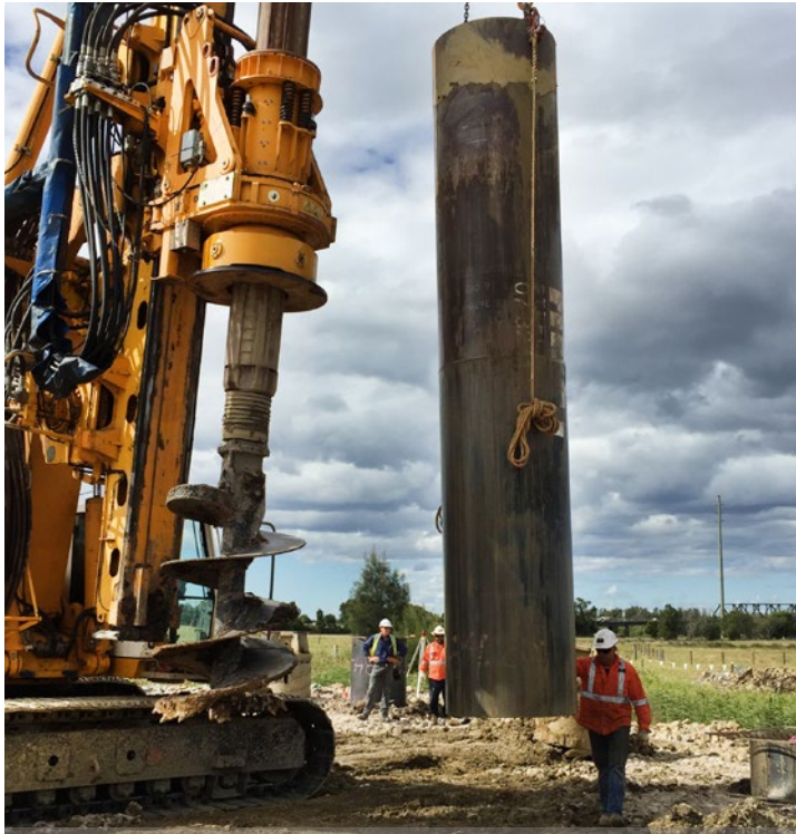
A temporary steel casing about to be driven into the ground during piling at the floodplain bridge just north of the Hastings River
