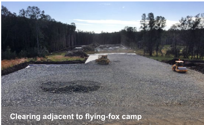
Looking south at earthworks and the building of a sedimentation basin west of the Boral quarry
