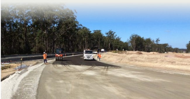
Spray sealing of the temporary traffic diversion near Blackmans Point turnoff
