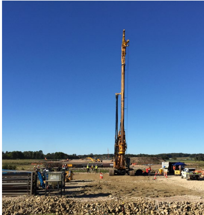
Bridge piling started at the floodplain bridge just north of the Hastings River
