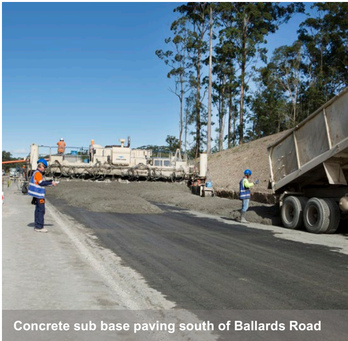
Building the lower layers of road surface looking south to the Ballards Road overbridge
