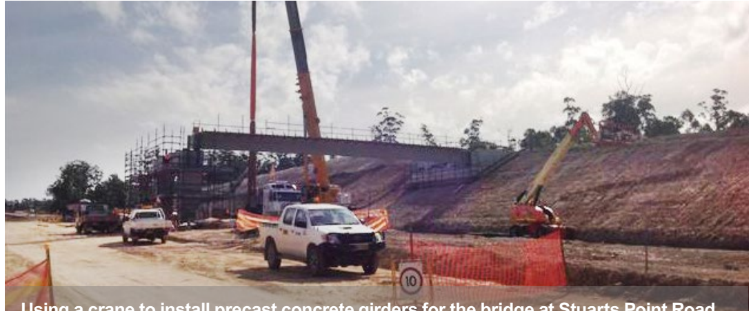
Using a crane to install precast concrete girders for the bridge at Stuarts Point Road interchange, looking north
