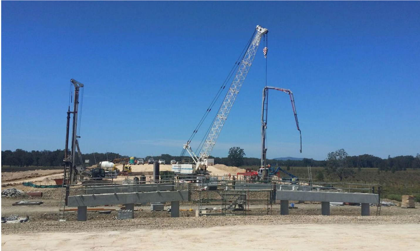
Pouring concrete for bored piles on the bridge over Johnsons Creek, looking north
