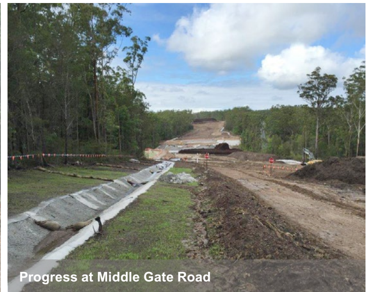
Stripping of topsoil in the Maria State Forest, looking south at Middle Gate Road
