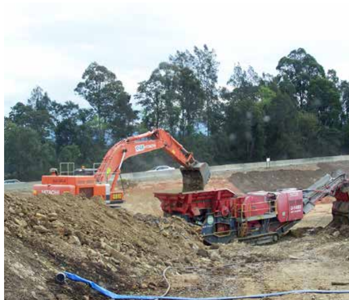
Crushing work being carried out at the cut north of Lower Warrell Creek
