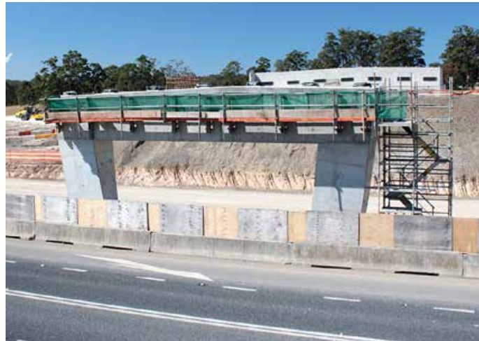
The centre pier erected for the Kundabung Road overbridge
