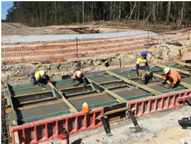
The first concrete pour for a culvert base slab was carried out in August
