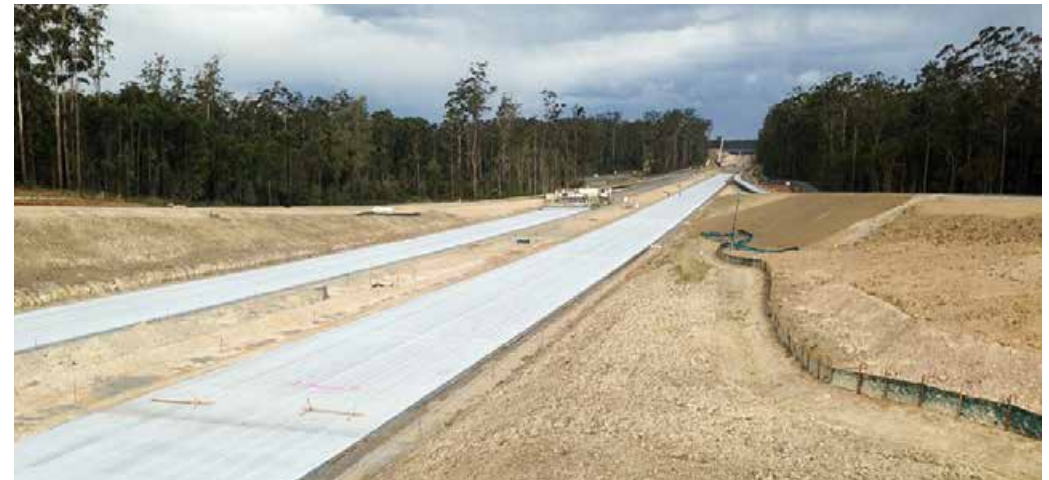
Sub-base pavement near the Borigalla Creek twin bridges
