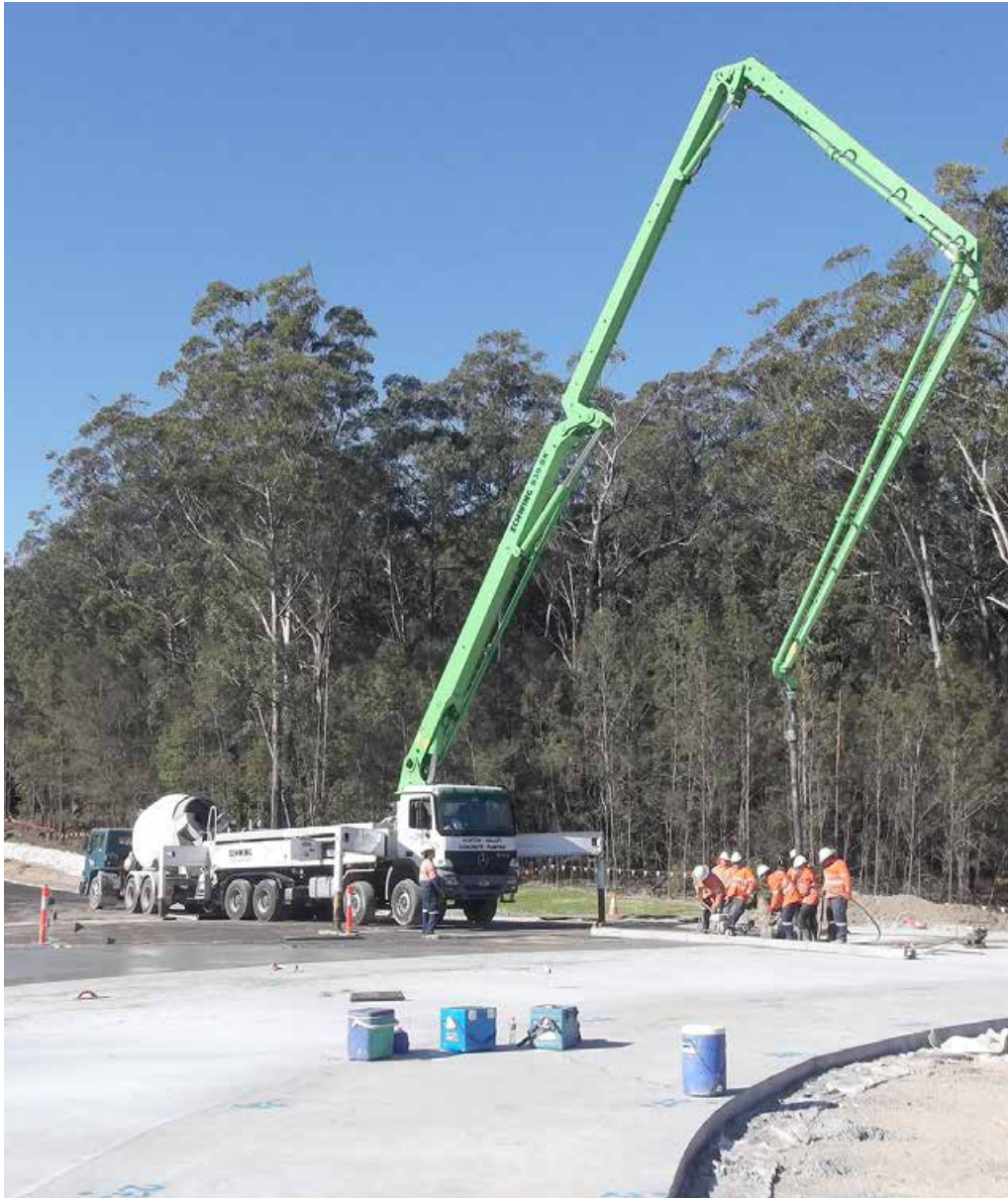
Pouring the lower layer concrete paving at the Fernbank Creek Road roundabout
