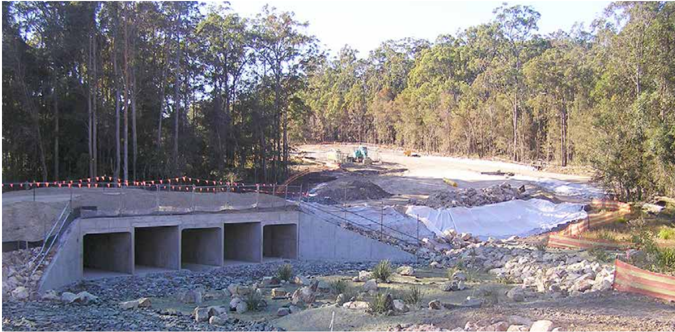
New box culvert under realigned Mingaletta Road
