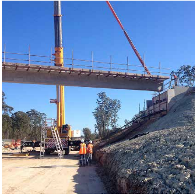
Erecting a girder at Barraganyatti Road overpass bridge
