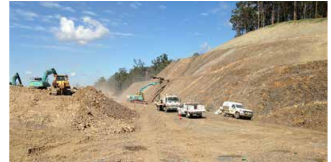
Working on the Cooperabung cutting, where controlled blasting has removed the rock and formed benches that improve the long term stability of the rock face
