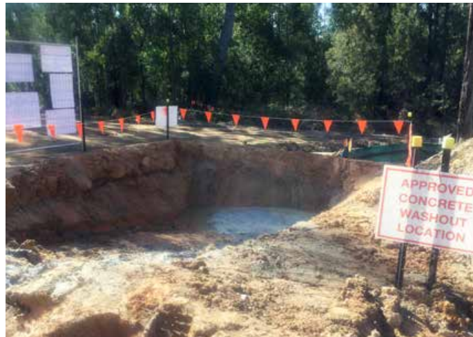
A concrete washout area
