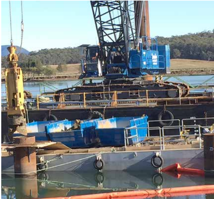
Steel tubular piles are driven through the alluvial river bed and into rock. Reinforced concrete is later placed inside the steel tube
