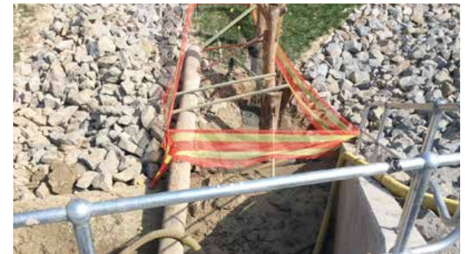
Animal refuge poles are being placed near box culverts, which allow wildlife to cross under the new highway
