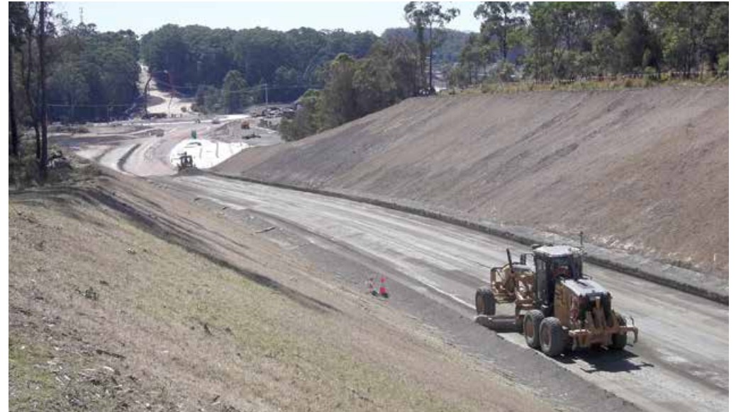
Finishing the top layer of earthwork in preparation for the start of pavement construction
