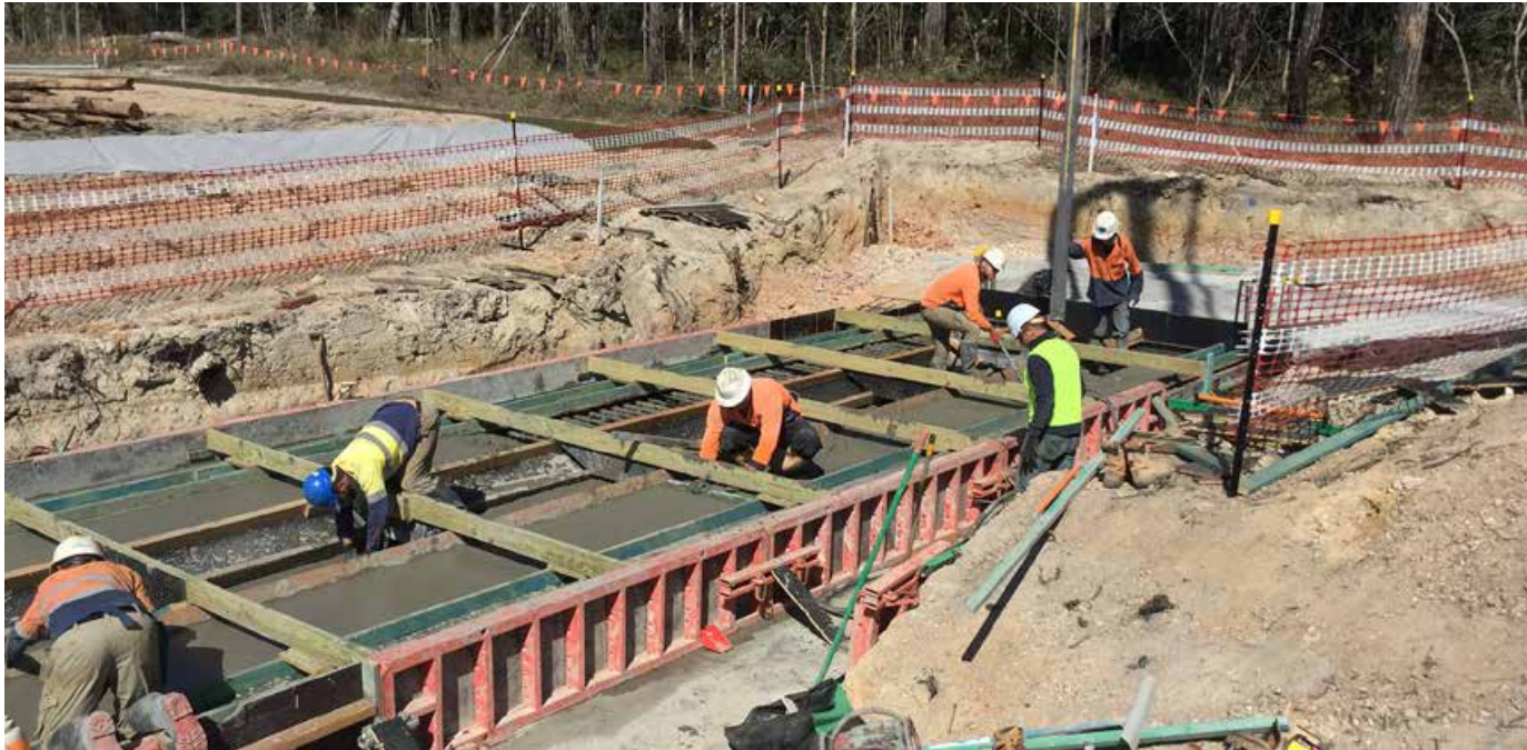
Pouring concrete for a culvert
