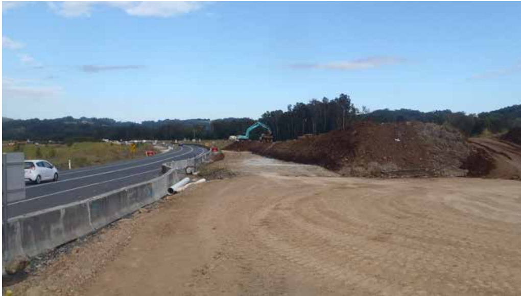
Removing surcharge south of Duck Creek
