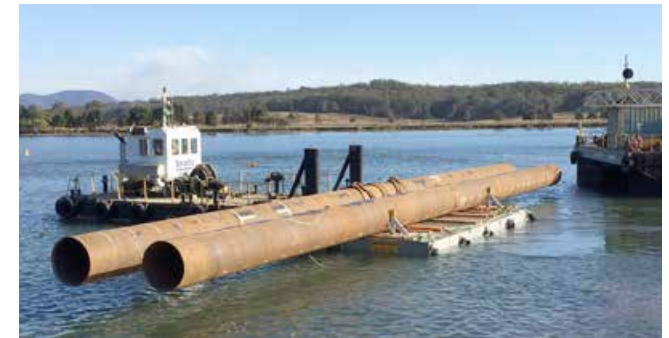
Steel tubular piles being delivered by barge to the larger main piling barge on the Hastings River
