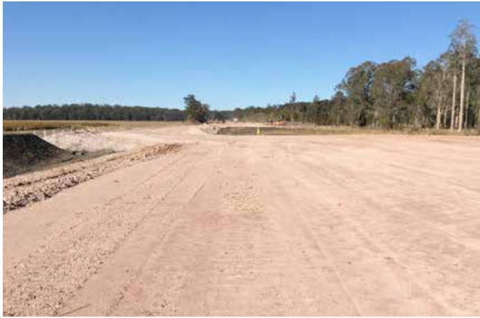
Earthwork foundations are now continuous across the Wilson River floodplain. Earthwork started from each end of the floodplain, and met in the middle, during August
