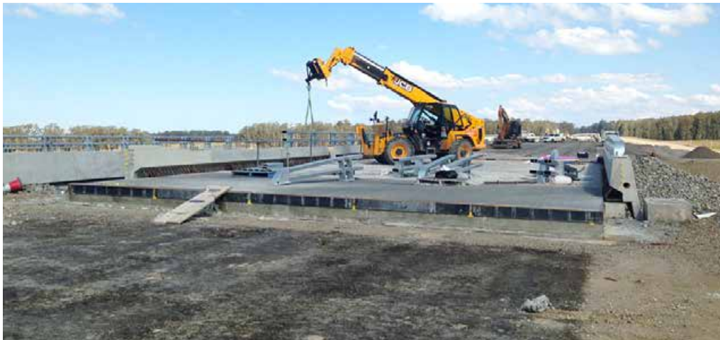
Installing bridge railings on bridge over Seven Oaks drain, looking south
