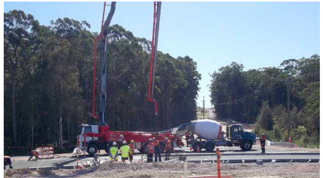
Pouring the lower layer of concrete paving for the Sancrox Road roundabout
