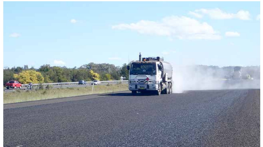
Spraying bitumen seal on the new Bruxner Highway alignment
