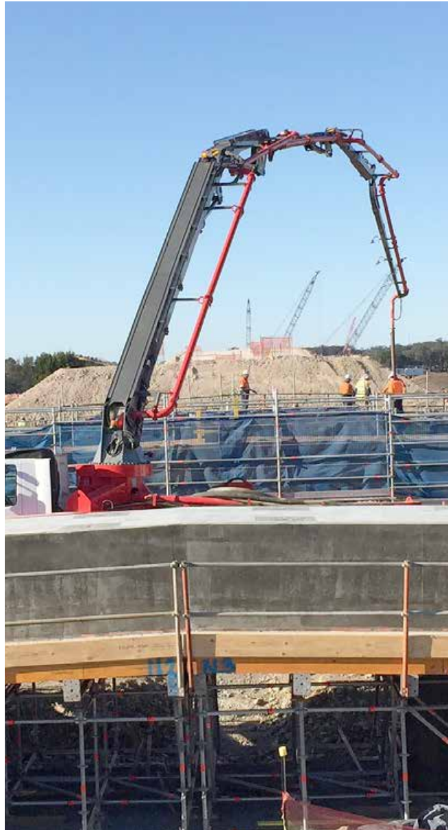
Concrete is pumped into place on the floodplain bridge being built just north of the Hastings River
