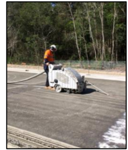
Concrete saw cutting
