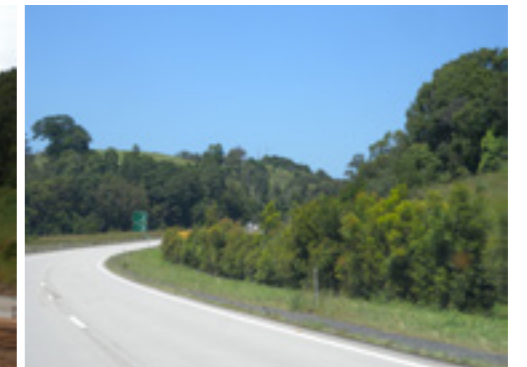
Figure 18: Ballina Bypass January 2015.
