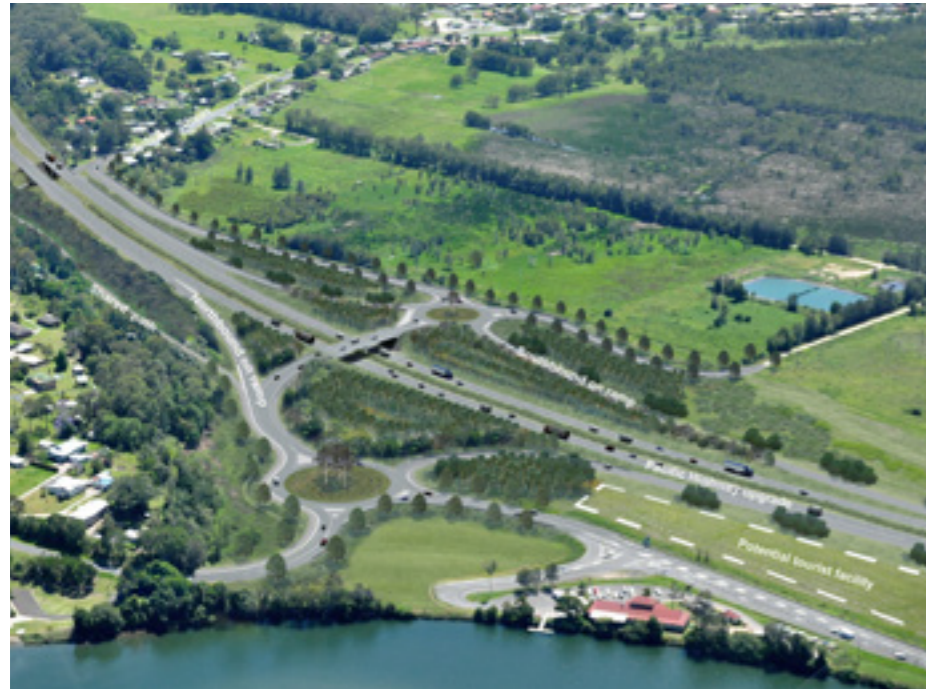
Figure 7: Maclean interchange – aerial view looking north. Subject to further community consultation and design development.
