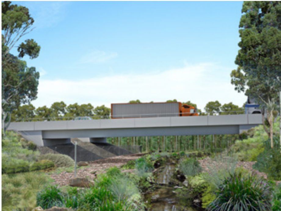
Figure 4: Twin bridges over combined fauna and drainage crossing. Subject to further community consultation and design development.
