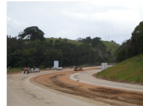
Figure 17: Ballina Bypass February 2011.
