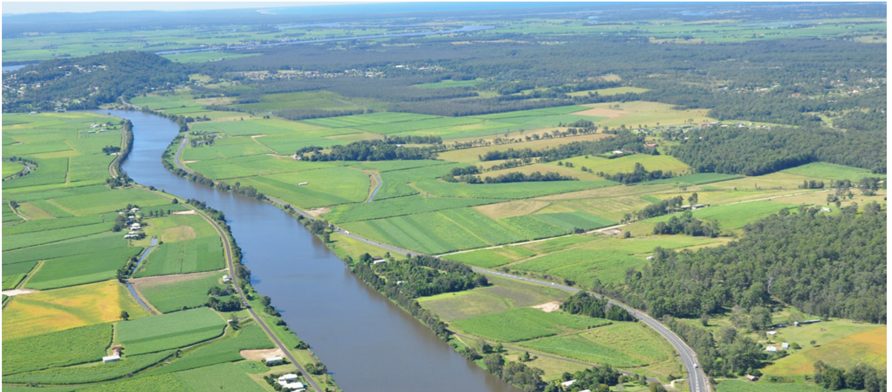
Figure 112: Oblique aerial looking north of Tyndale interchange with Green Hill in foreground and Maclean interchange in background. Source: Pacific Complete
