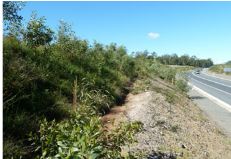
Figure 99: Glenugie batter slope soon after completion showing germination from the soil seedbank.
