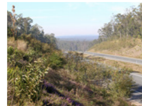
Figure 26: Glenugie upgrade August 2013
