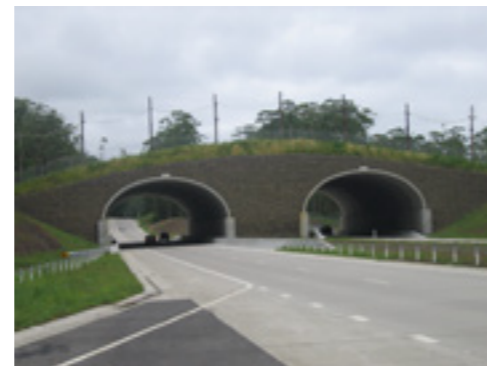
Figure 20: Bonville Koala Bridge February 2009.
