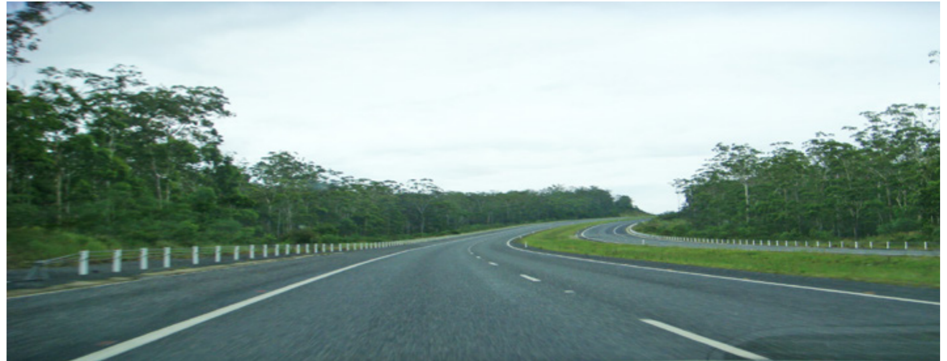
Figure 64: Pacific Highway looking north at Glenugie.
