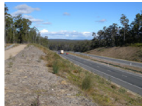
Figure 25: Glenugie upgrade July 2012.
