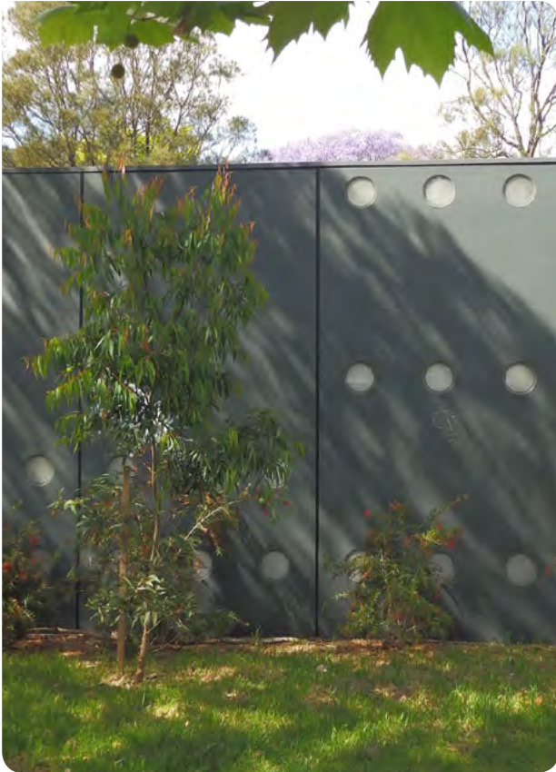
The walls on Syd Einfeld Drive are architecturally designed to protect the park and streets on the residential side and provide a human scale. They have a dark grey recessive colouration. There is great attention given to proportion and articulation of panels and to detail, such as the acrylic portholes.
