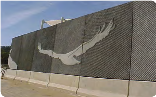
This noise wall on the West Charlestown Bypass has a sea eagle motif that is of significance to the local Aboriginal community and is part of a broader bird life theme. The eagle is set across concrete panels whose diagonal mouldings are a stylisation of the underground coal seams in the area. This forms a strong architectural composition.
