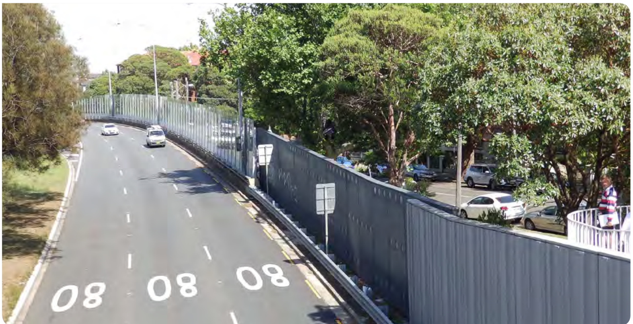
Syd Einfeld Drive: A composition of noise wall types designed to address different conditions on the road and residential side but unified and context sensitive.
