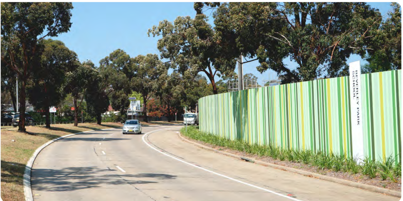
A system of interlocked concrete noise walls protects two Campbelltown schools at Thomas and Moore Streets and helps define this precinct.
