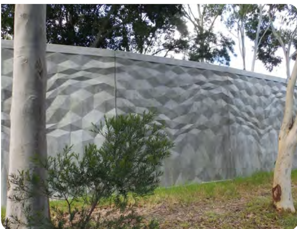
These precast concrete, full height panels at Sexton Place above the Warringah Expressway in Cammeray have a sculptural design on the front face that is both decorative and helps deter graffiti.
