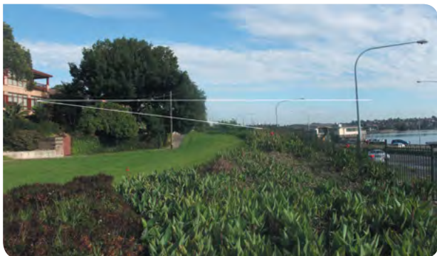
This carefully scaled and well sculpted and landscaped noise mound adjacent to the City West Link in Sydney not only blocks noise from traffic but allows views of the harbour.
