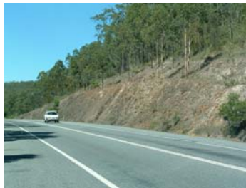
Existing highway cutting in Cooperabung Hill. The Proposal would duplicate the existing highway requiring widening of the cutting.
